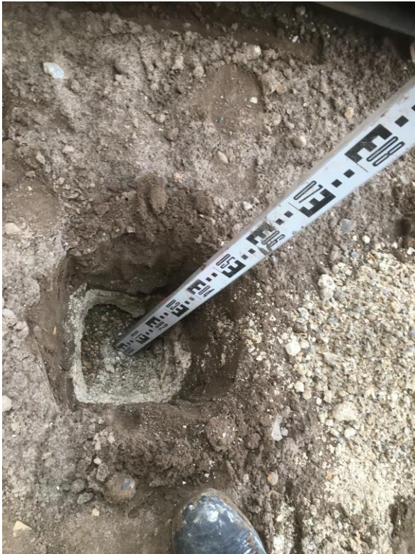
Photographs 8 and 9 , taken on the 10 th December 2019 showing where pea shingle and coarse gravel were encountered within hand dug trial pits (HDT262-03 and HDT266-01) and presumed to indicate the presence of services.
