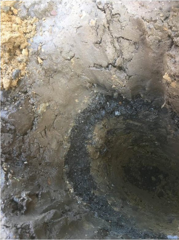
Photographs 5-6 , taken on the 14 th December 2020 showing the black material found, and the attempt to delineate the material within plot 7. The material in question was not present in the three surrounding exploratory locations.
