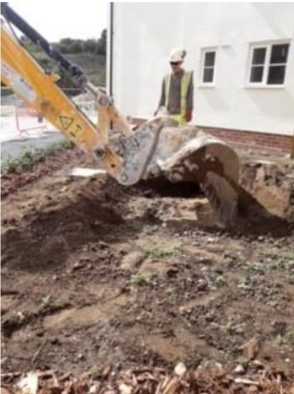
Photographs 6 - 7 , taken on the 6 th September 2019, showing the excavation and removal of the concrete obstruction from the front garden of plot 169 (client supplied).
