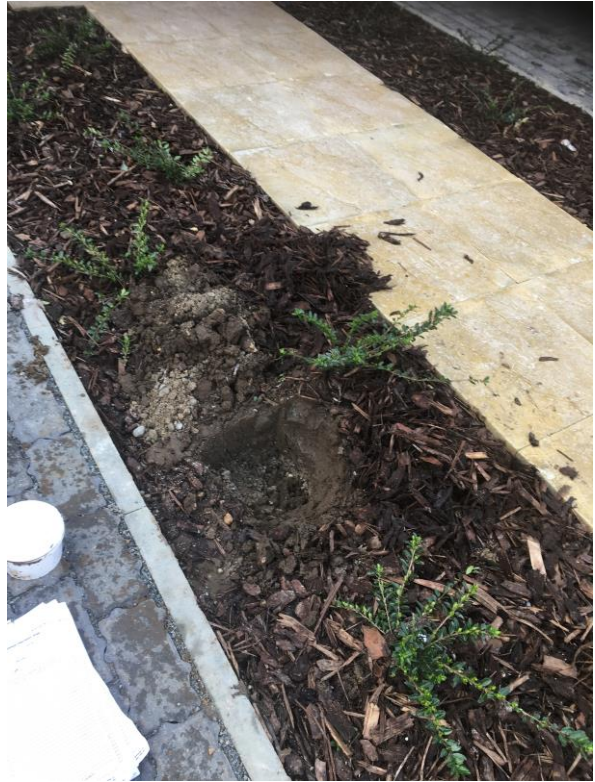
Photographs 5 - 6 , taken on the 4 th February 2020, showing the area of soft landscaping adjacent to the footpath to plot 263 which comprises topsoil over concrete.
