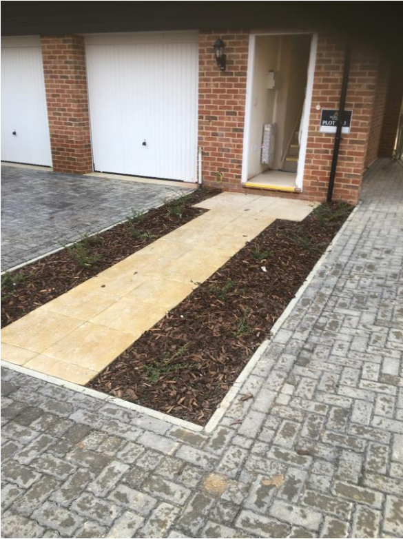
Photographs 5 - 6 , taken on the 4 th February 2020, showing the area of soft landscaping adjacent to the footpath to plot 263 which comprises topsoil over concrete.
