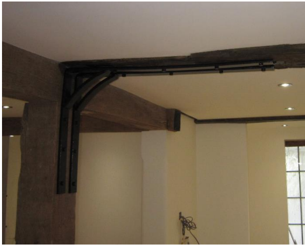
FH4 – showing the steel bracket reinforcing the broken spine beam.
