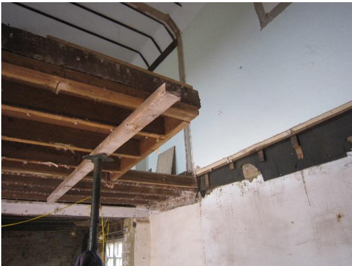
TH6 – the original stairwell
