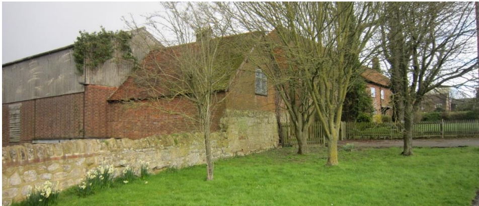
10. Views of the Outhouse and stone wall from the SW
