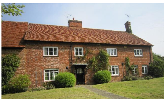
1. Farmhouse - south elevation
