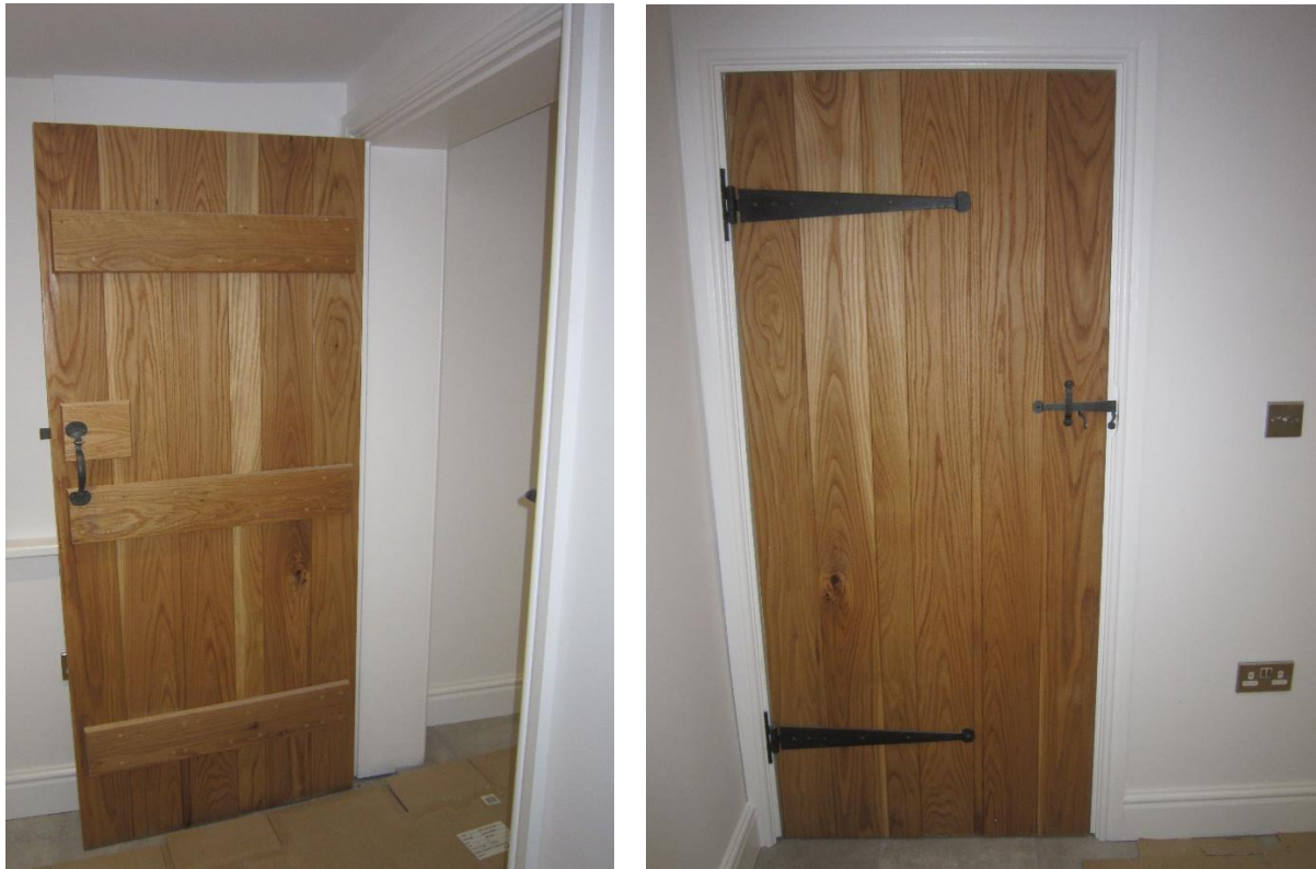
Typical replacement doors showing both sides of the same door
