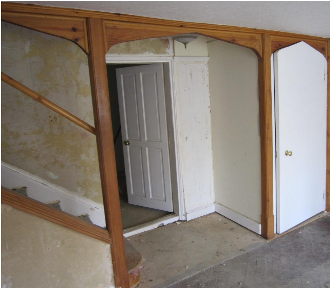
FH1 – showing the modern framework, door and partition – now removed.
