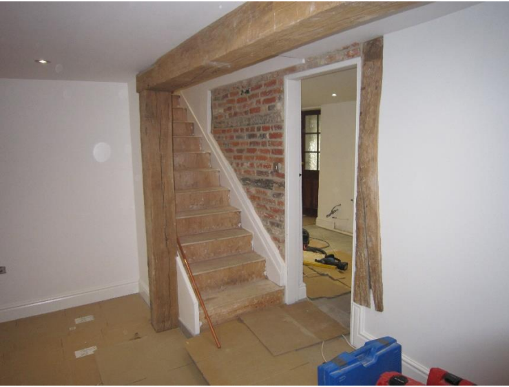
FH3 – existing staircase.
