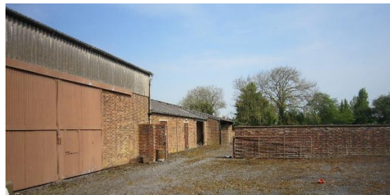
8. Modern farm buildings and yard
