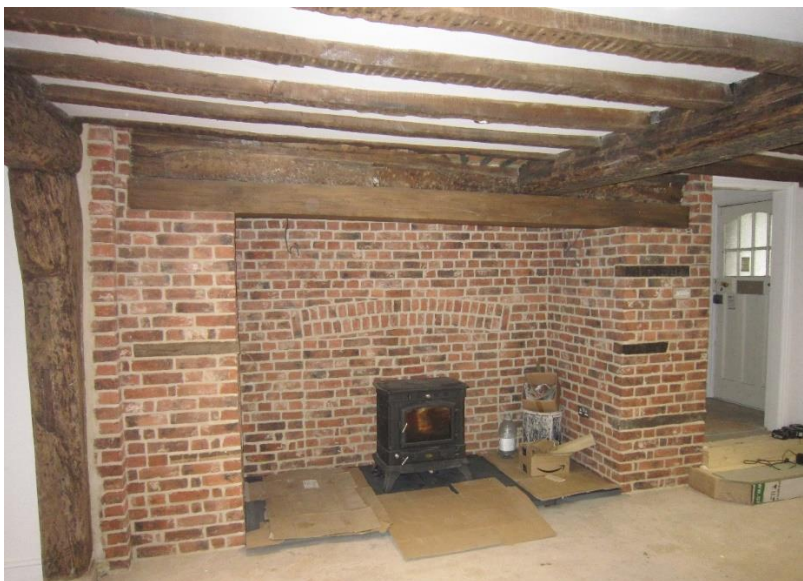
FH5 – showing the refurbished open fireplace and new log burner.
