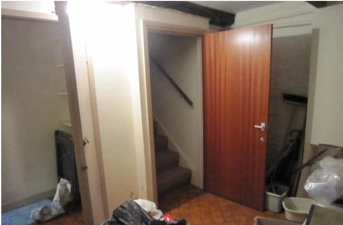
TH5 – original staircase
