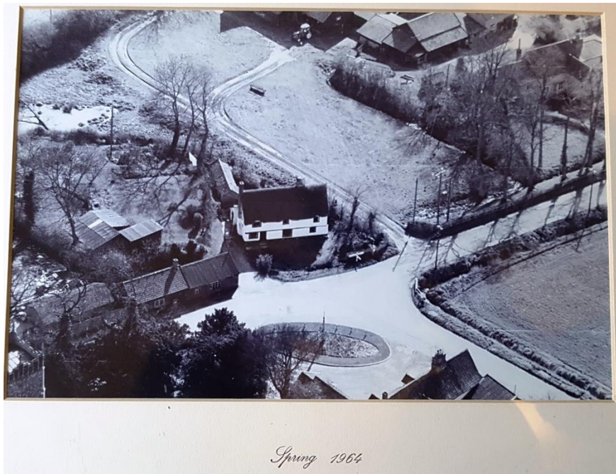
The Old Forge, spring 1964. Lean-to structure not in existence.
