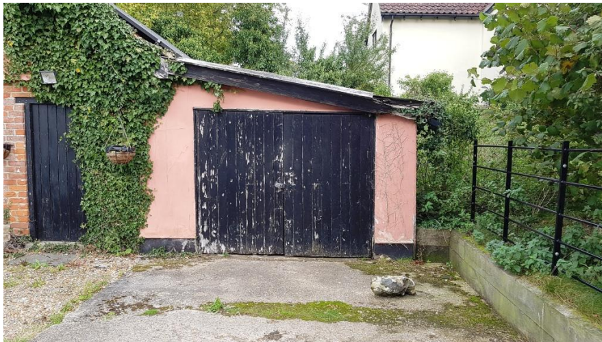
Existing lean-to garage.
