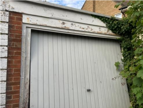
Photograph 5: External of garage
