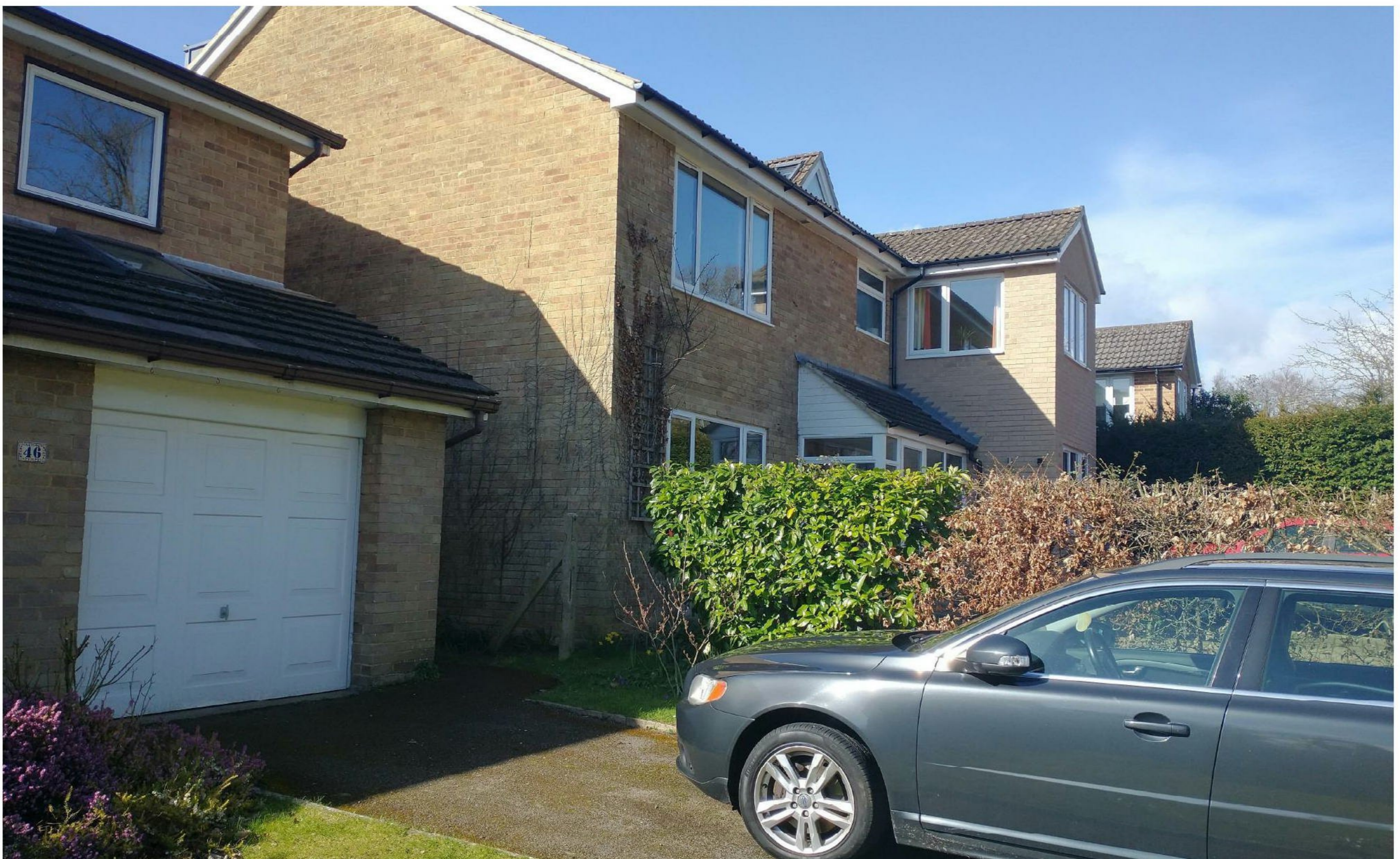
03 View from No.46 showing flank windows at numbers 42 and 44 in context.
