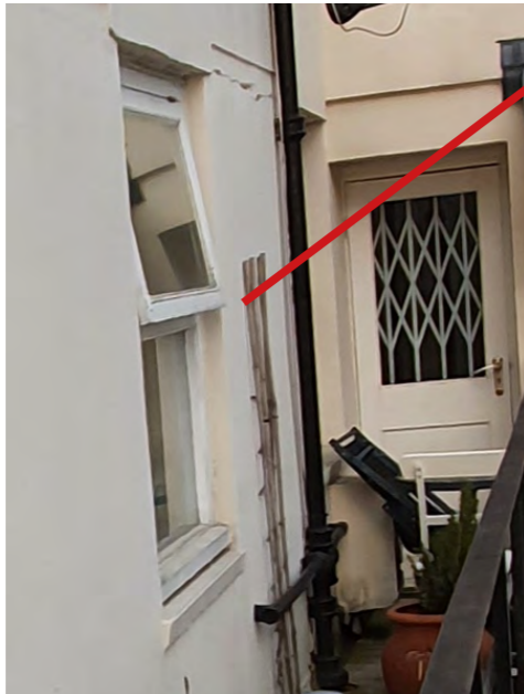
Window to be replaced with white aluminium framed COR 70 hidden sash double doors
