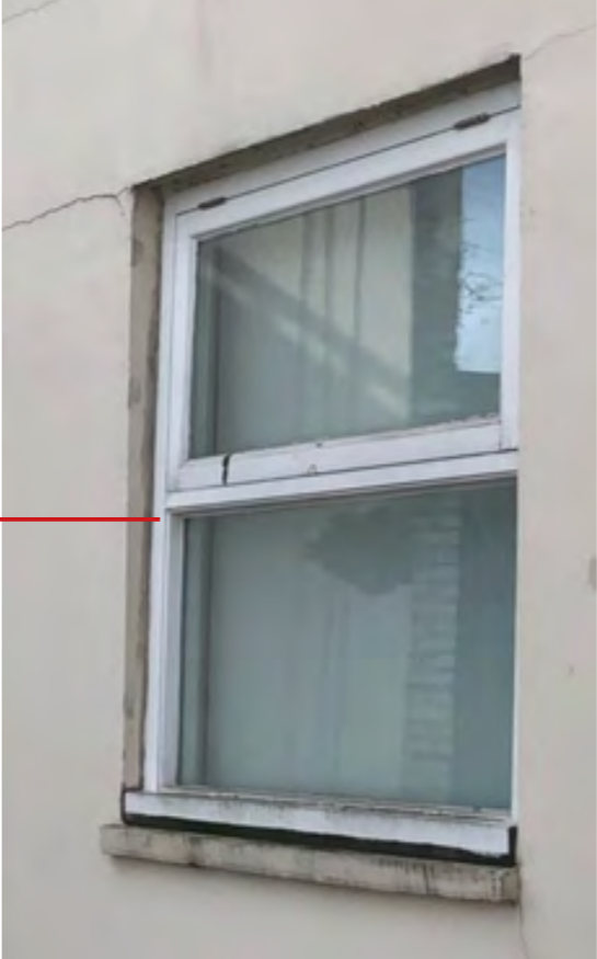
Window to be replaced with white aluminium framed COR 70 hidden sash window
