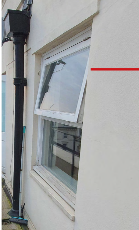
Window to be replaced with white aluminium framed COR 70 hidden sash window
