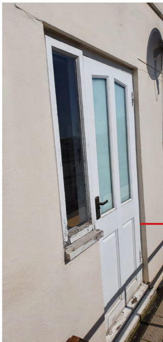
Door and small window to be replaced with white aluminium framed COR 70 hidden sash double doors
