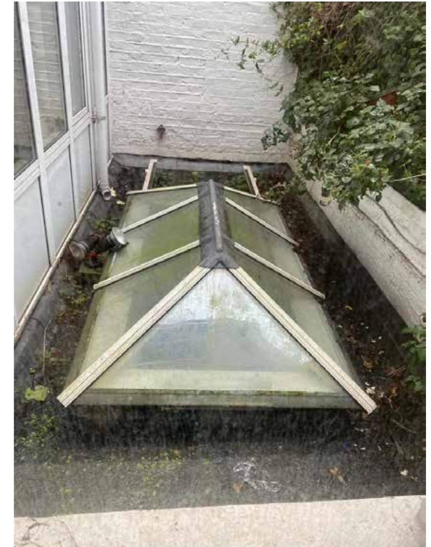
Glazed rooflight and conservatory-like extension to the rear of the property at ground level
