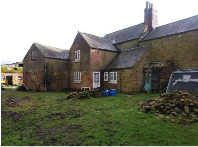
Photograph 1: Farmhouse (north-west elevation)
