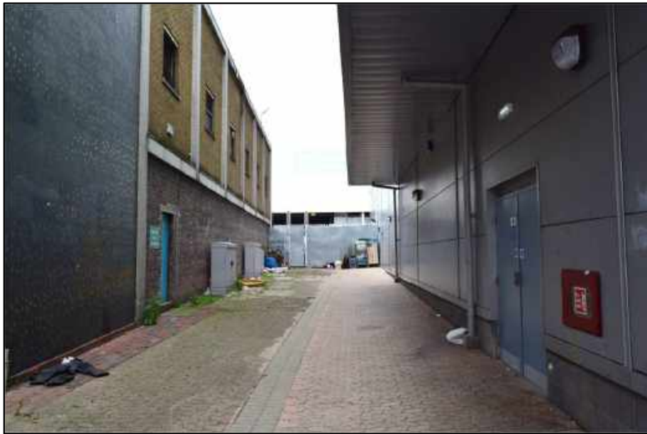
Plate 4: View of alleyway separating the development site from Asda, looking west-southwest
