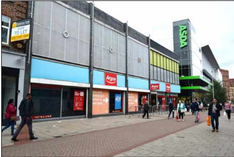
Plate 1: View of the development site (Argos), looking northwest
