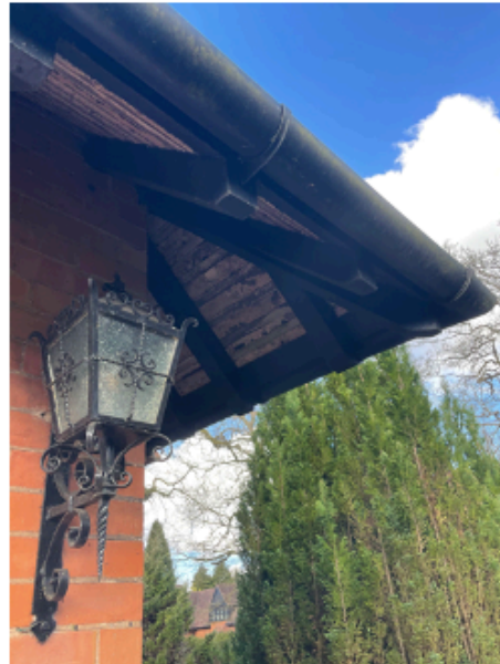
ORIGINAL HOUSE CAST IRON GUTTERING
