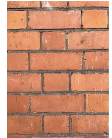
ORIGINAL HOUSE WALL
