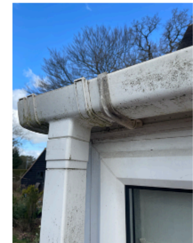
CONSERVATORY – WHITE PLASTIC GUTTERING / DOWNPIPES
