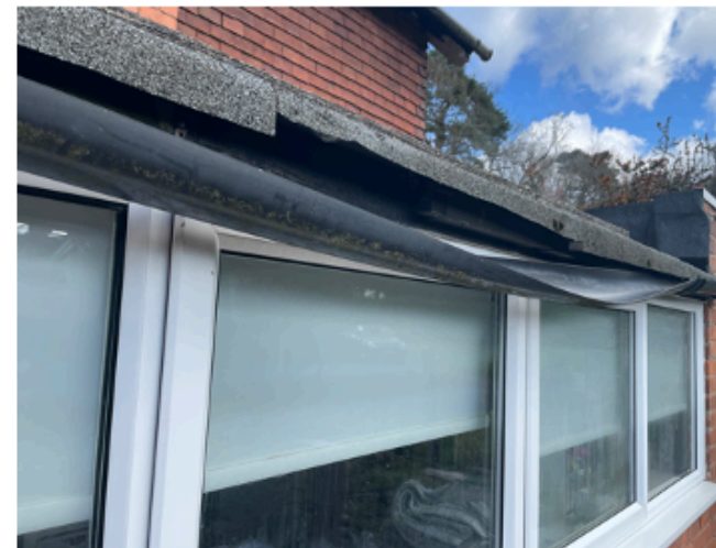
UTILITY ROOM / WC – BLACK PLASTIC GUTTERING
