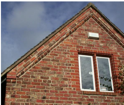
Above left; detail to gable of Onion Farm, showing corbelling to brickwork adjacent to the roof and right; detail of decorative brickwork to the gable of Primrose Cottage.
