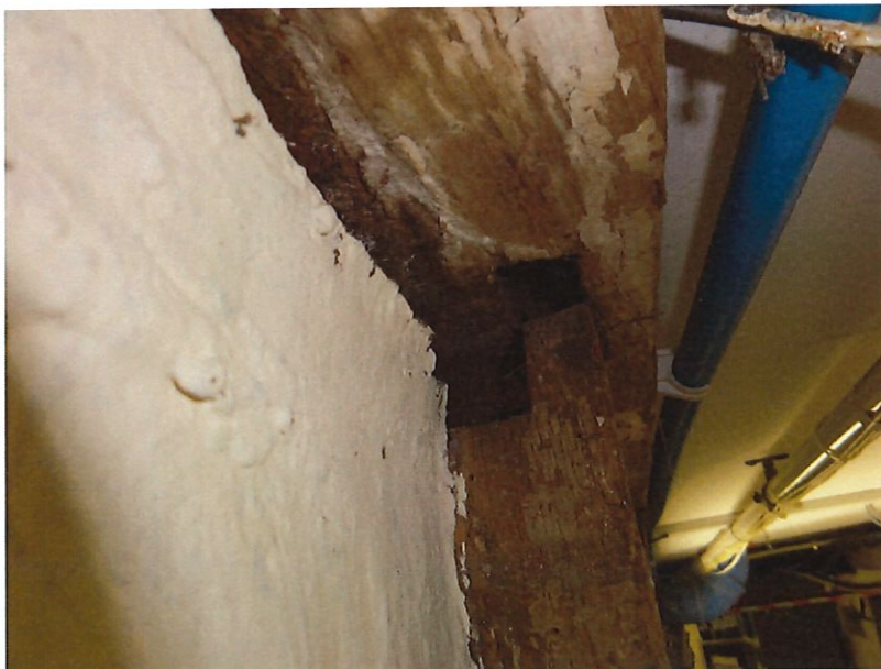
Photo 8 – Vertical stud dropped
