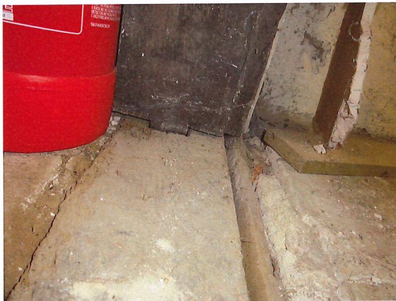
Photo 4 – Threshold dropped exposing tenon
