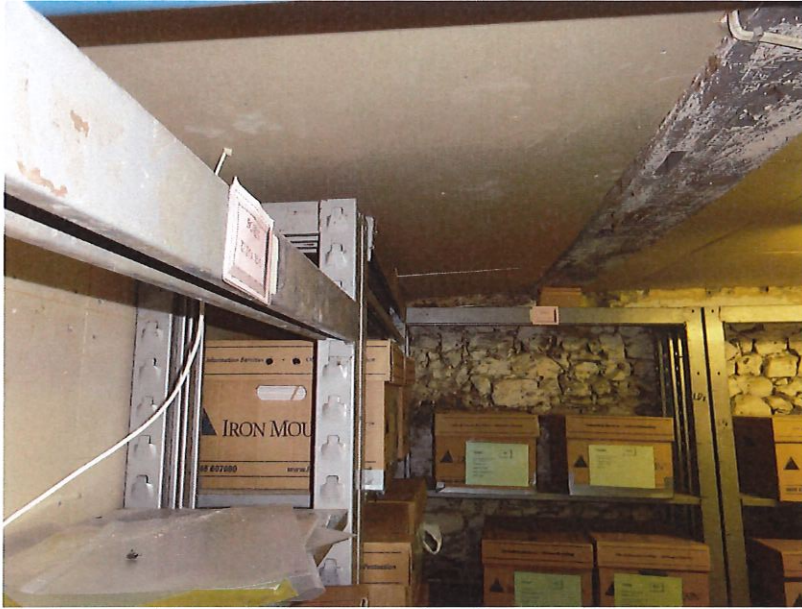
Photo 5 – Archive, note sloping floor (over)
