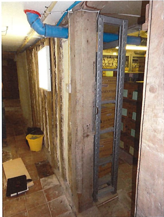
Photo 1 – Timber partition in basement
