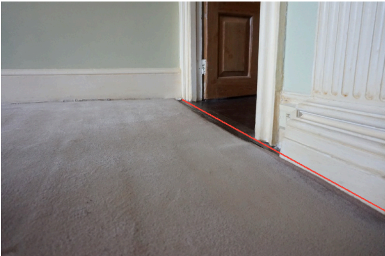
Fig. 12 - Red line taken as plum showing approx. 70mm deflection
