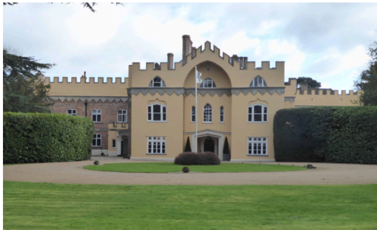
Fig. 4 Contemporary view of the west elevation
