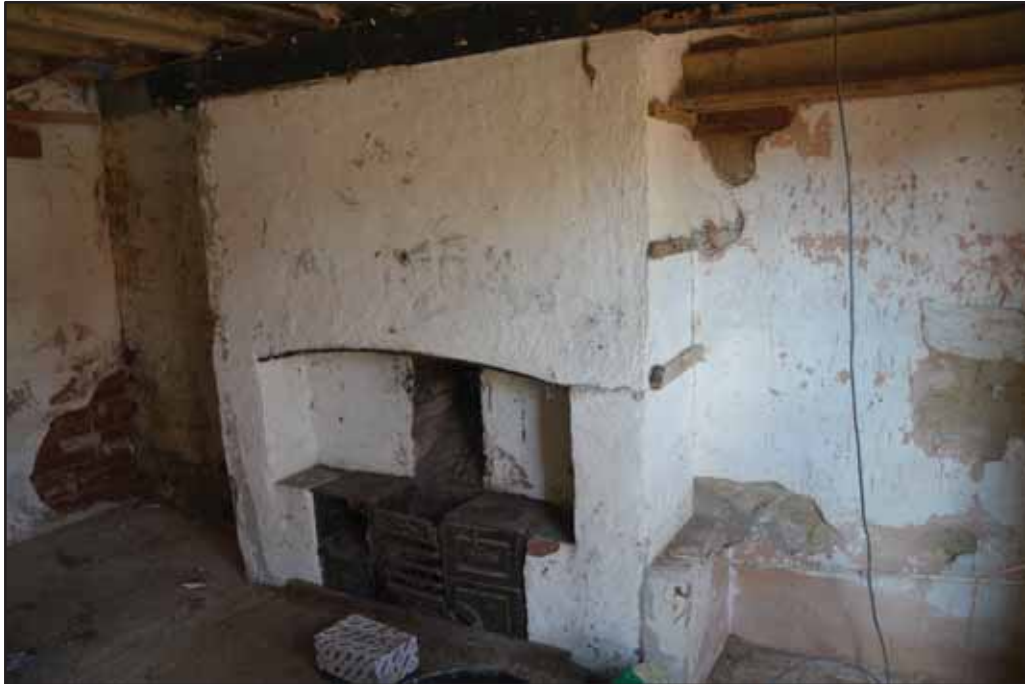
Image 13: Chimney breast and fireplace on north wall
