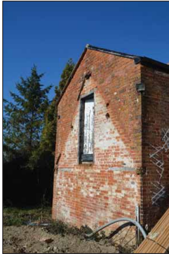
Image 9: South-facing gable end of Swallow Cottage showing position of former extension.
