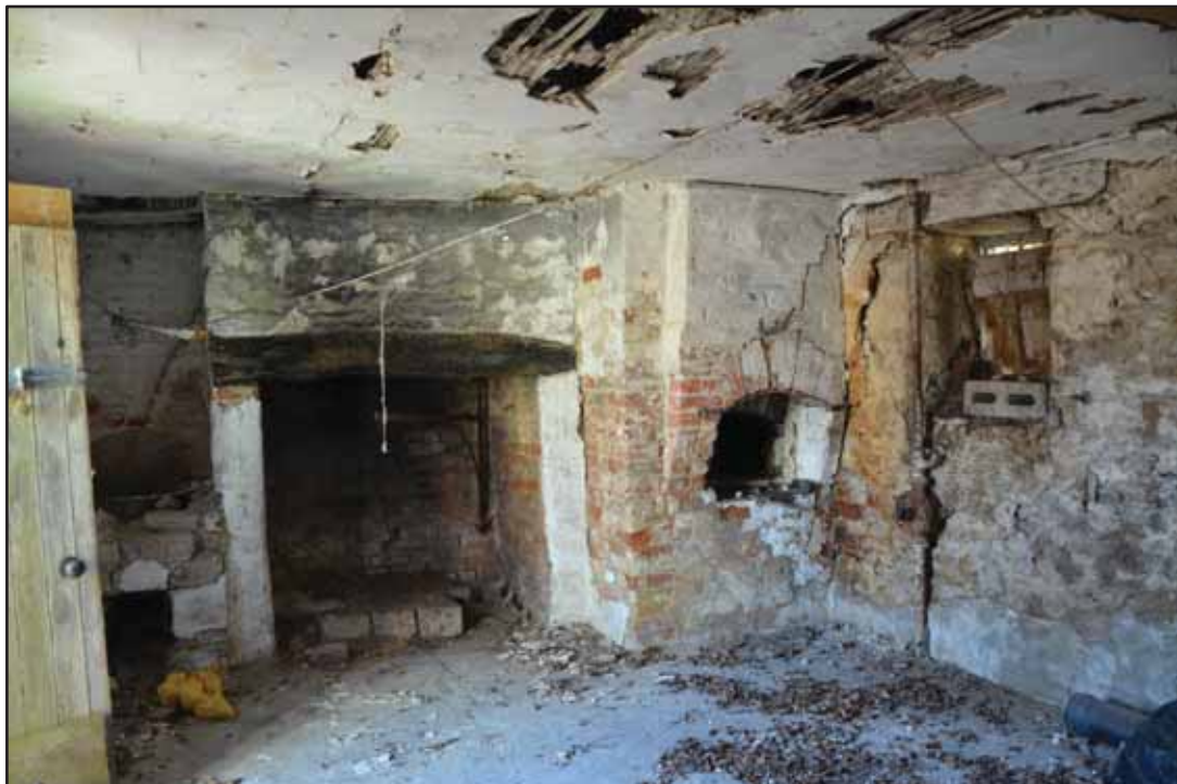
Image 15: South wall with fireplace; brewing equipment to left and oven to right
