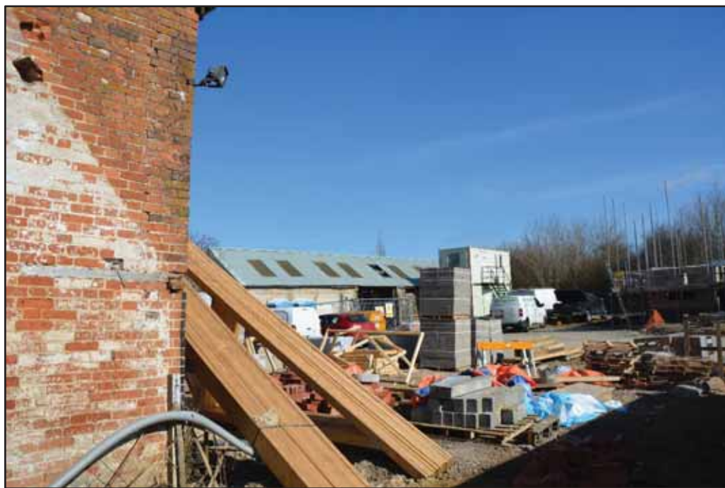
Image 4: View northeast from Swallow Cottage to extant barn
