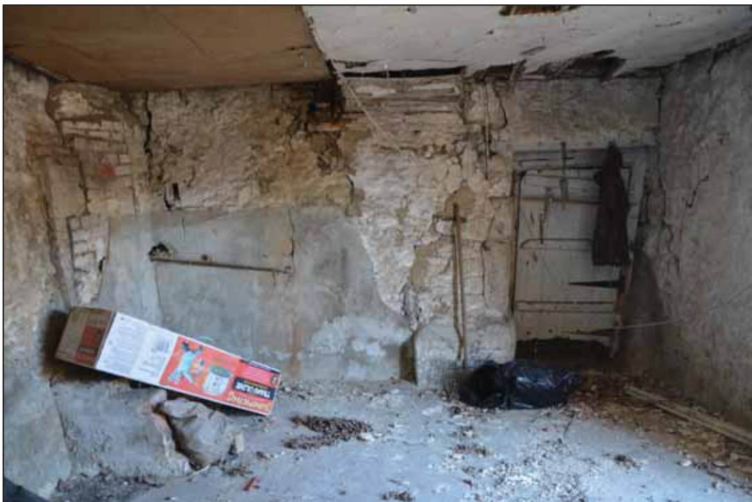
Image 17: Rear wall of Brewhouse showing ceiling remains and rear door
