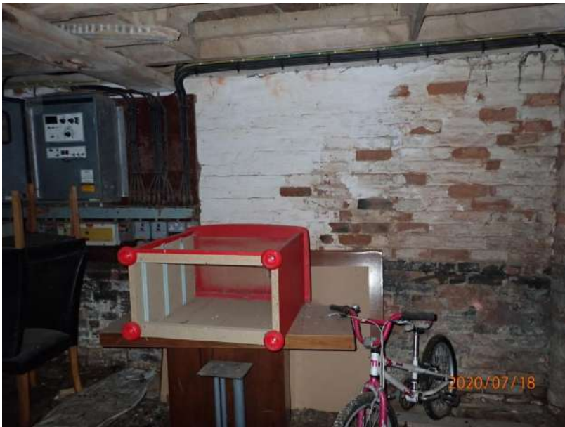
Plate 303: View of the south wall of Cell 13, from the north
