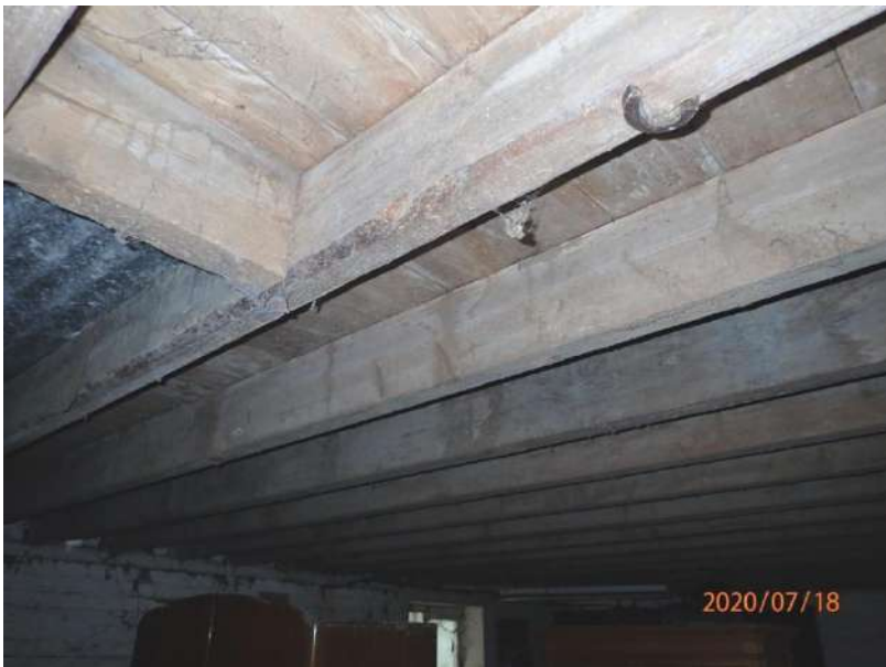
Plate 313: View of the ceiling structure of Cell 13, from the north-west
