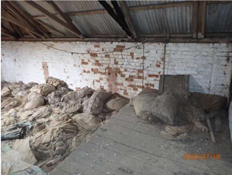
Plate 372: View of the west wall of Cell 17, from the east
