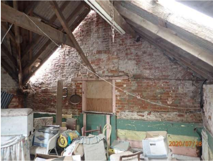
Plate 324: View of the west wall of Cell 14, from the east
