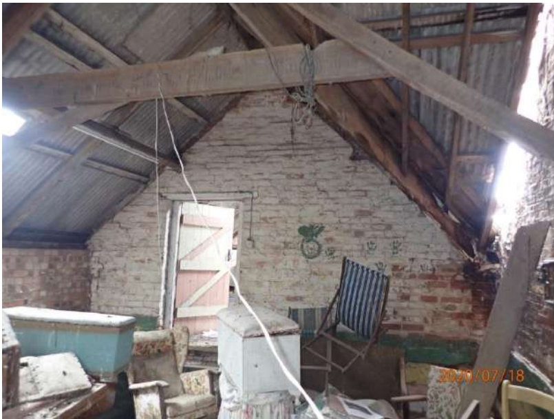
Plate 331: View of the south wall of Cell 14, from the north
