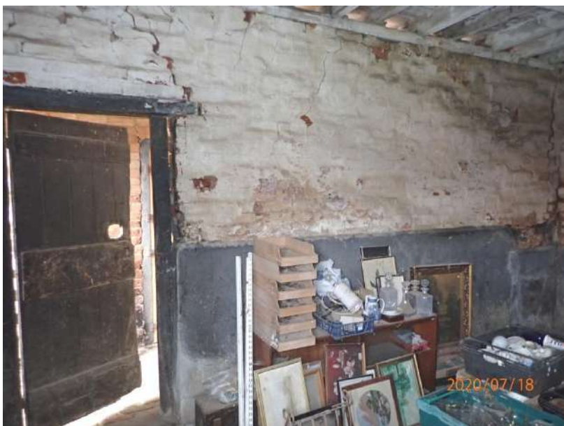
Plate 219: View of the north wall of Cell 8, from the south
