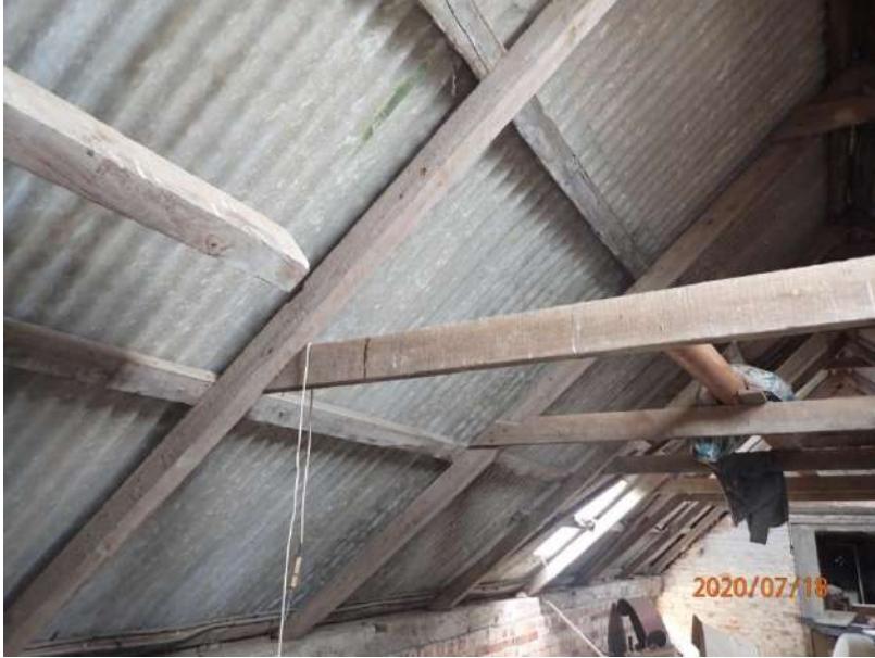
Plate 344: View of the roof supporting structure of Cell 15, from the north
