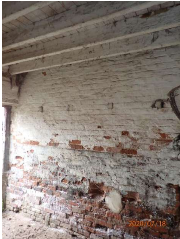
Plate 276: View of the north wall of Cell 12, from the south
