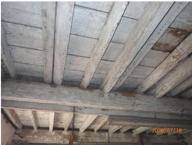
Plate 237: View of the ceiling of Cell 8, from the south
