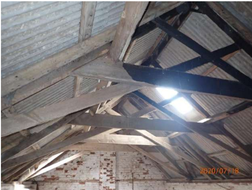
Plate 379: View of the roof supporting structure of Cell 17, from the north
