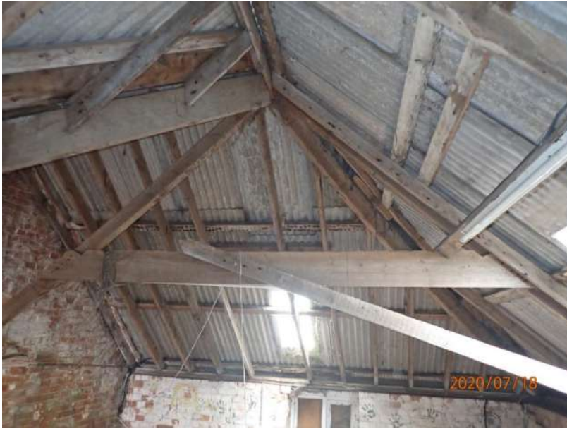
Plate 318: View of the roof supporting structure of Cell 14, from the south
