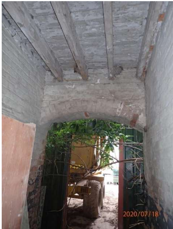
Plate 287: View of the interior of the south tunnel, from the west
