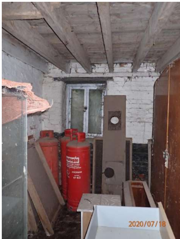
Plate 311: View of the east wall of Cell 13, from the west
