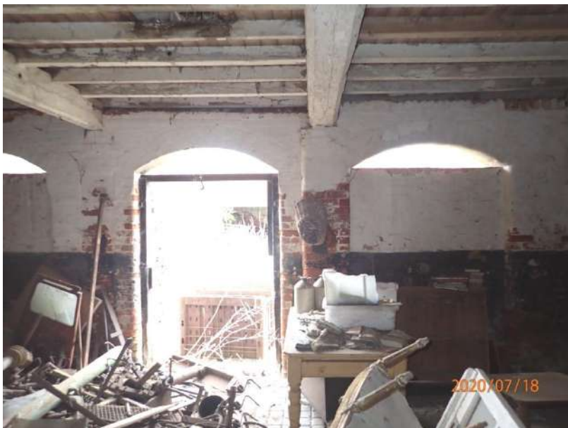
Plate 257: View of the west wall of Cell 10, from the east
