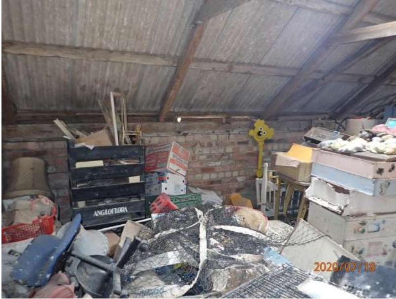
Plate 336: View of the west wall of Cell 15, from the east
