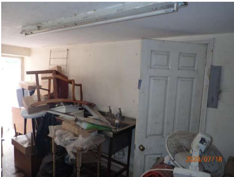
Plate 205: View of the south wall of Cell 6, from the west
