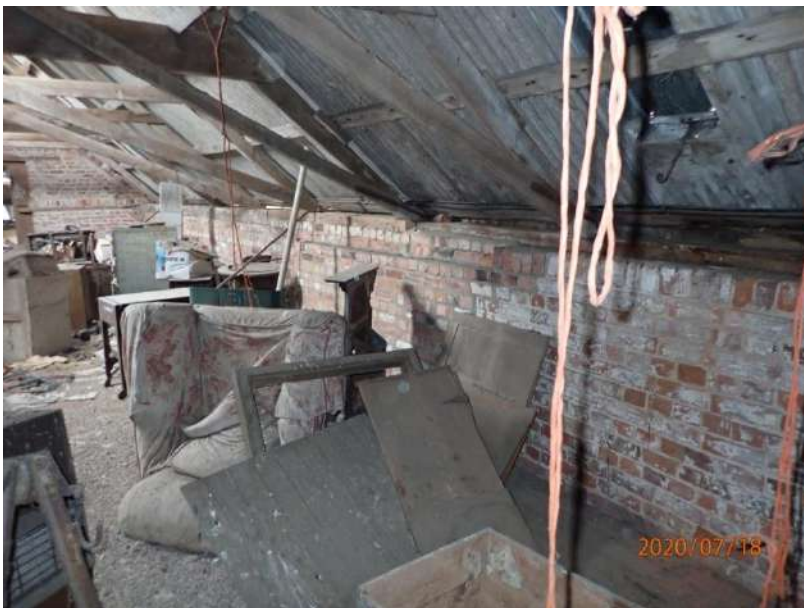
Plate 365: View of the east wall of Cell 16, from the south
