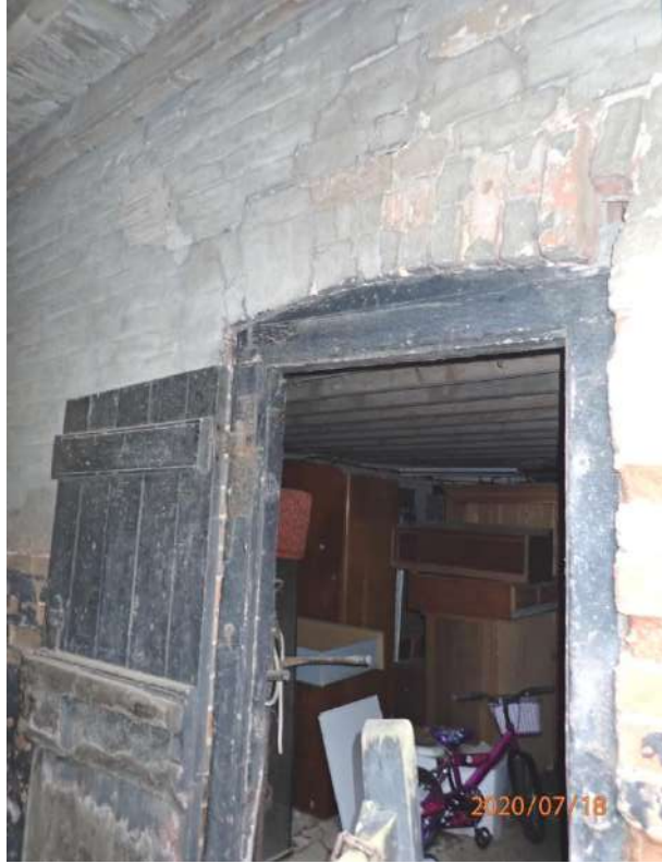
Plate 293: View of the interior of the south tunnel, from the west
