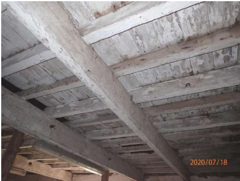
Plate 236: View of the ceiling of Cell 8, from the east
