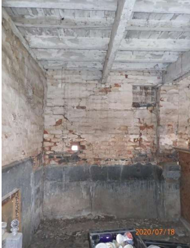
Plate 221: View of the east wall of Cell 8, from the west
