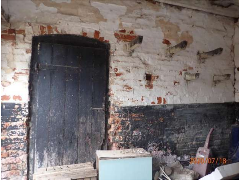
Plate 266: View of the north wall of Cell 11, from the south
