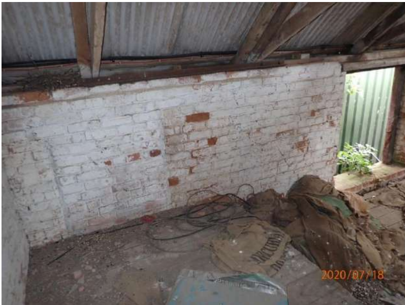
Plate 367: View of the east wall of Cell 17, from the west
