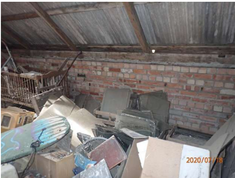
Plate 357: View of the west wall of Cell 16, from the east
