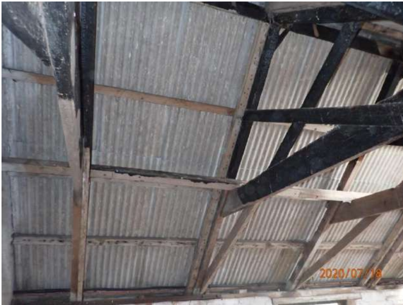
Plate 380: View of the roof supporting structure of Cell 17, from the west
