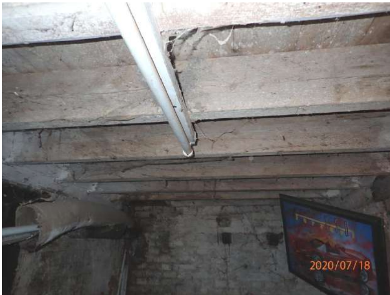
Plate 215: View of the ceiling of Cell 7, from the east
