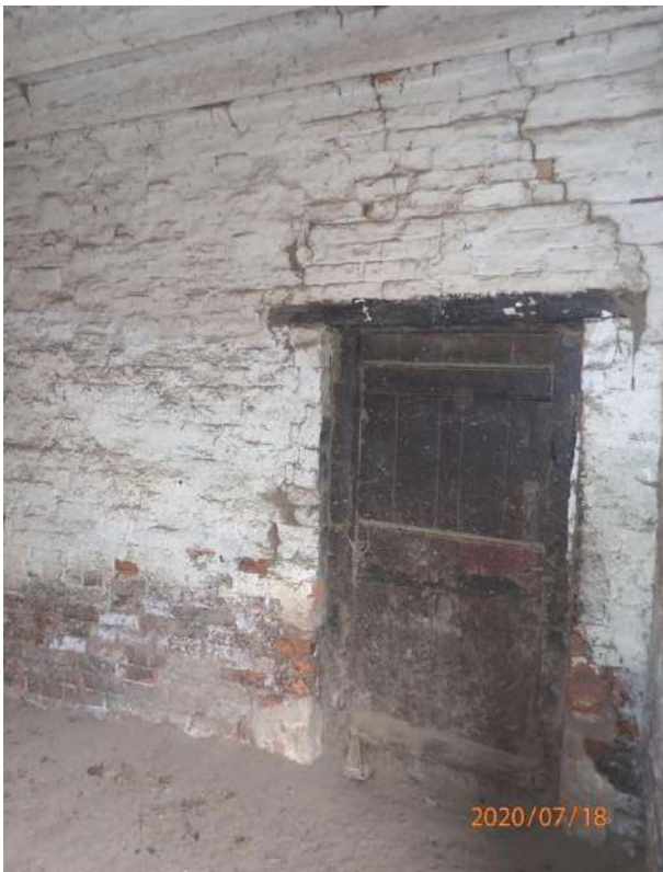
Plate 278: View of the south wall of Cell 12, from the north
