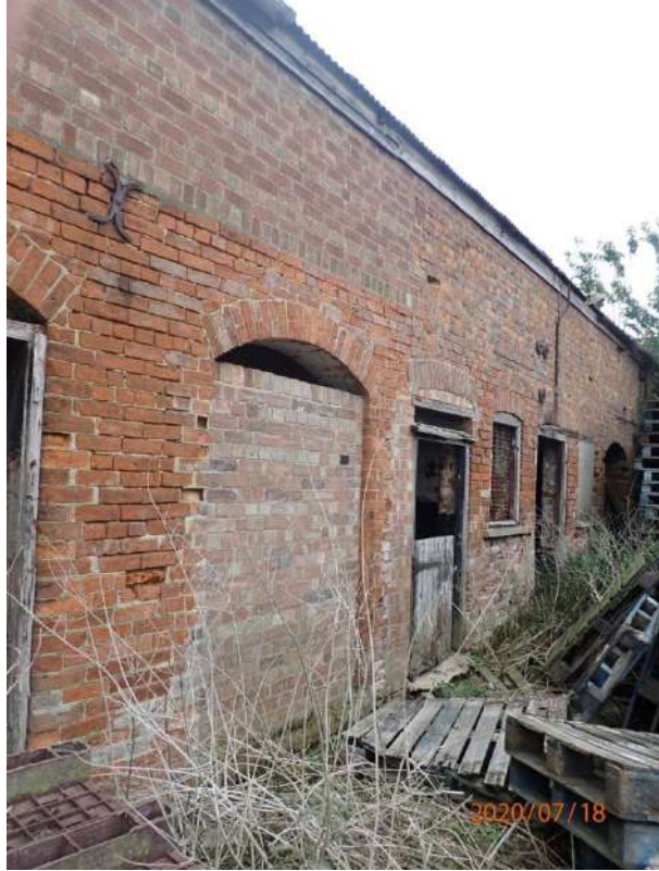
Plate 199: View of the West Elevation of the East Range, from the north
