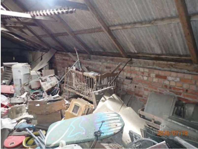
Plate 358: View of the west wall of Cell 16, from the north
