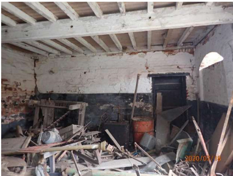
Plate 253: View of the south wall of Cell 10, from the north
