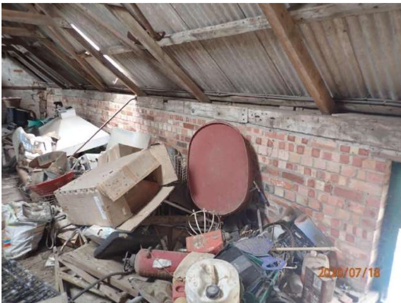
Plate 339: View of the east wall of Cell 15, from the south
