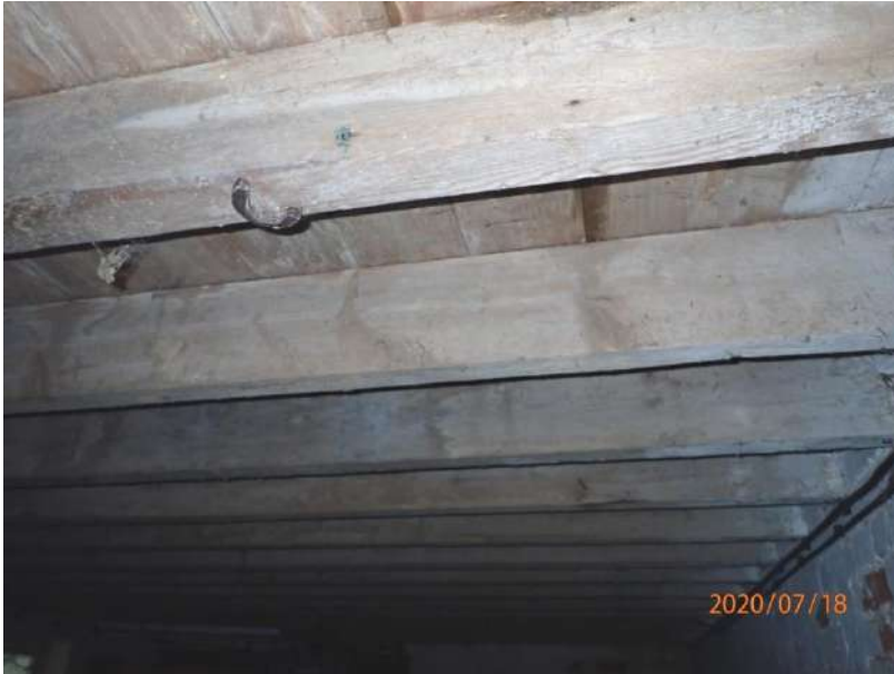
Plate 312: View of the ceiling structure of Cell 13, from the north
