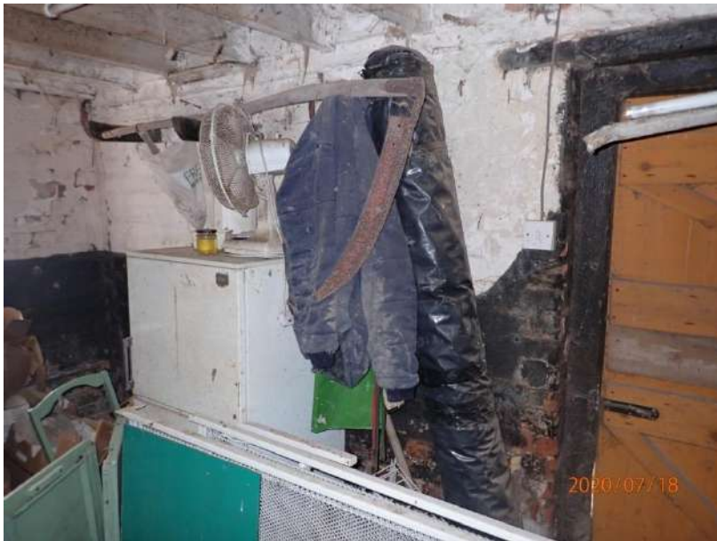
Plate 212: View of the south wall of Cell 7, from the north-west
