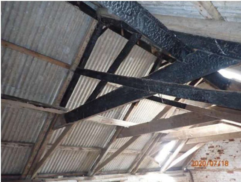
Plate 381: View of the roof supporting structure of Cell 17, from the north
