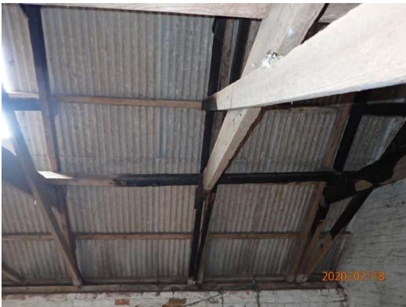
Plate 377: View of the roof supporting structure of Cell 17, from the east
