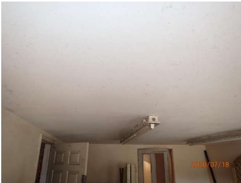
Plate 201: View of the ceiling of Cell 6, from the east
