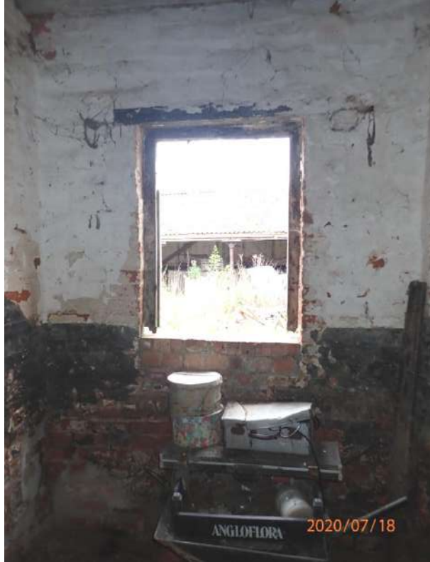
Plate 247: View of the west wall of Cell 9, from the east
