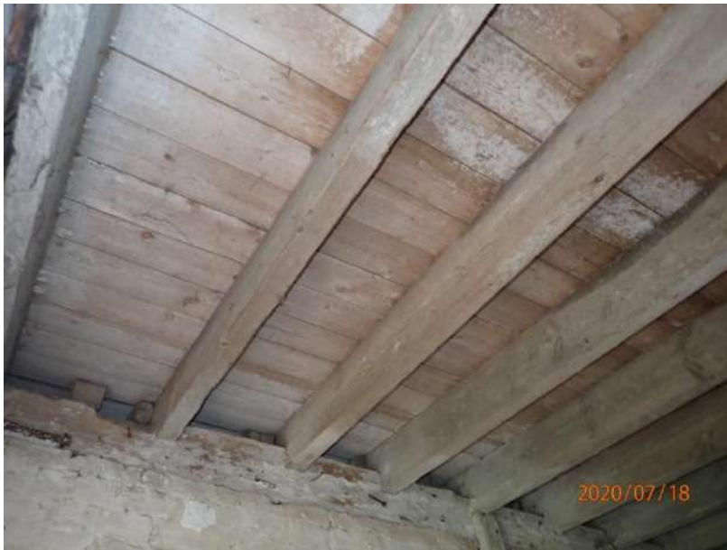
Plate 250: View of the ceiling of Cell 9, from the south
