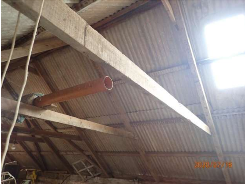
Plate 350: View of the roof supporting structure of Cell 15, from the north
