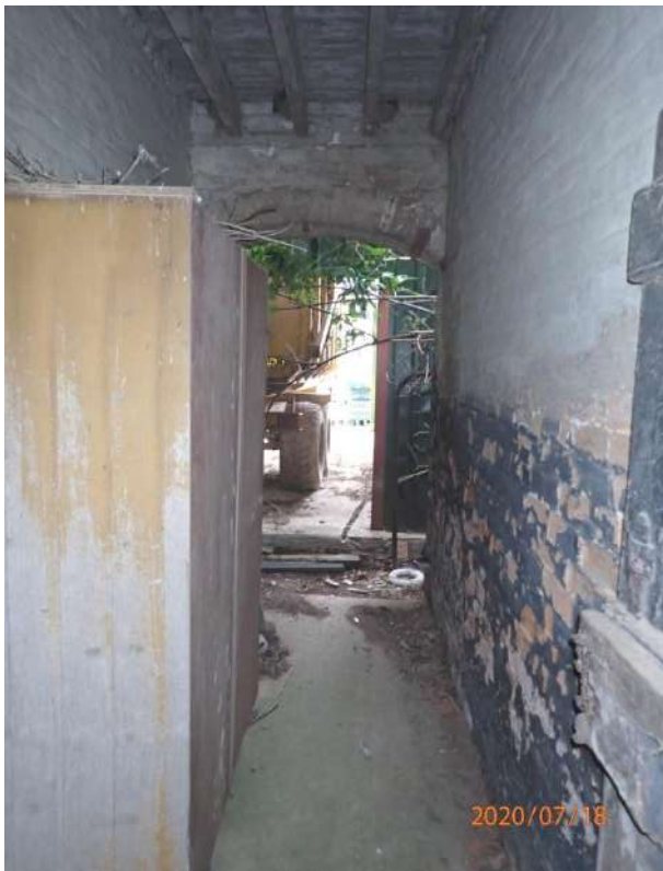
Plate 285: View of the interior of the south tunnel, from the west
