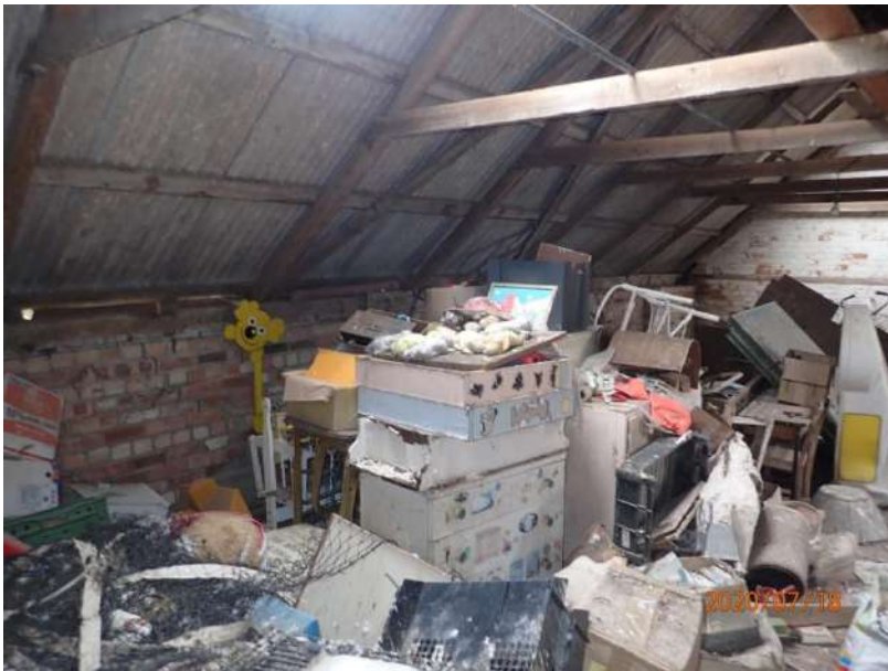
Plate 337: View of the west wall of Cell 15, from the south-east
