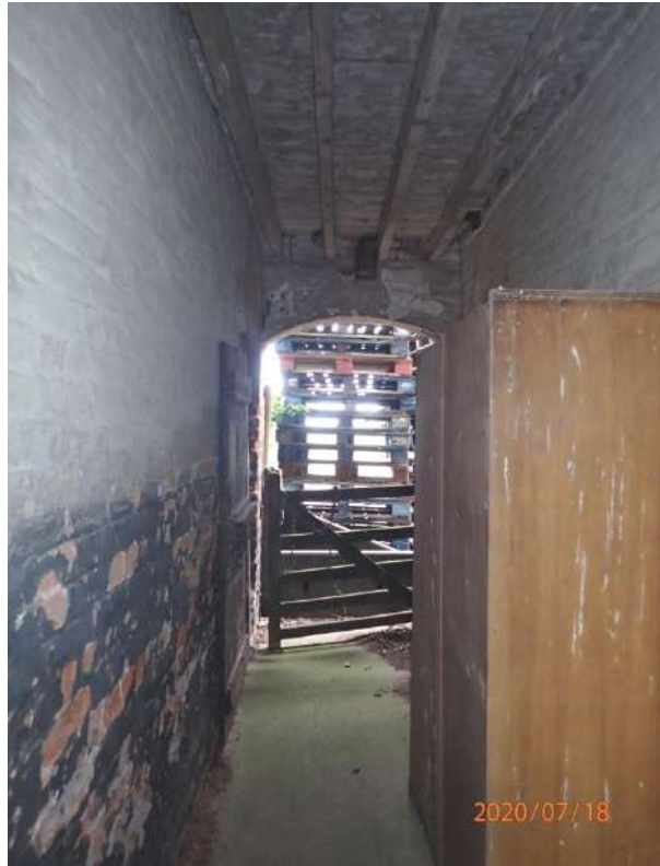
Plate 283: View of the interior of the south tunnel, from the east
