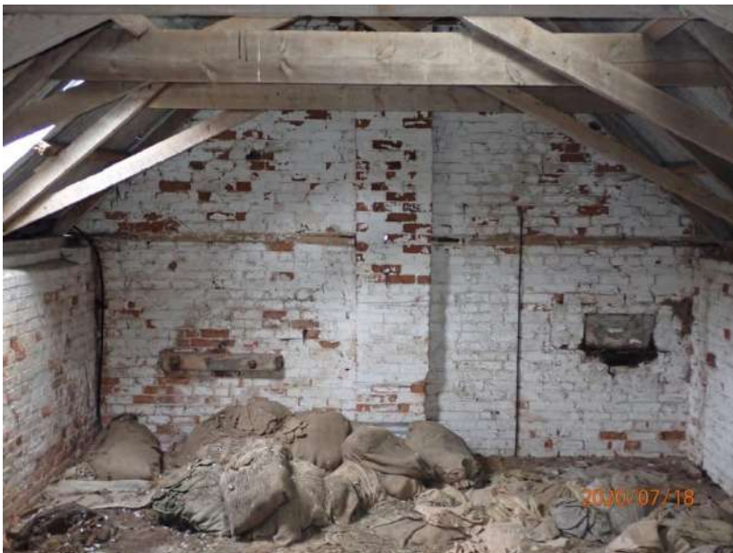
Plate 369: View of the south wall of Cell 17, from the north
