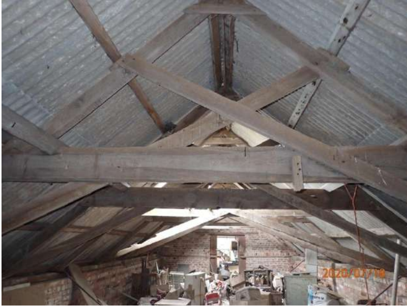
Plate 362: View of the roof supporting structure of Cell 16, from the south
