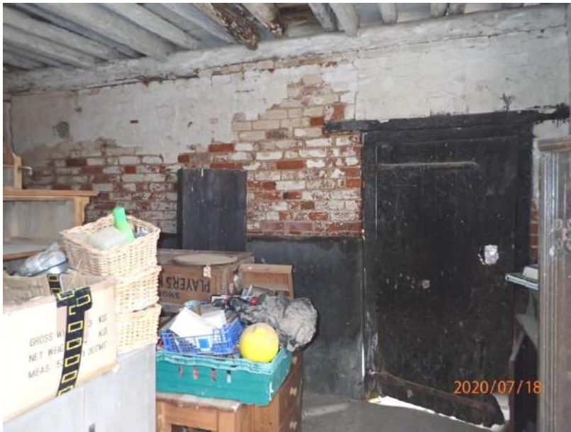
Plate 227: View of the south wall of Cell 8, from the north
