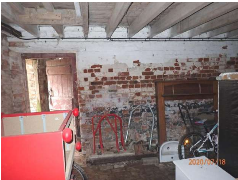
Plate 309: View of the west wall of Cell 13, from the east
