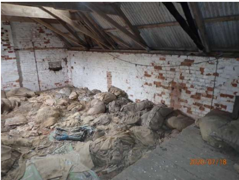
Plate 373: View of the west wall of Cell 17, from the north
