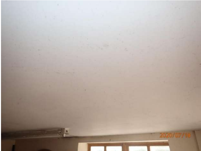
Plate 202: View of the ceiling of Cell 6, from the south
