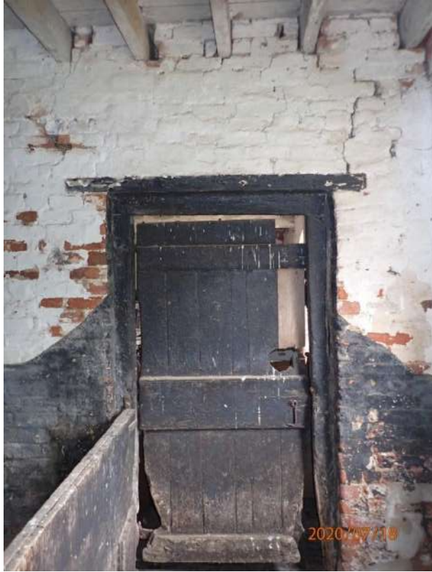
Plate 242: View of the south wall of Cell 9, from the north
