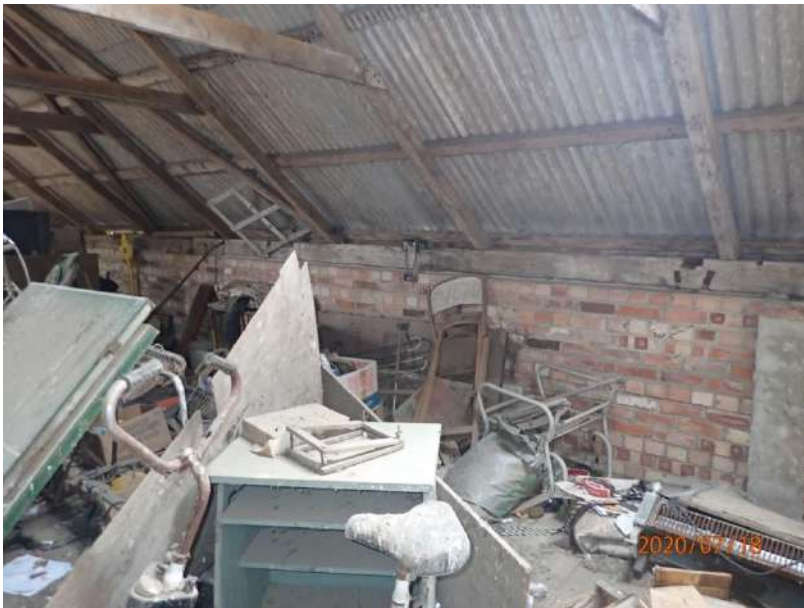
Plate 341: View of the west wall of Cell 15, from the north
