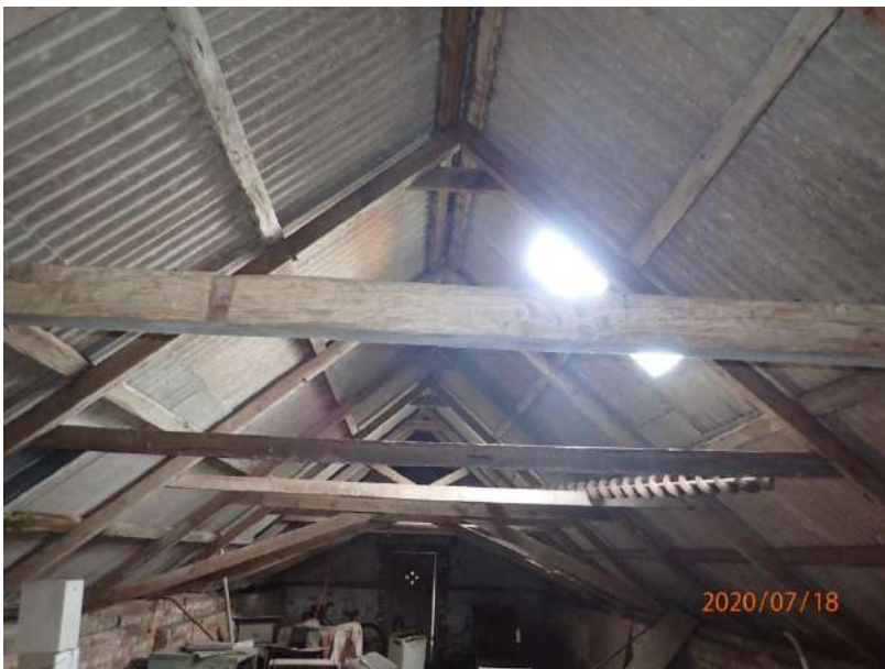
Plate 353: View of the roof supporting structure of Cell 16, from the north
