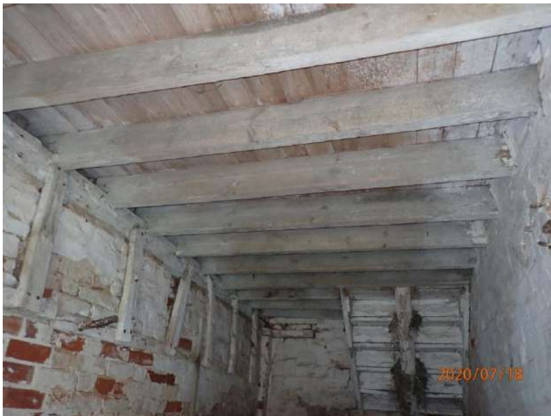
Plate 249: View of the ceiling of Cell 9, from the west
