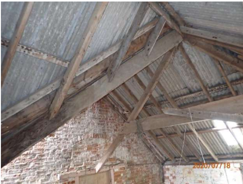
Plate 319: View of the roof supporting structure of Cell 14, from the south-east
