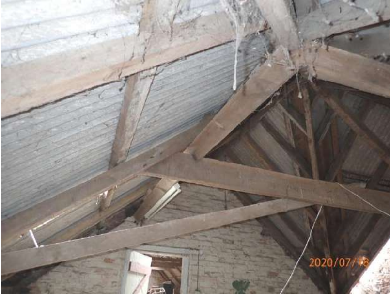
Plate 326: View of the roof supporting structure of Cell 14, from the north
