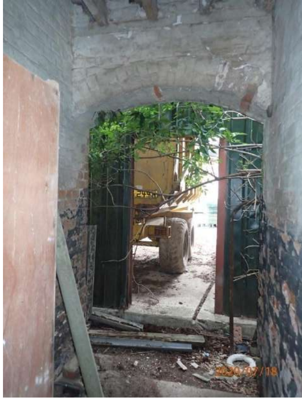
Plate 286: View of the interior of the south tunnel, from the west
