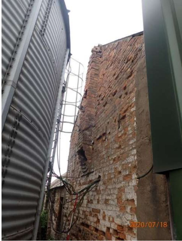
Plate 172: View of the South Elevation of the East Range, from the east
