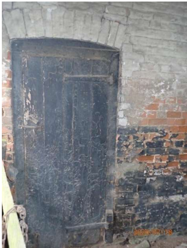
Plate 294: View of the interior of the south tunnel, from the west
