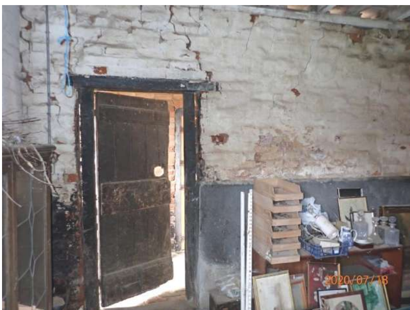
Plate 220: View of the north wall of Cell 8, from the south
