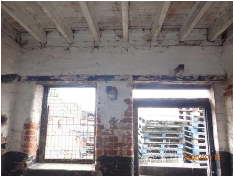
Plate 269: View of the west wall of Cell 11, from the east
