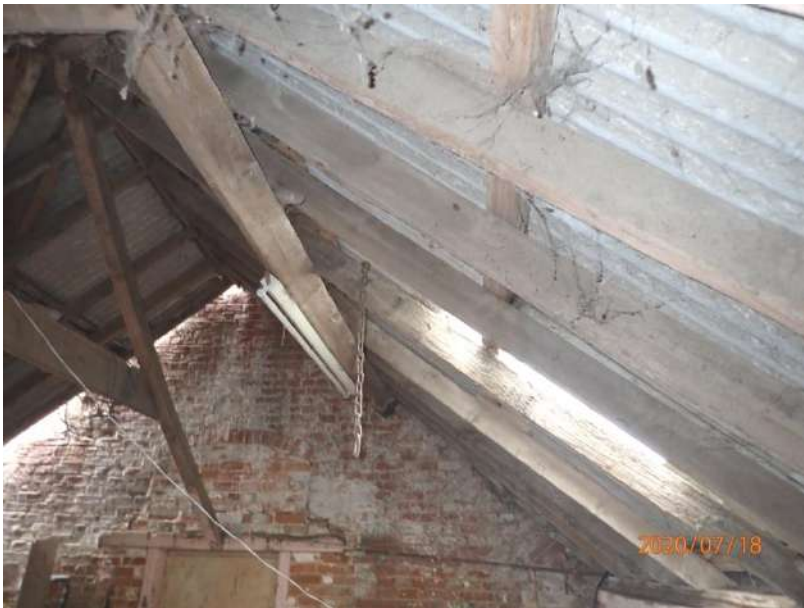
Plate 329: View of the roof supporting structure of Cell 14, from the east
