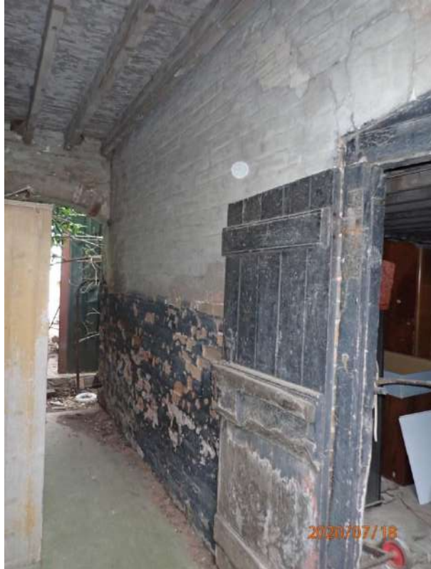
Plate 291: View of the interior of the south tunnel, from the west
