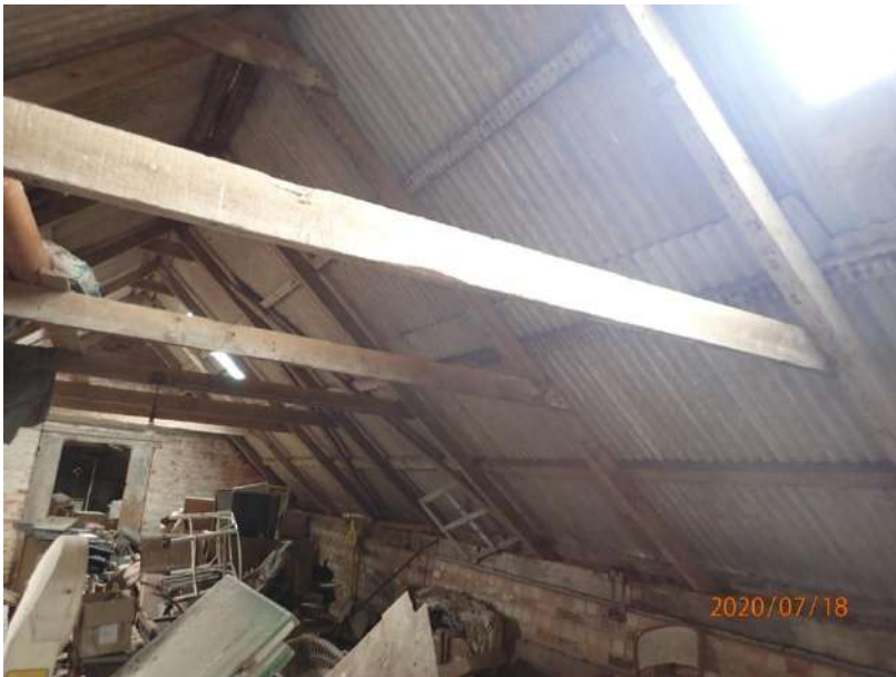
Plate 345: View of the roof supporting structure of Cell 15, from the north
