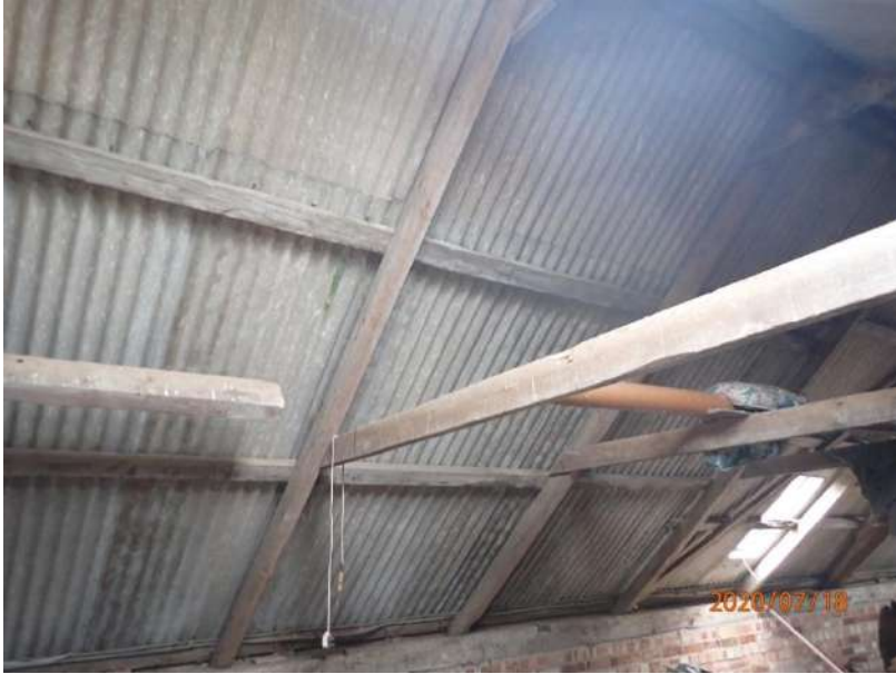
Plate 348: View of the roof supporting structure of Cell 15, from the north
