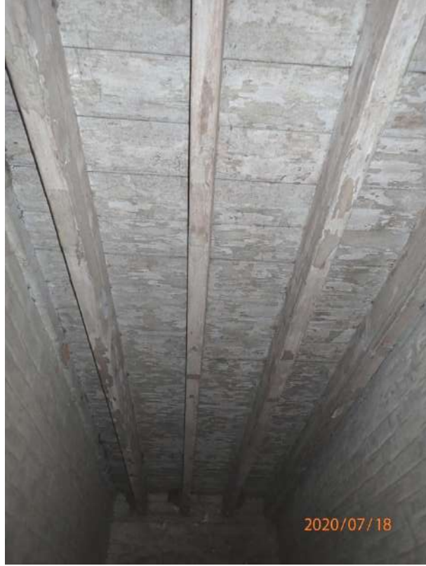
Plate 288: View of the interior of the south tunnel, from the west
