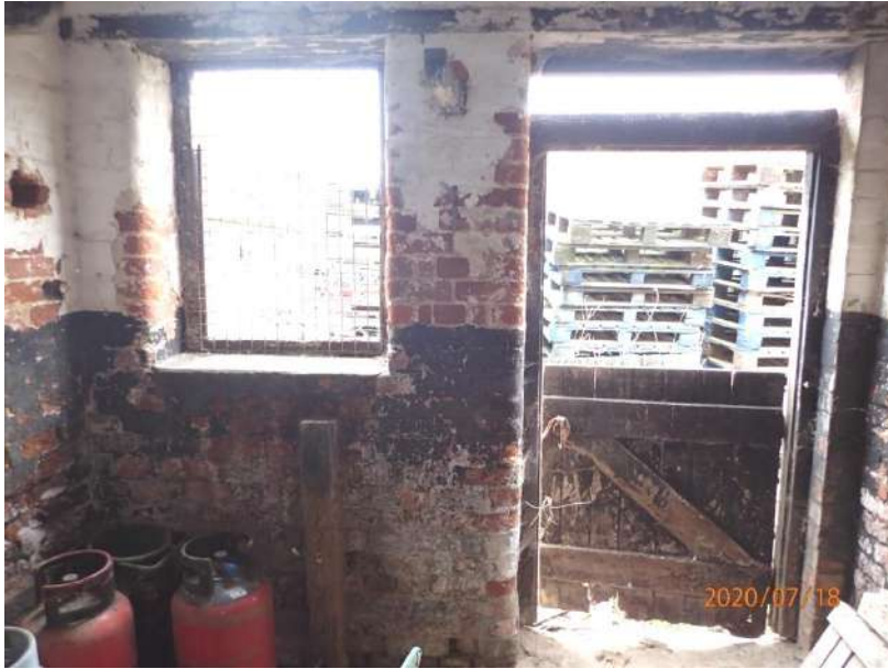
Plate 268: View of the west wall of Cell 11, from the east
