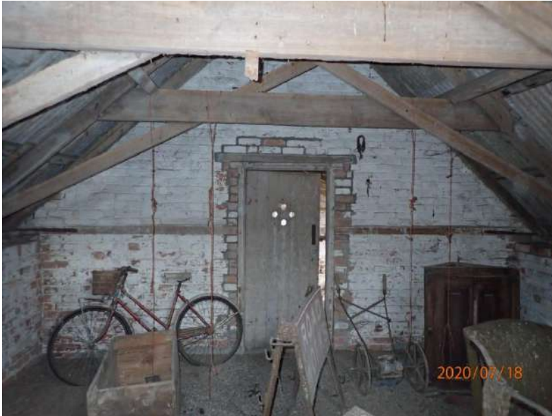
Plate 360: View of the south wall of Cell 16, from the north
