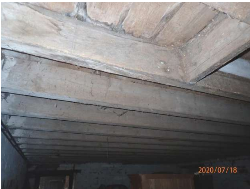
Plate 315: View of the ceiling structure of Cell 13, from the north
