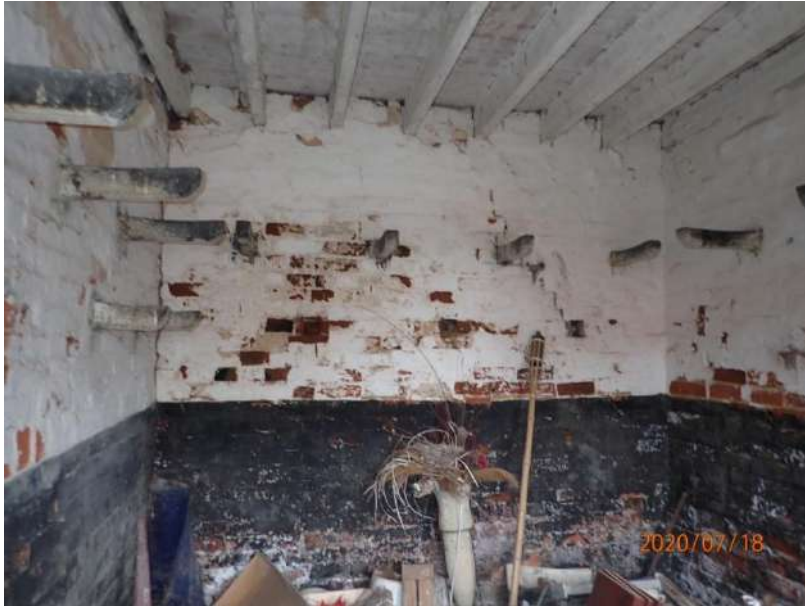
Plate 264: View of the east wall of Cell 11, from the west
