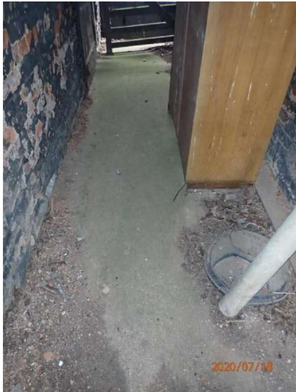
Plate 282: View of the interior of the south tunnel, from the east
