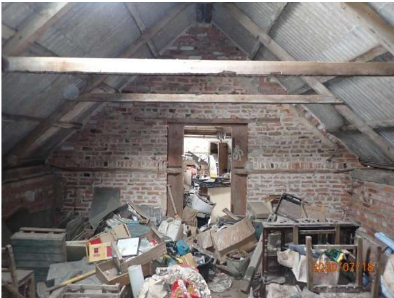
Plate 359: View of the north wall of Cell 16, from the south
