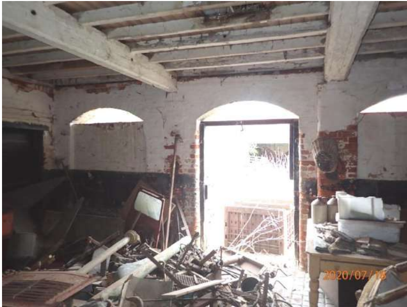
Plate 256: View of the west wall of Cell 10, from the east
