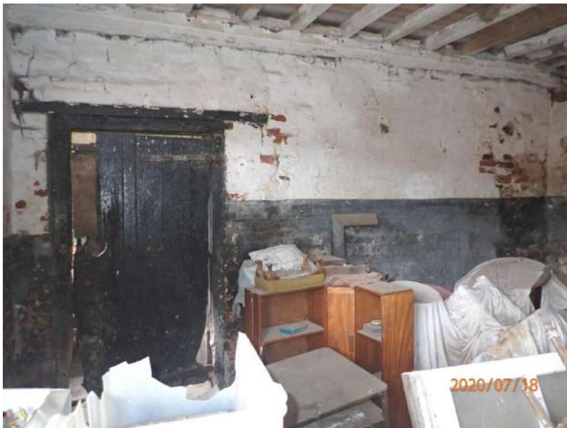
Plate 255: View of the north wall of Cell 10, from the south
