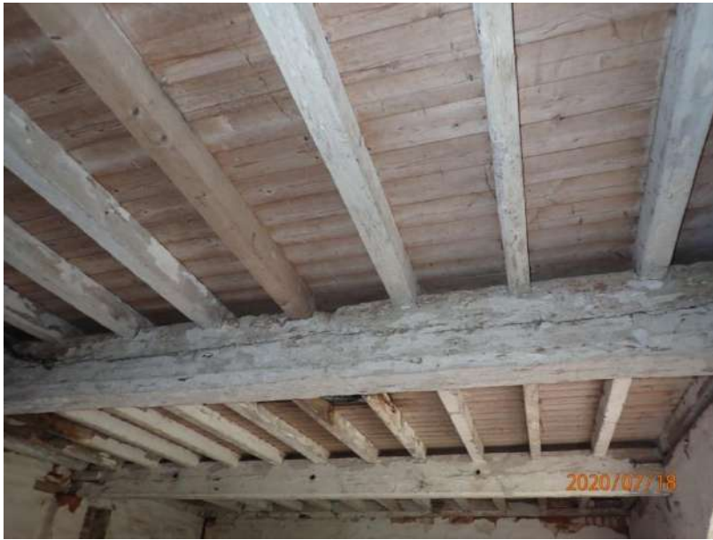
Plate 258: View of the ceiling of Cell 10, from the south
