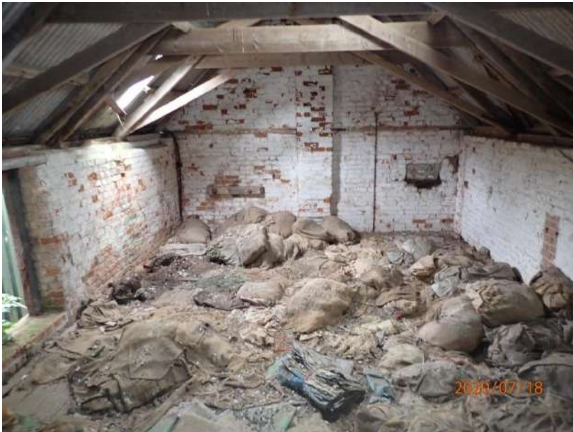
Plate 371: General view of the interior of Cell 17, from the north
