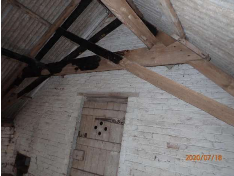
Plate 376: View of the north wall of Cell 17, from the east
