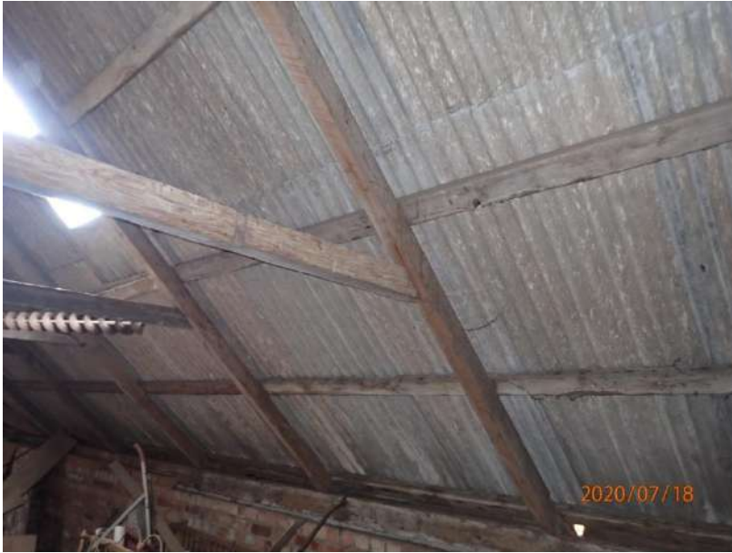
Plate 354: View of the roof supporting structure of Cell 16, from the north
