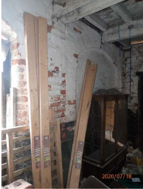
Plate 232: View of the west wall of Cell 8, from the east
