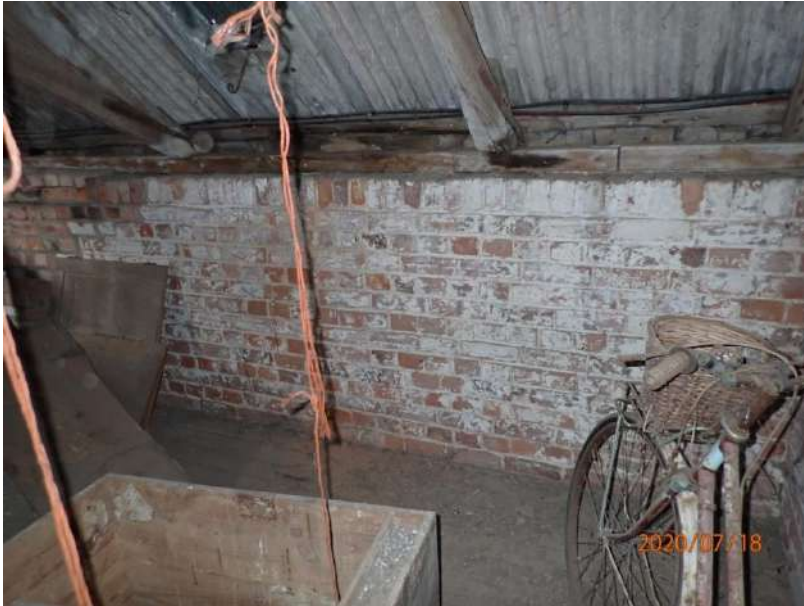
Plate 364: View of the east wall of Cell 16, from the south
