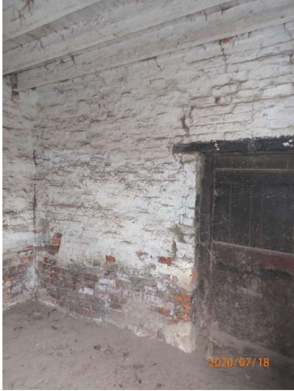
Plate 279: View of the south wall of Cell 12, from the north
