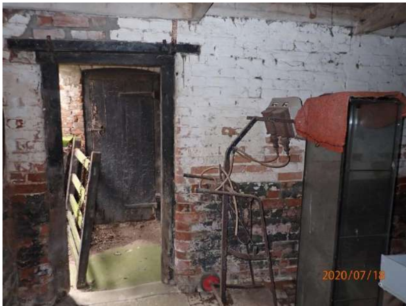
Plate 301: View of the north wall of Cell 13, from the south
