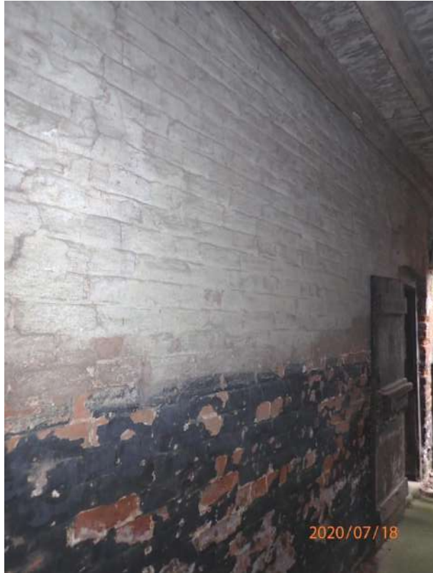
Plate 290: View of the interior of the south tunnel, from the west
