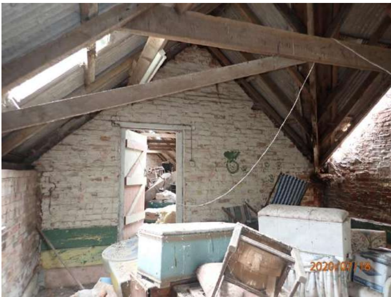
Plate 325: View of the south wall of Cell 14, from the north
