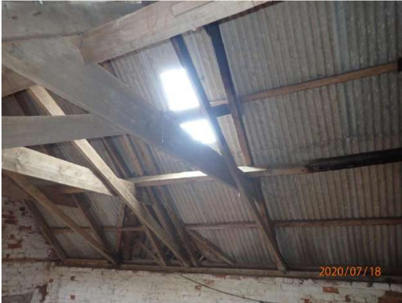
Plate 378: View of the roof supporting structure of Cell 17, from the east
