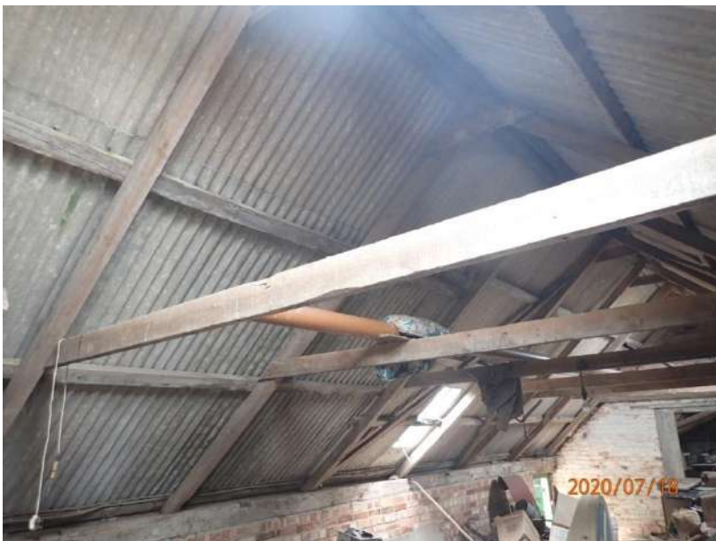
Plate 347: View of the roof supporting structure of Cell 15, from the north
