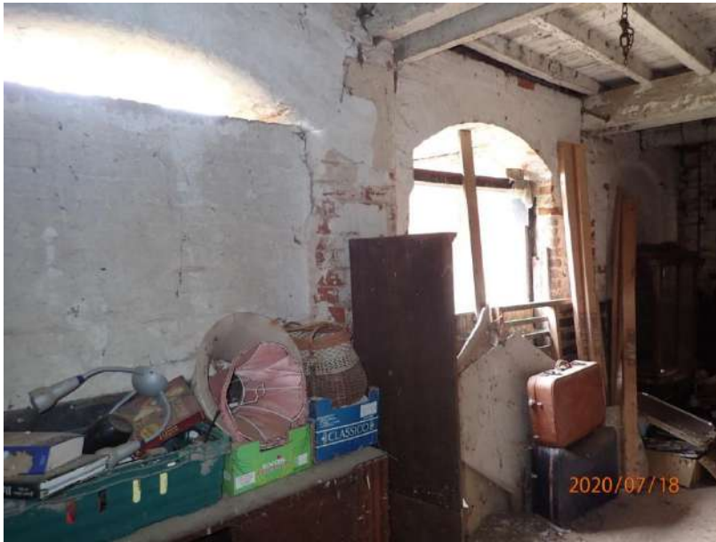
Plate 229: View of the west wall of Cell 8, from the south-east
