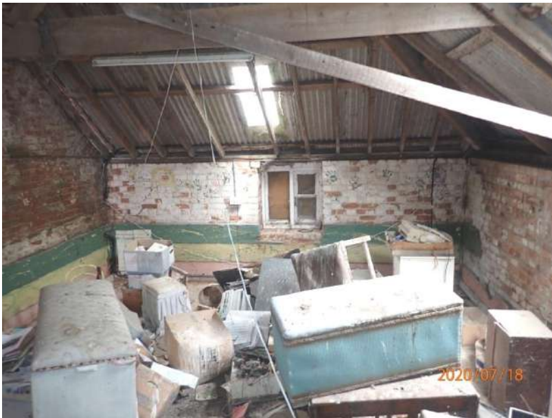
Plate 317: General view of the interior of Cell 14, from the south
