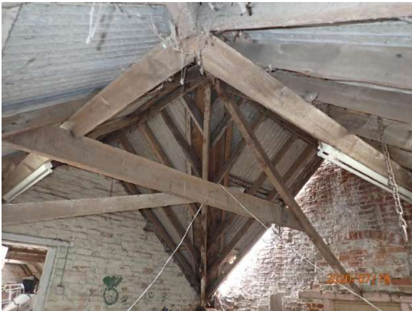
Plate 327: View of the roof supporting structure of Cell 14, from the north-east
