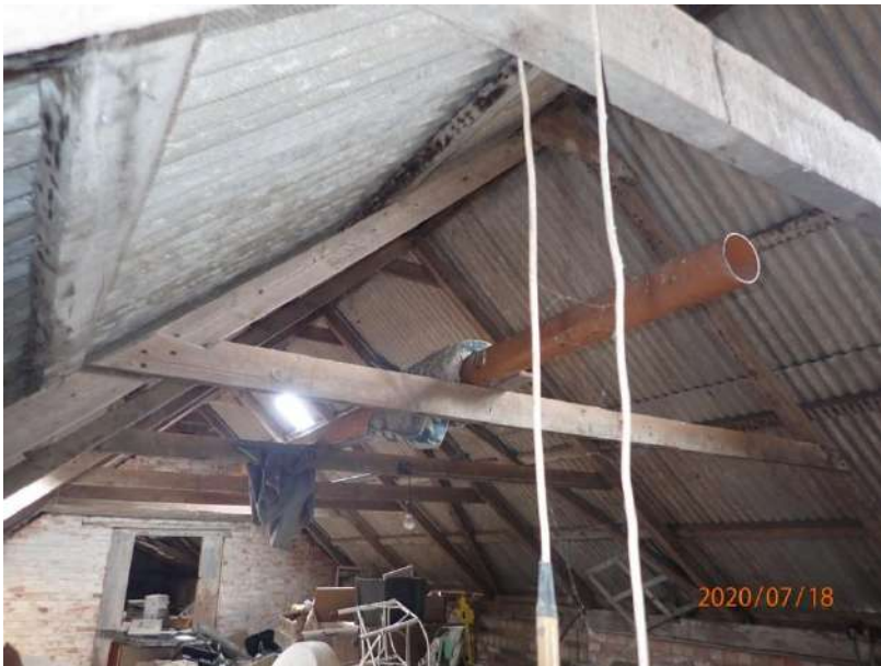
Plate 349: View of the roof supporting structure of Cell 15, from the north
