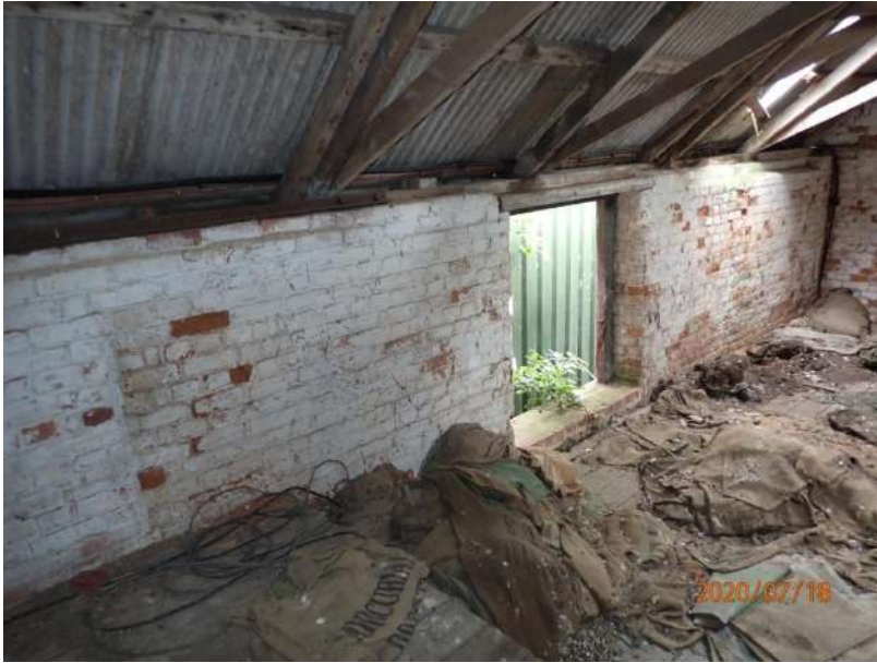
Plate 368: View of the east wall of Cell 17, from the south
