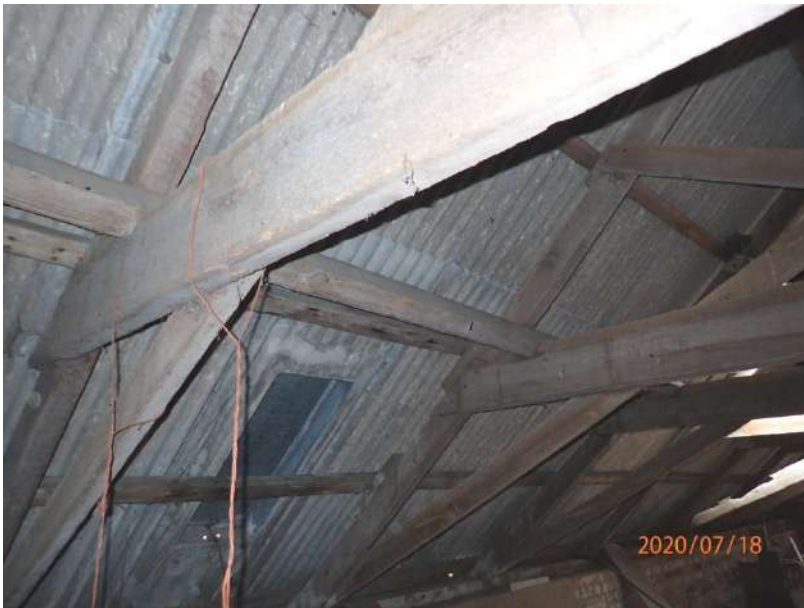
Plate 361: View of the roof supporting structure of Cell 16, from the south
