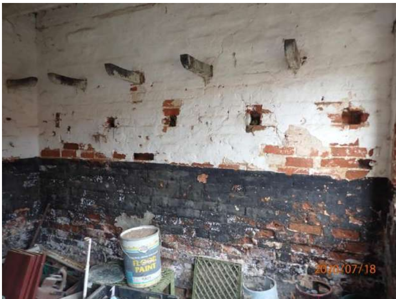
Plate 265: View of the south wall of Cell 11, from the north
