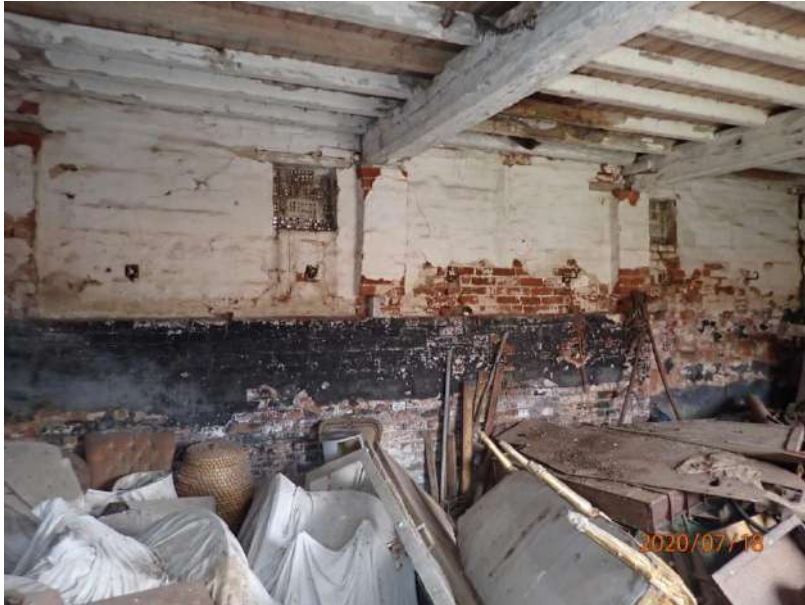
Plate 254: View of the east wall of Cell 10, from the west
