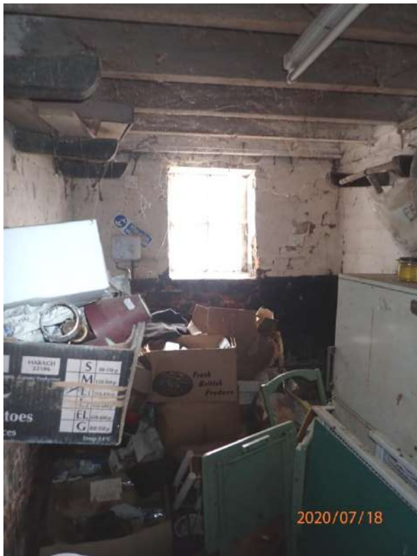
Plate 209: View of the east wall of Cell 7, from the west
