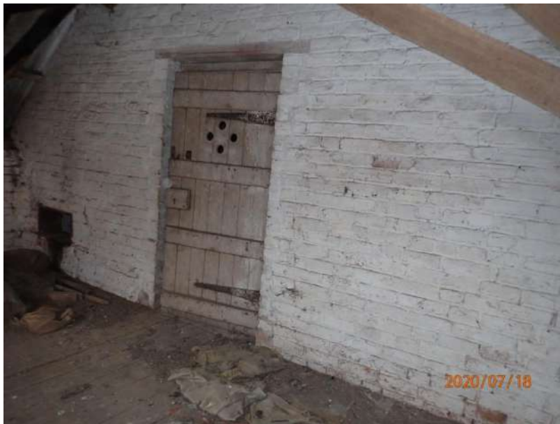
Plate 375: View of the north wall of Cell 17, from the east
