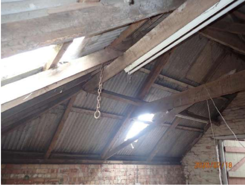
Plate 332: View of the roof supporting structure of Cell 14, from the north-west
