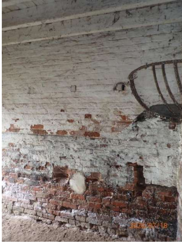
Plate 277: View of the north wall of Cell 12, from the south
