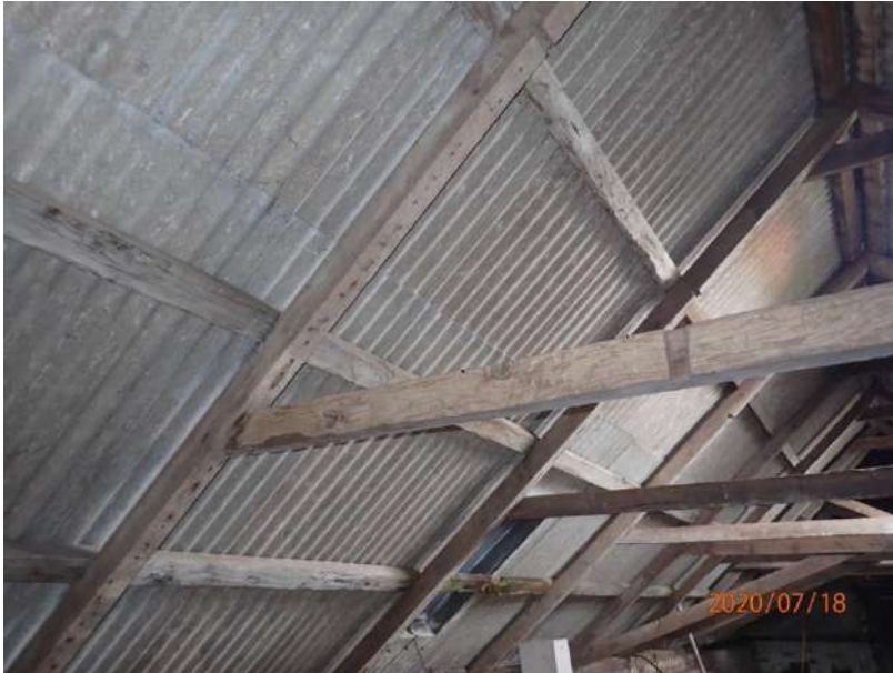
Plate 352: View of the roof supporting structure of Cell 16, from the north
