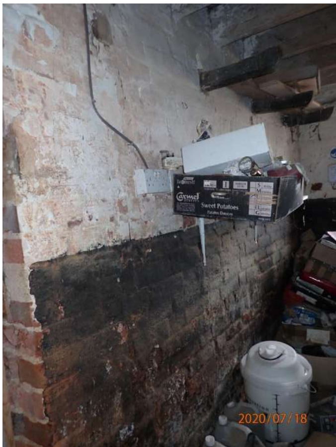
Plate 213: View of the north wall of Cell 7, from the west
