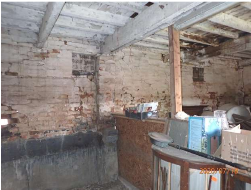
Plate 222: View of the east wall of Cell 8, from the west
