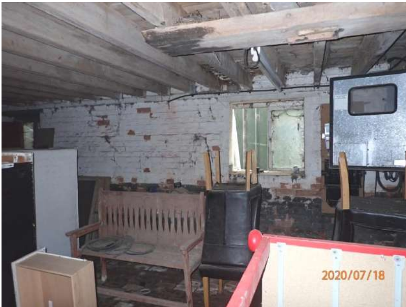
Plate 305: View of the east wall of Cell 13, from the west
