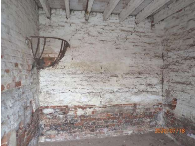
Plate 274: View of the east wall of Cell 12, from the west
