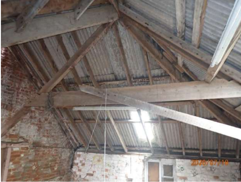
Plate 322: View of the roof supporting structure of Cell 14, from the south
