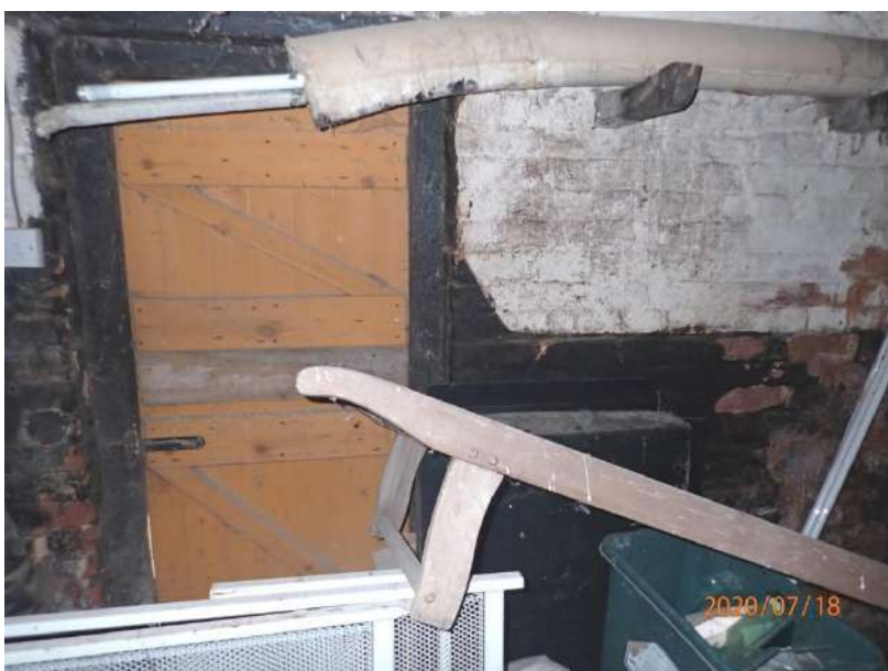
Plate 211: View of the south wall of Cell 7, from the north
