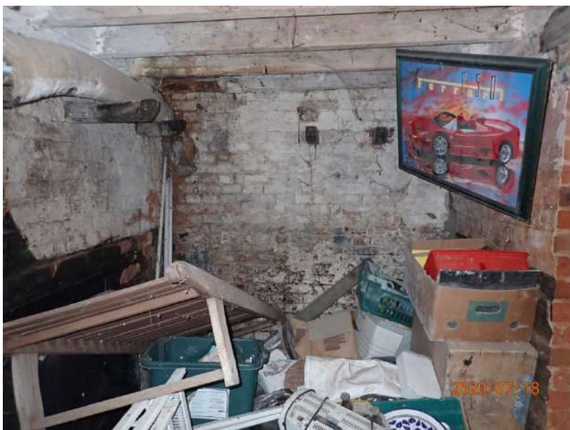
Plate 210: View of the west wall of Cell 7, from the east
