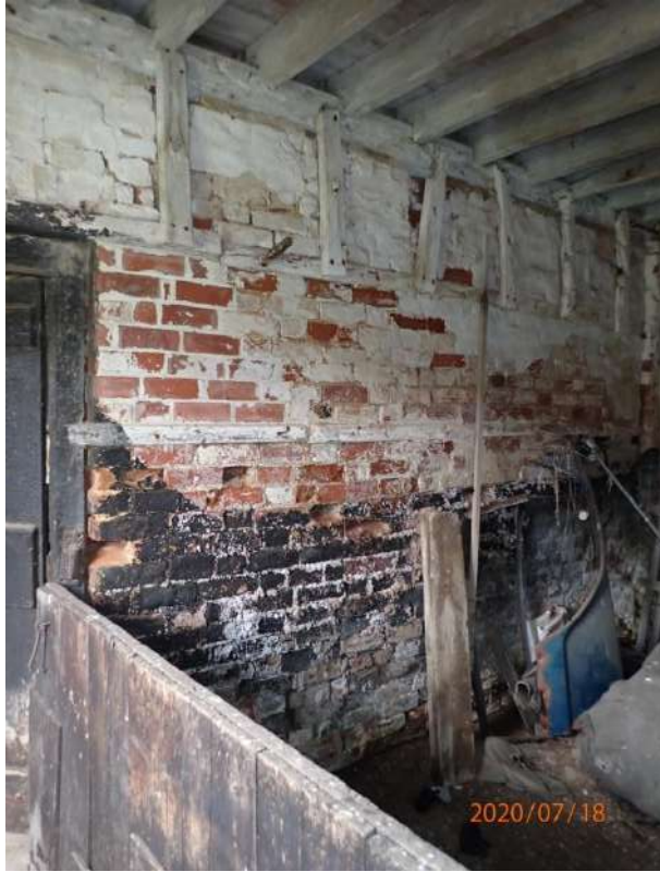
Plate 245: View of the south wall of Cell 9, from the west
