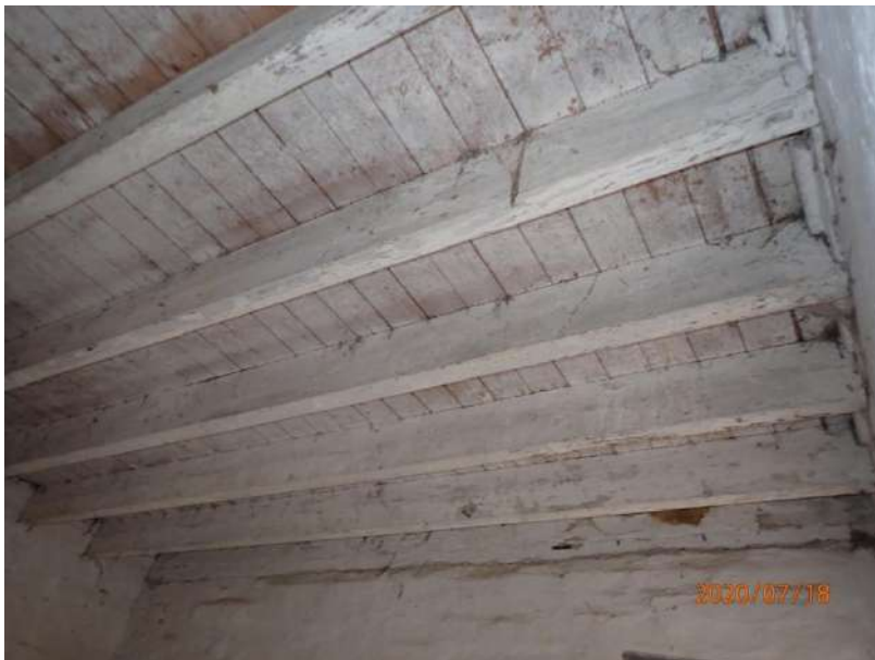
Plate 271: View of the ceiling of Cell 11, from the north
