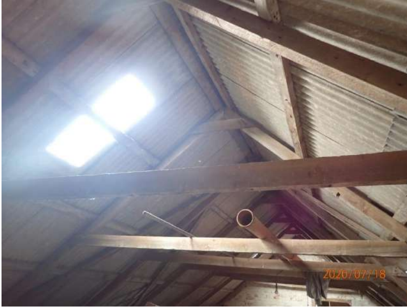
Plate 334: View of the roof supporting structure of Cell 15, from the south
