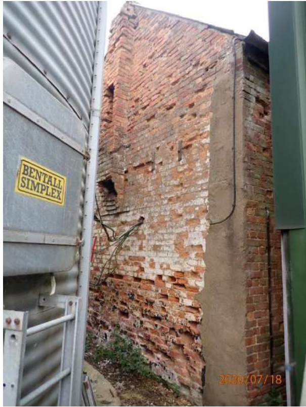
Plate 170: View of the South Elevation of the East Range, from the east
