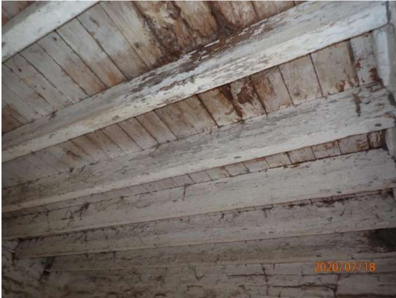
Plate 281: View of the ceiling of Cell 12, from the north
