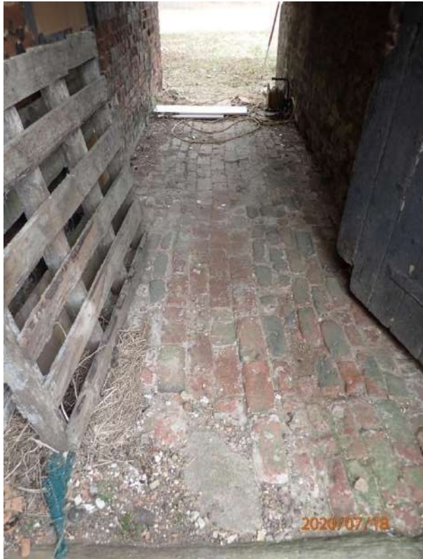
Plate 184: View of the interior of the northern tunnel within the East Range, from the west
