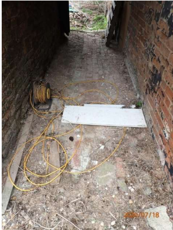
Plate 182: View of the interior of the northern tunnel within the East Range, from the east
