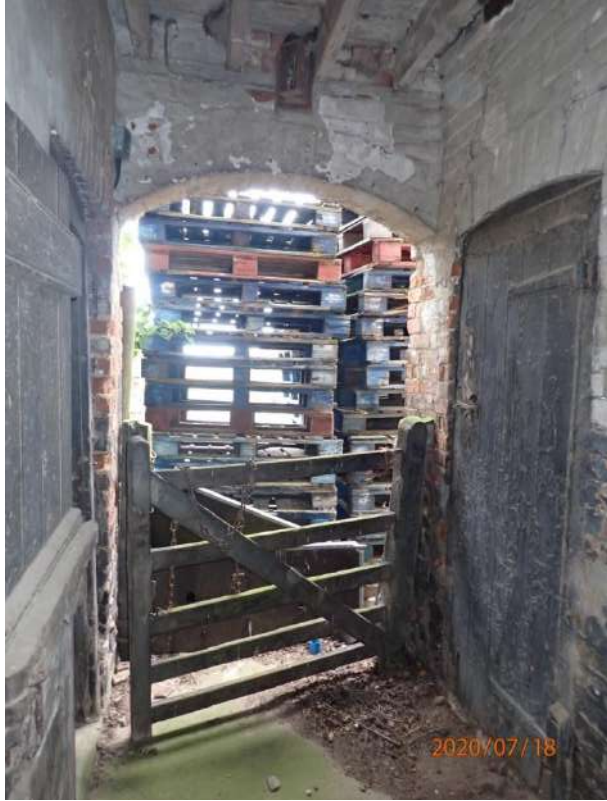
Plate 284: View of the interior of the south tunnel, from the east
