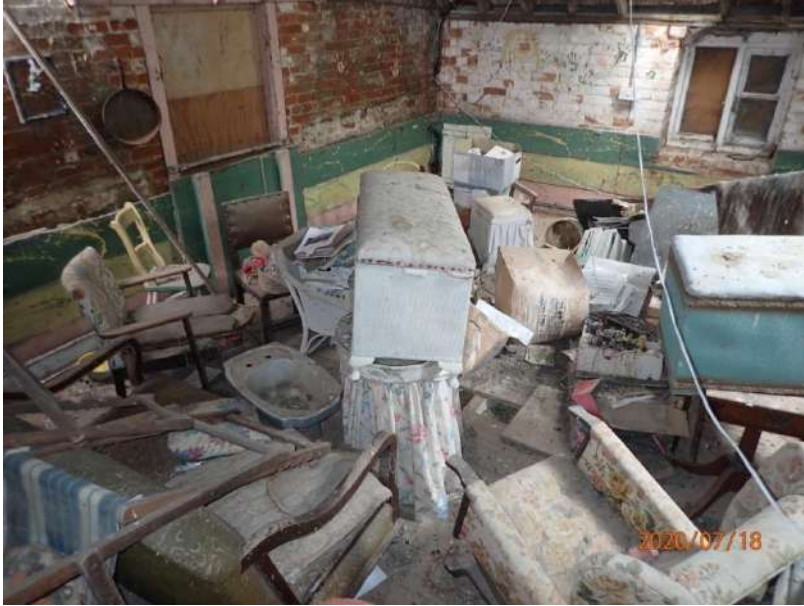
Plate 316: General view of the interior of Cell 14, from the south
