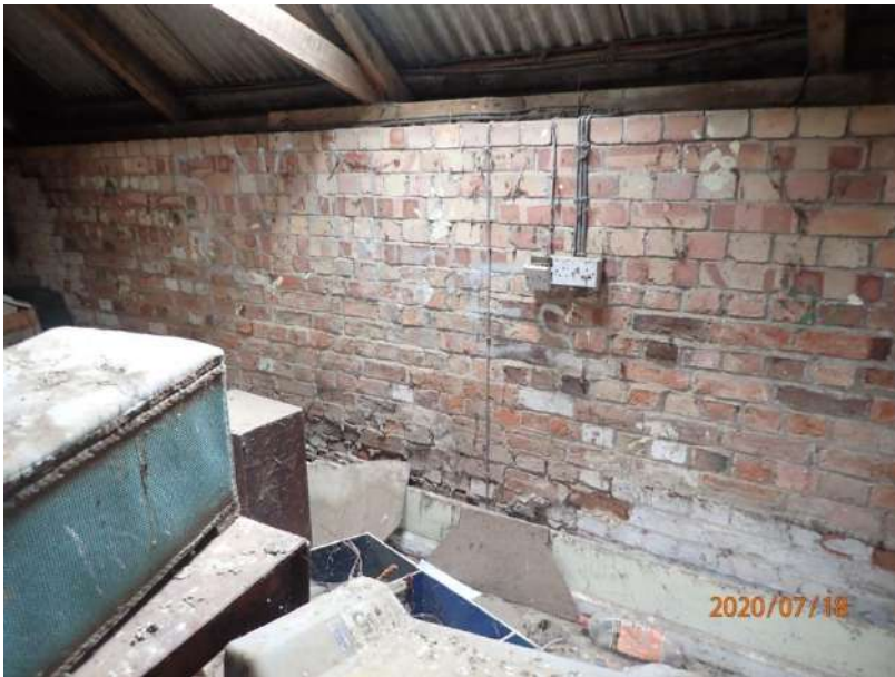
Plate 323: View of the east wall of Cell 14, from the south-west
