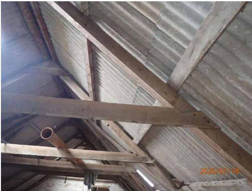
Plate 335: View of the roof supporting structure of Cell 15, from the south
