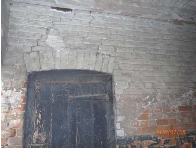
Plate 295: View of the interior of the south tunnel, from the south
