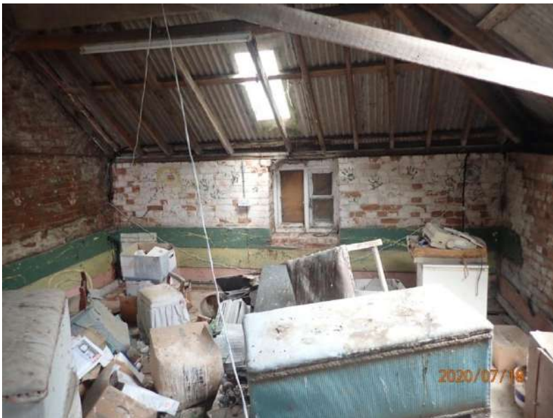
Plate 321: View of the north wall of Cell 14, from the south
