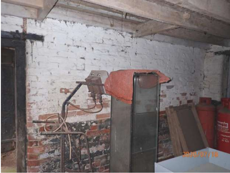
Plate 302: View of the north wall of Cell 13, from the south
