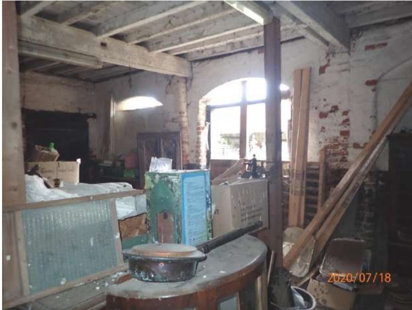
Plate 225: View of the west wall of Cell 8, from the north-east
