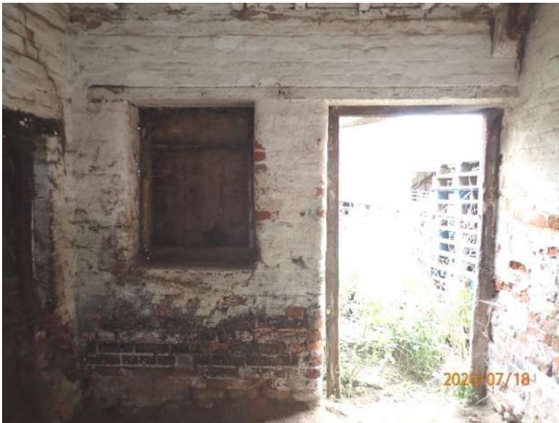
Plate 275: View of the west wall of Cell 12, from the east
