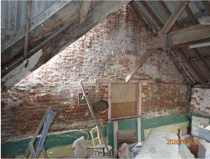
Plate 320: View of the west wall of Cell 14, from the south-east
