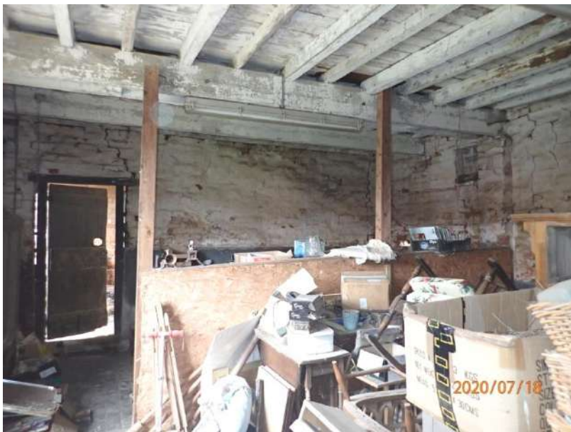
Plate 228: General view of the interior of Cell 8, from the south
