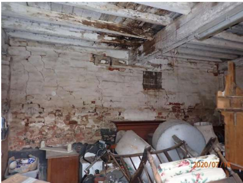
Plate 226: View of the east wall of Cell 8, from the west
