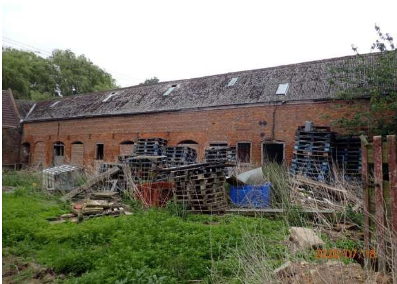
Plate 192: General view of the West Elevation of the East Range, from the west
