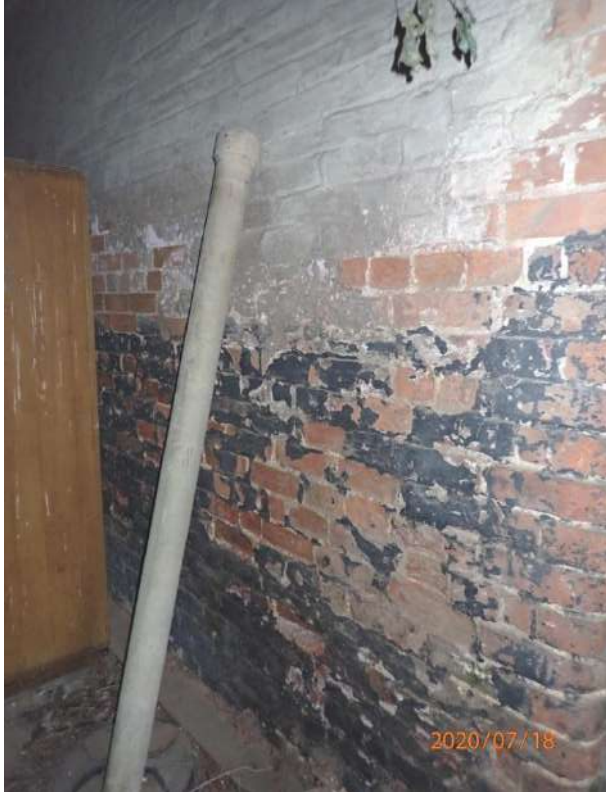
Plate 297: View of the interior of the south tunnel, from the east
