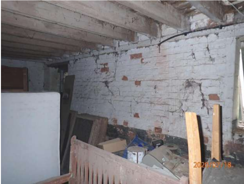
Plate 308: View of the east wall of Cell 13, from the south
