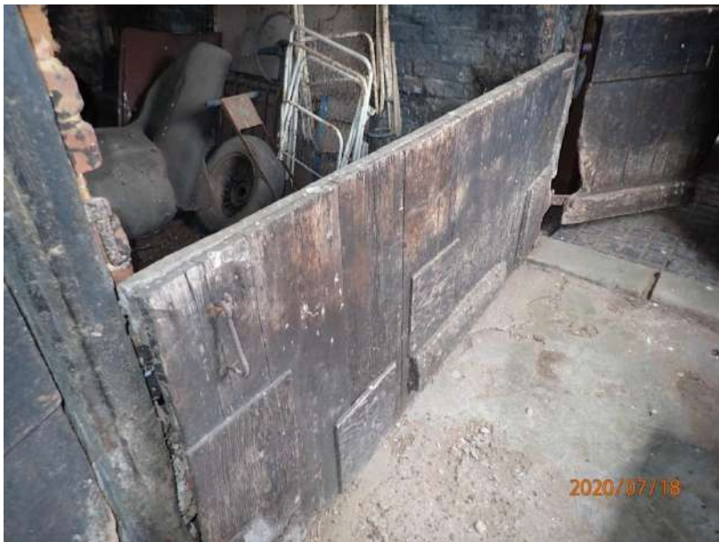
Plate 246: View of the low timber partition, from the north
