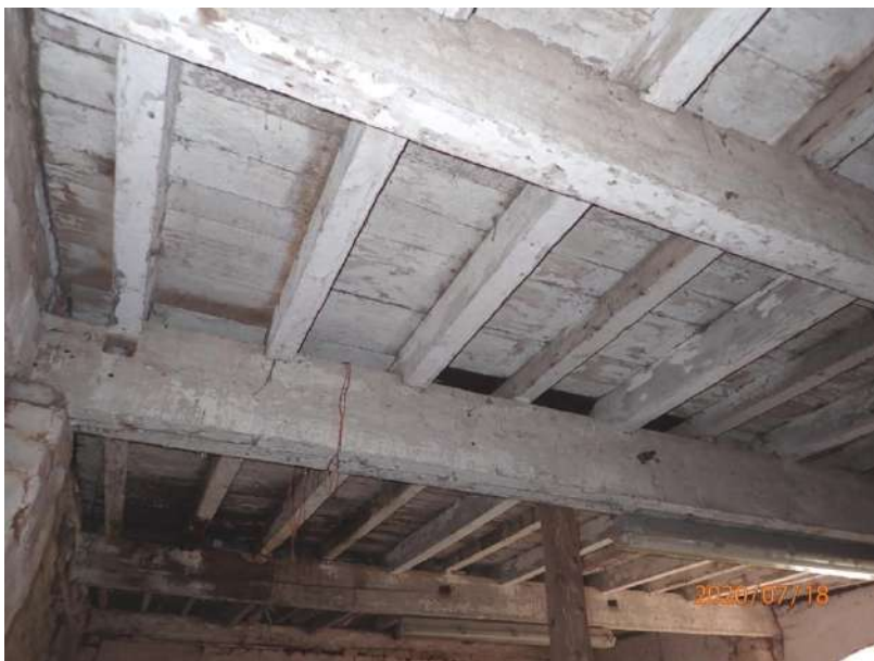
Plate 235: View of the ceiling of Cell 8, from the south
