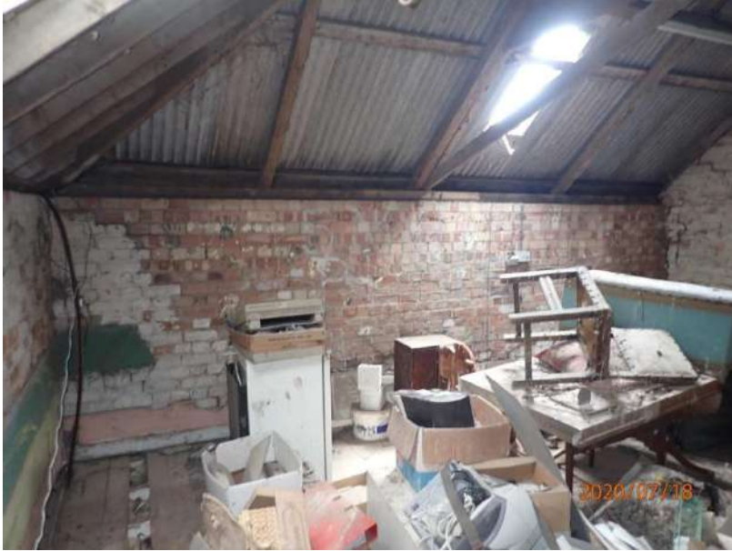
Plate 330: View of the east wall of Cell 14, from the west
