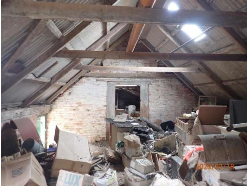
Plate 346: View of the south wall of Cell 15, from the north
