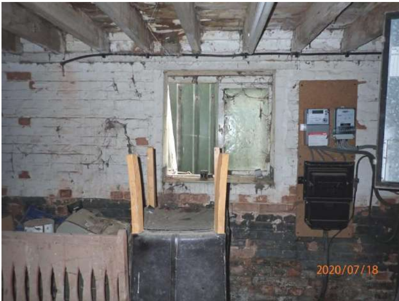
Plate 307: View of the east wall of Cell 13, from the west
