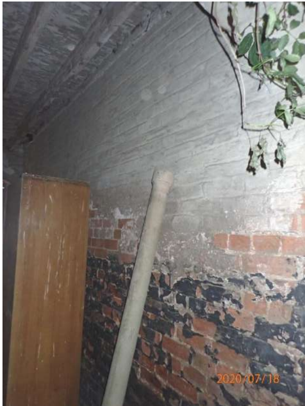
Plate 298: View of the interior of the south tunnel, from the east
