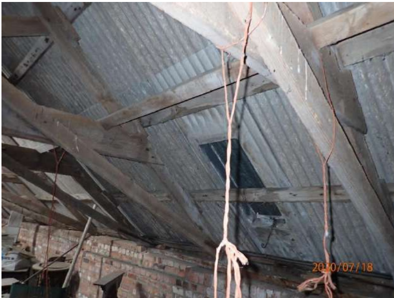
Plate 363: View of the roof supporting structure of Cell 16, from the south
