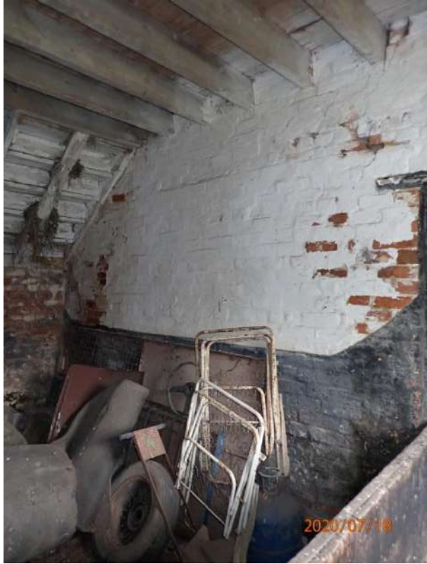
Plate 243: View of the south wall of Cell 9, from the north
