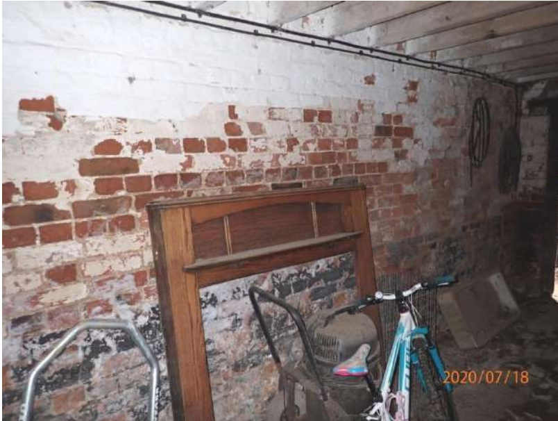
Plate 310: View of the west wall of Cell 13, from the east
