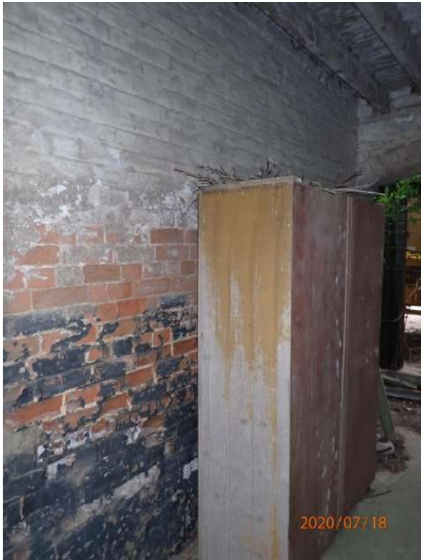
Plate 296: View of the interior of the south tunnel, from the west
