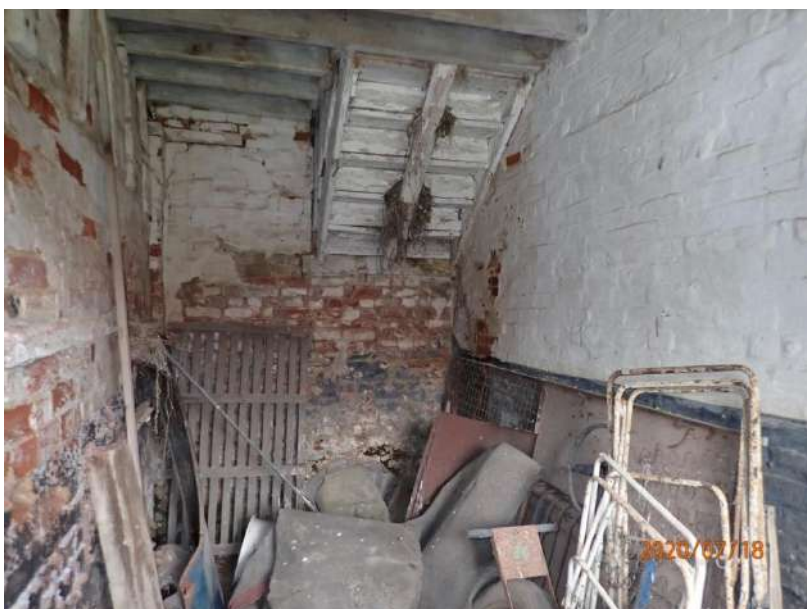
Plate 239: View of the east wall of Cell 9, from the west
