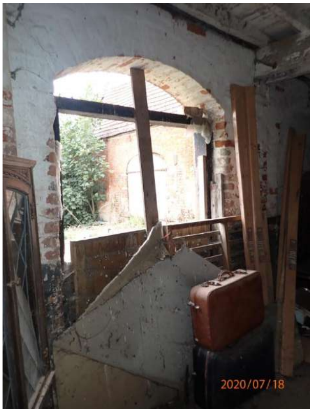
Plate 231: View of the west wall of Cell 8, from the east
