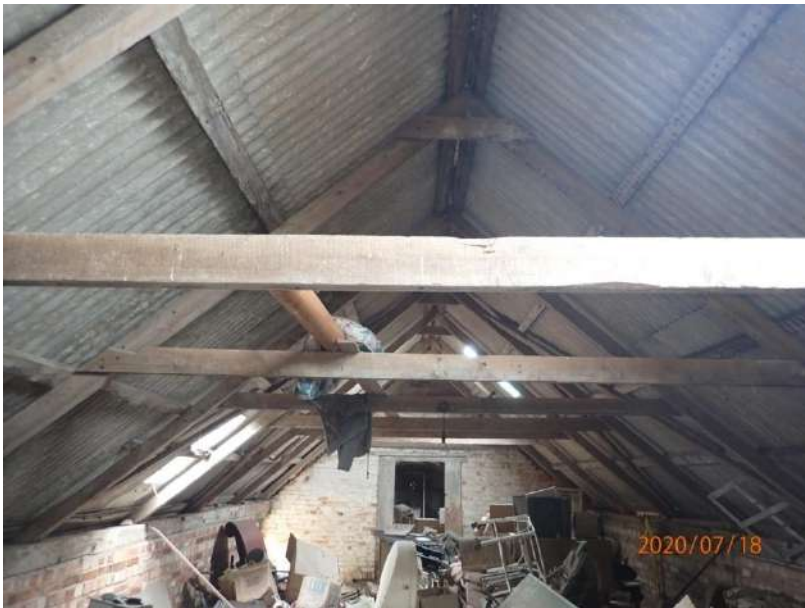
Plate 343: View of the roof supporting structure of Cell 15, from the north
