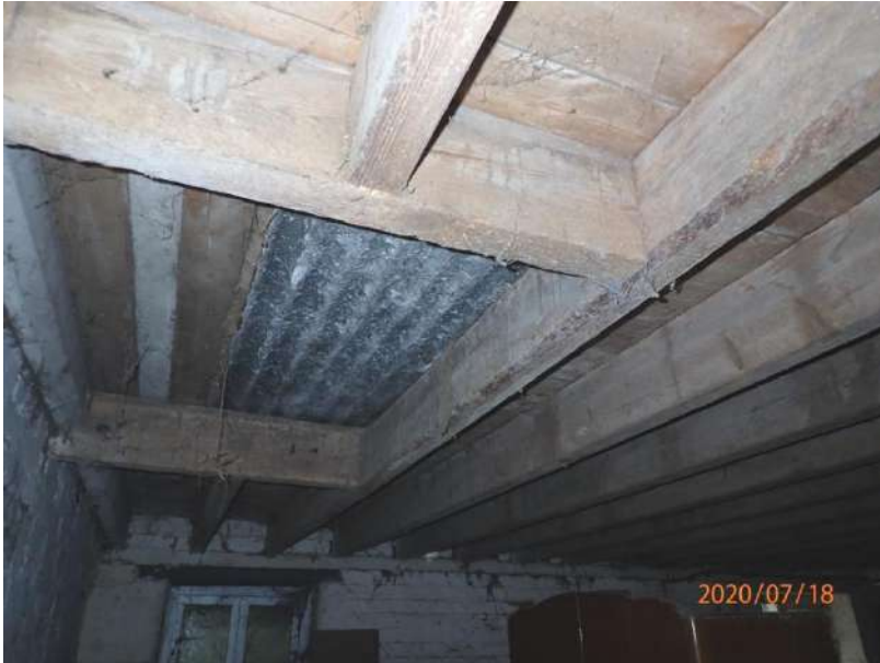
Plate 314: View of the ceiling structure of Cell 13, from the west
