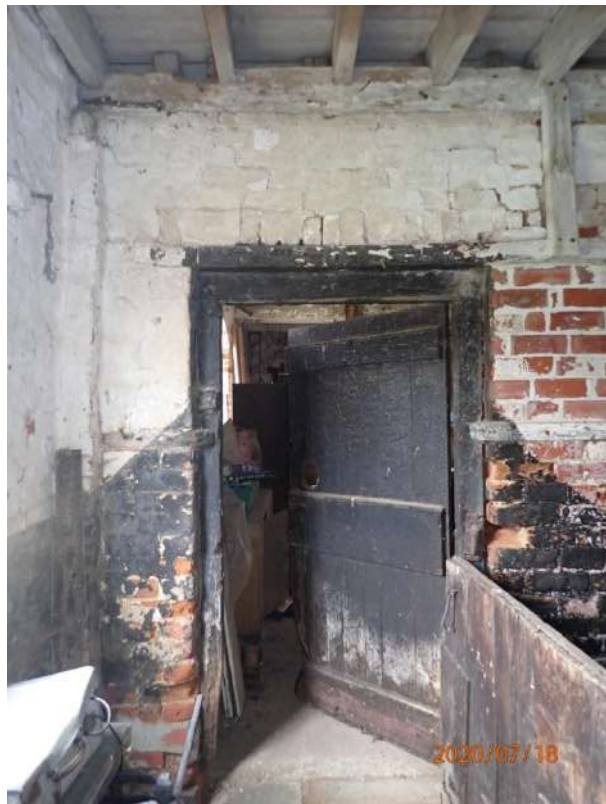
Plate 244: View of the south wall of Cell 9, from the north
