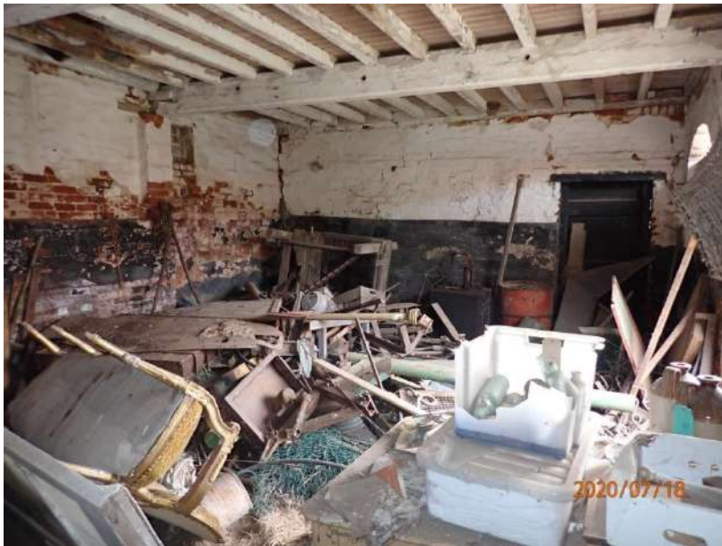
Plate 252: General view of the interior of Cell 10, from the north
