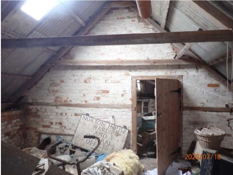
Plate 340: View of the north wall of Cell 15, from the south
