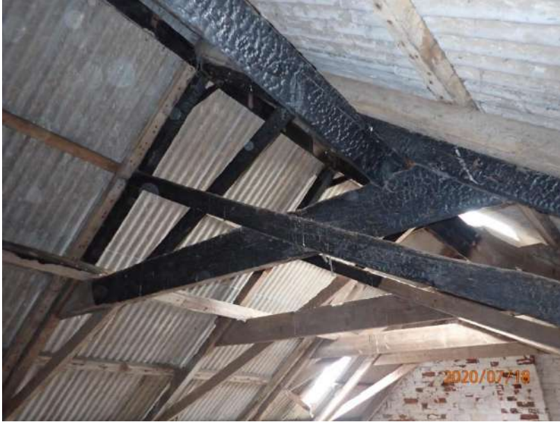
Plate 382: View of the roof supporting structure of Cell 17, from the north
