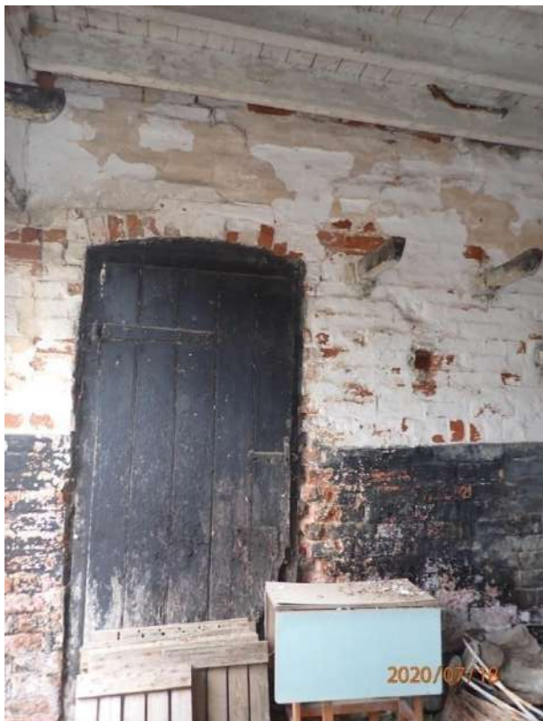
Plate 267: View of the north wall of Cell 11, from the south
