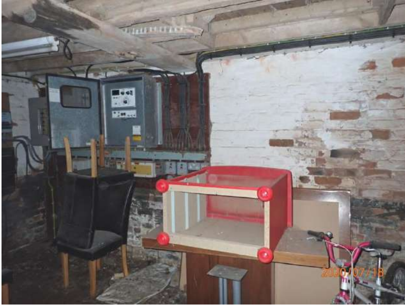
Plate 304: View of the south wall of Cell 13, from the north
