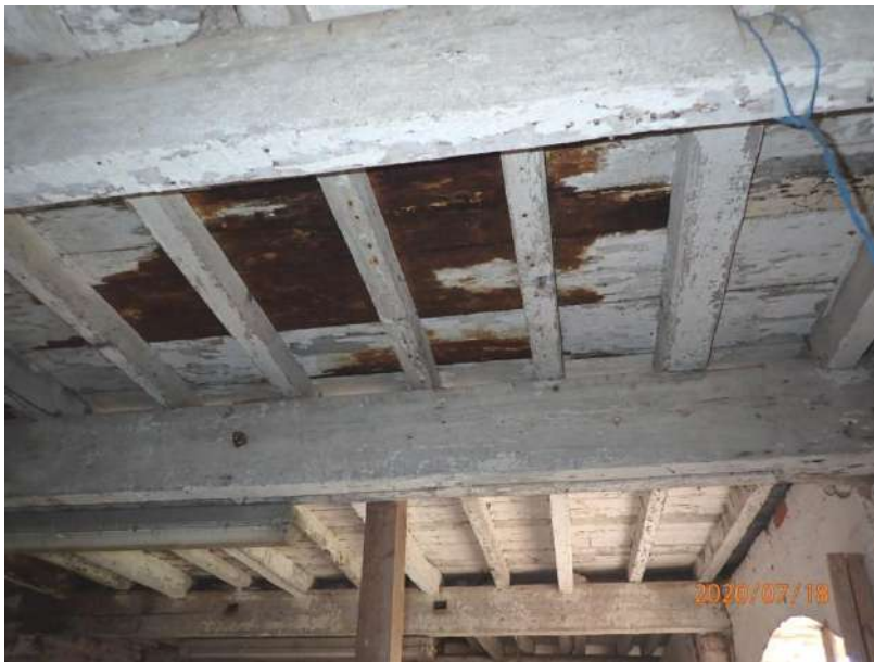
Plate 233: View of the ceiling of Cell 8, from the north
