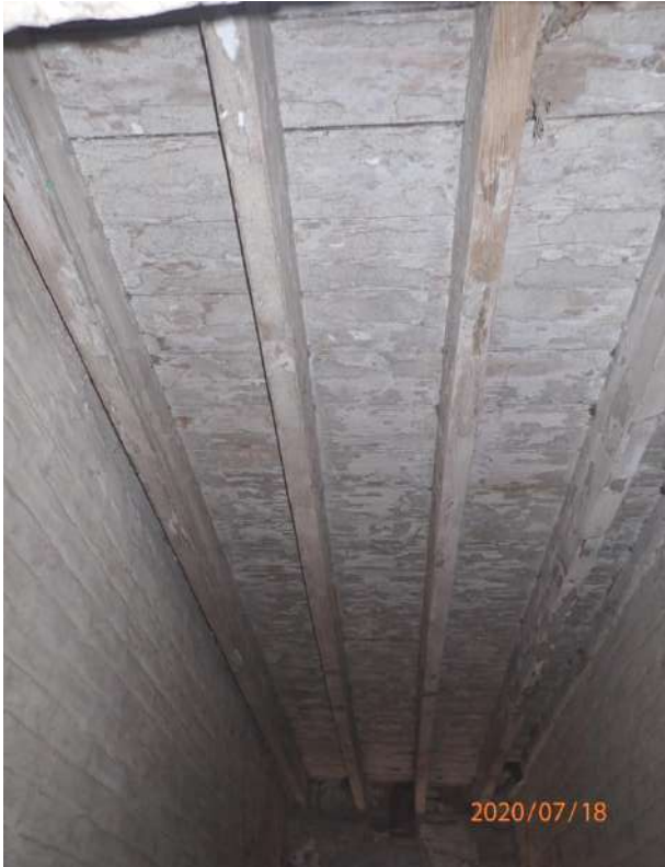
Plate 289: View of the interior of the south tunnel, from the east
