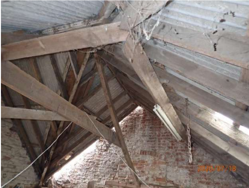
Plate 328: View of the roof supporting structure of Cell 14, from the east
