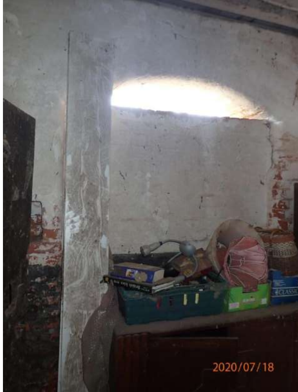
Plate 230: View of the west wall of Cell 8, from the east
