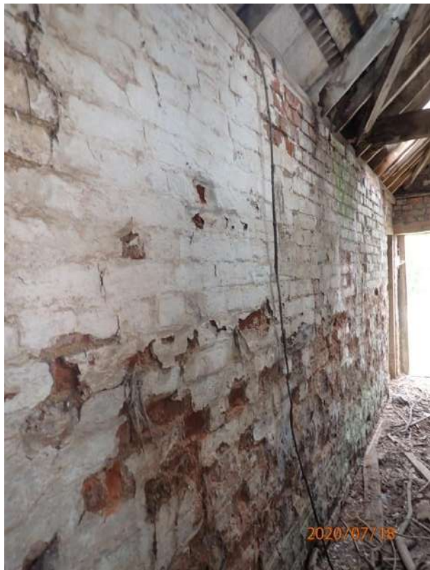
Plate 410: View of the interior of Cell 18, from the east
