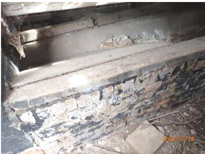
Plate 403: View of the interior of Cell 18, from the south
