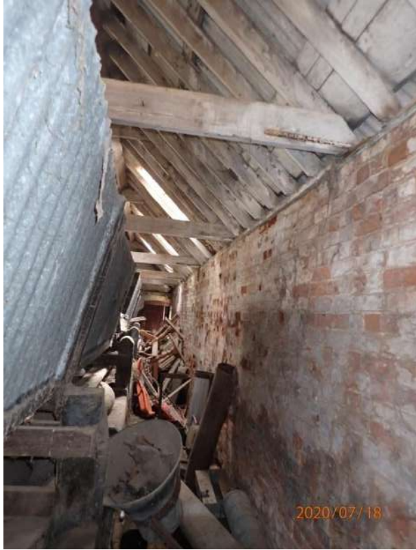
Plate 409: View of the interior of Cell 18, from the west
