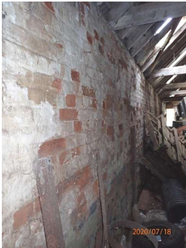
Plate 412: View of the interior of Cell 18, from the east
