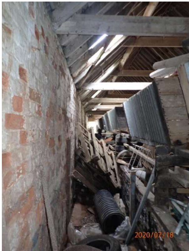
Plate 414: View of the interior of Cell 18, from the east
