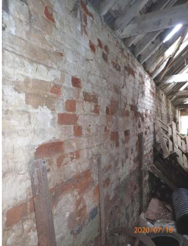
Plate 415: View of the interior of Cell 18, from the east
