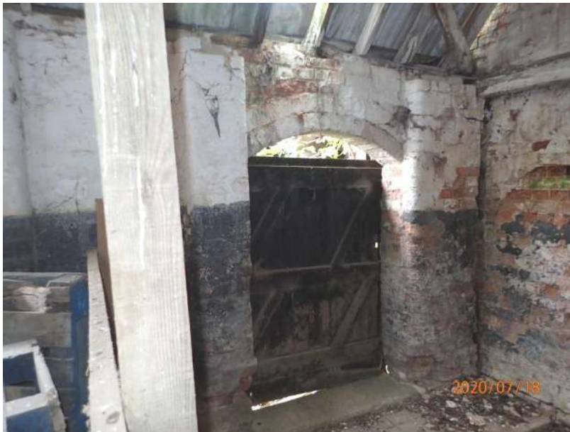
Plate 477: View of the interior of the South Range, from the south-west
