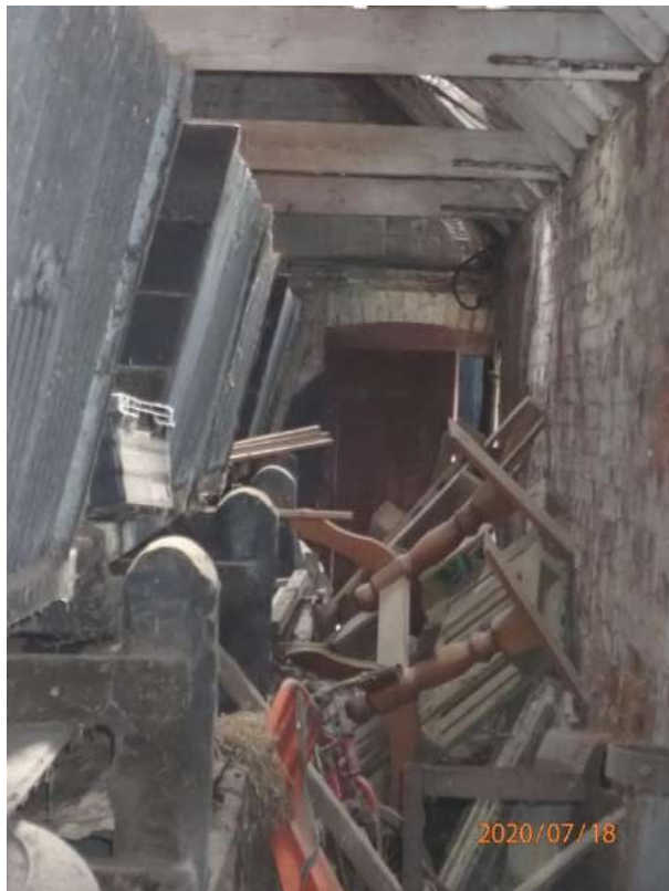
Plate 408: View of the interior of Cell 18, from the west
