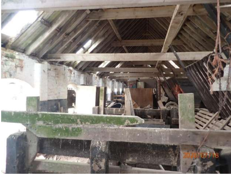
Plate 453: View of the interior of the South Range, from the west
