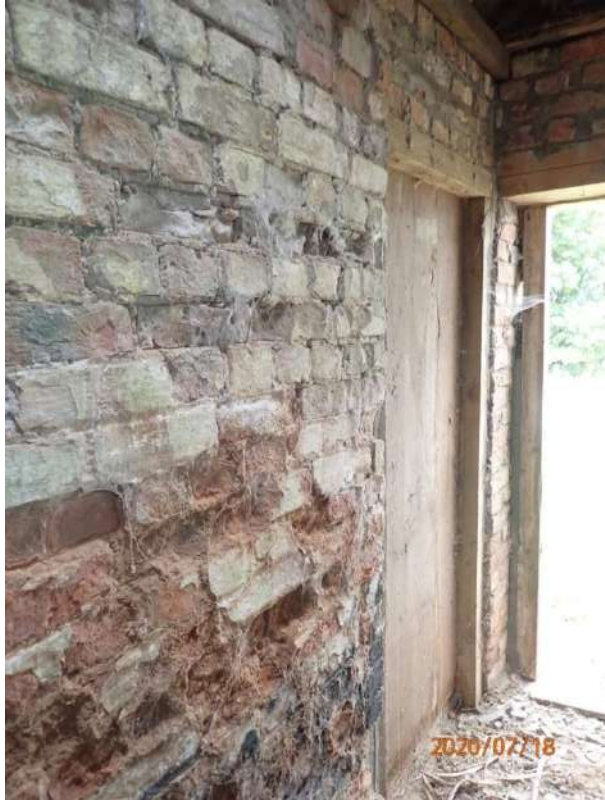
Plate 411: View of the interior of Cell 18, from the east
