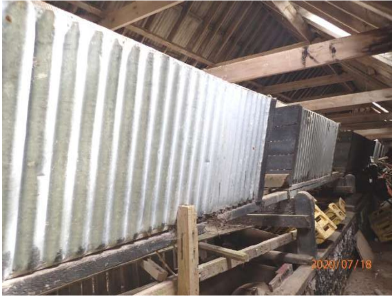
Plate 405: View of the interior of Cell 18, from the west
