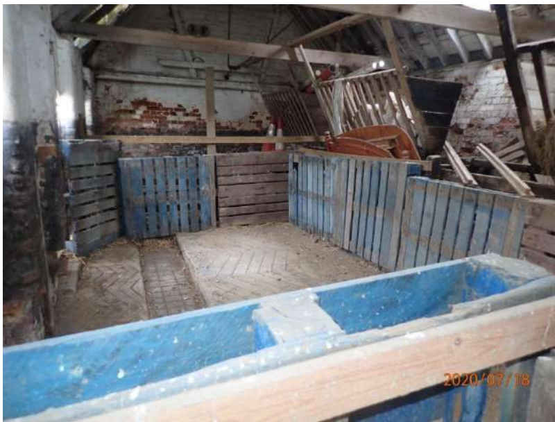
Plate 468: View of the interior of the South Range, from the west
