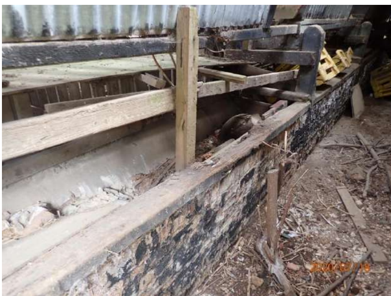
Plate 404: View of the interior of Cell 18, from the west
