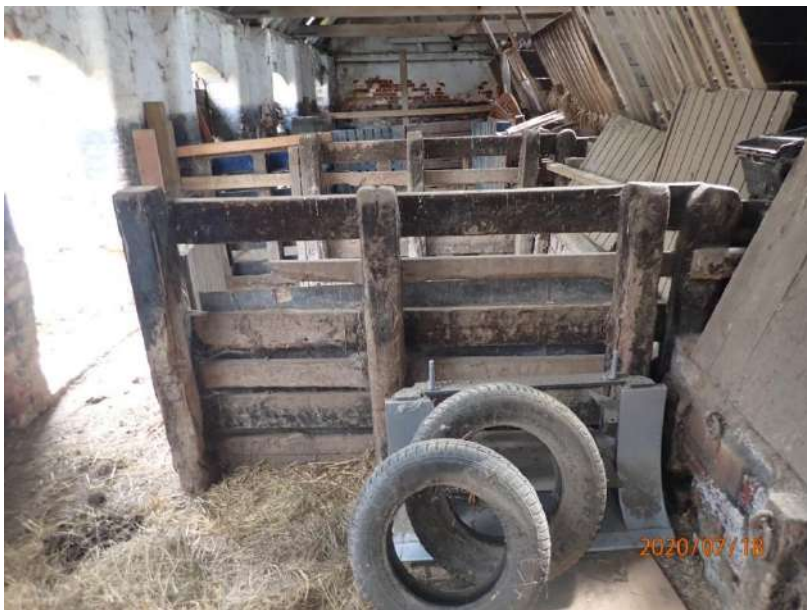
Plate 460: View of the interior of the South Range, from the west
