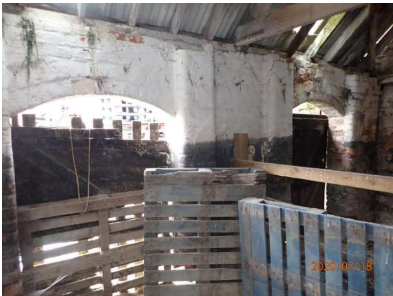
Plate 476: View of the interior of the South Range, from the south-west
