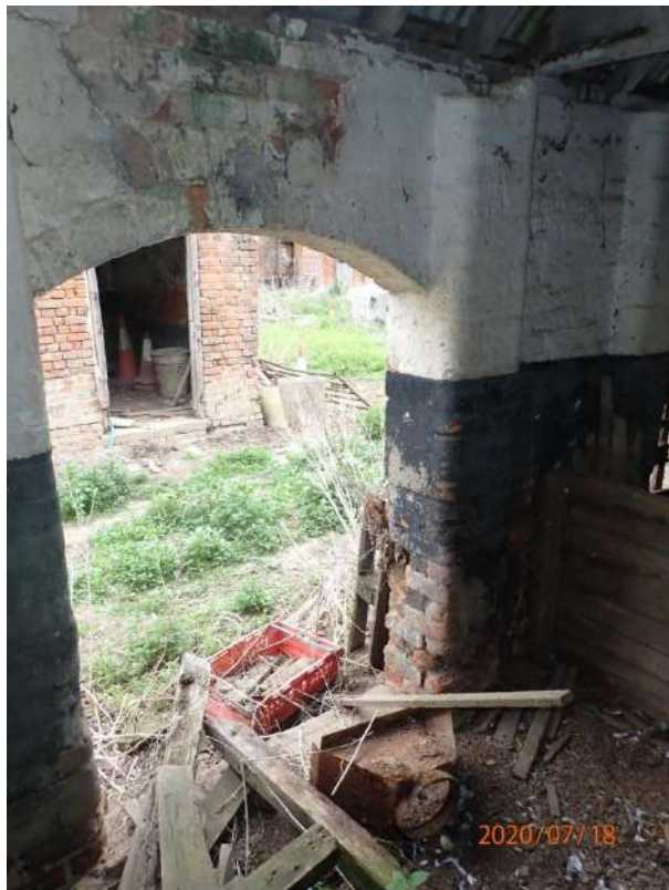
Plate 450: View of the interior of the South Range, from the south-west
