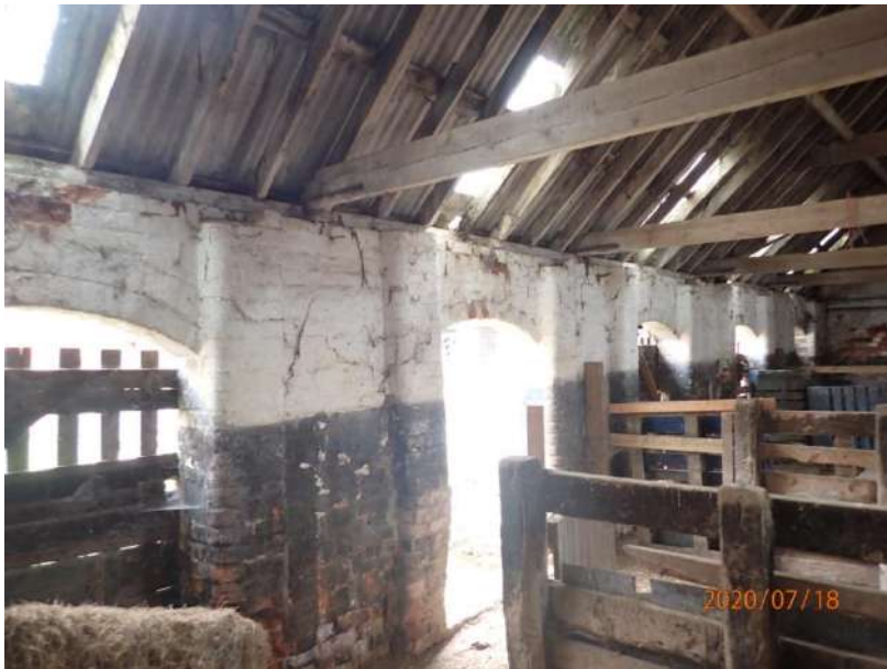
Plate 463: View of the interior of the South Range, from the south-west
