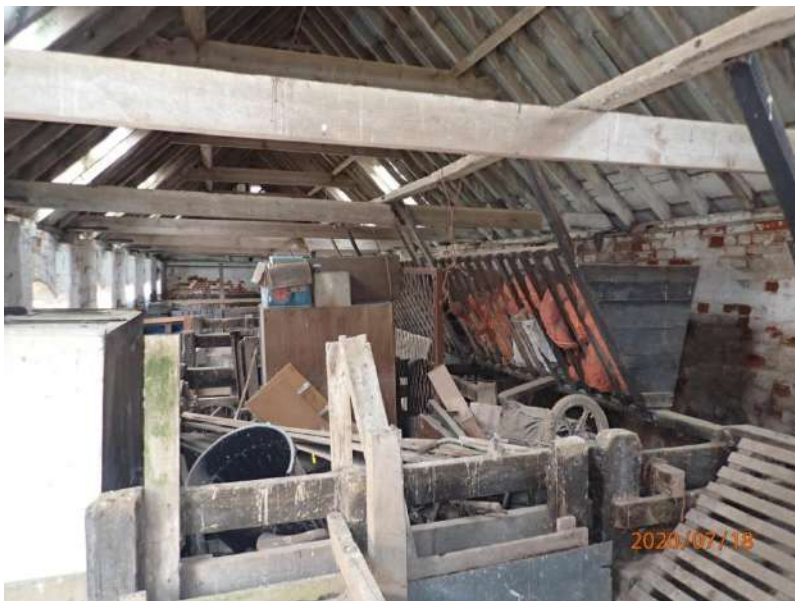
Plate 448: View of the interior of the South Range, from the west
