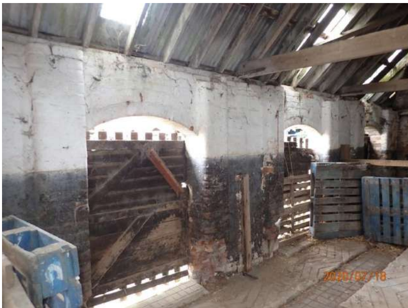
Plate 470: View of the interior of the South Range, from the south-west
