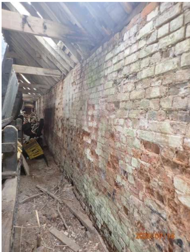
Plate 406: View of the interior of Cell 18, from the west
