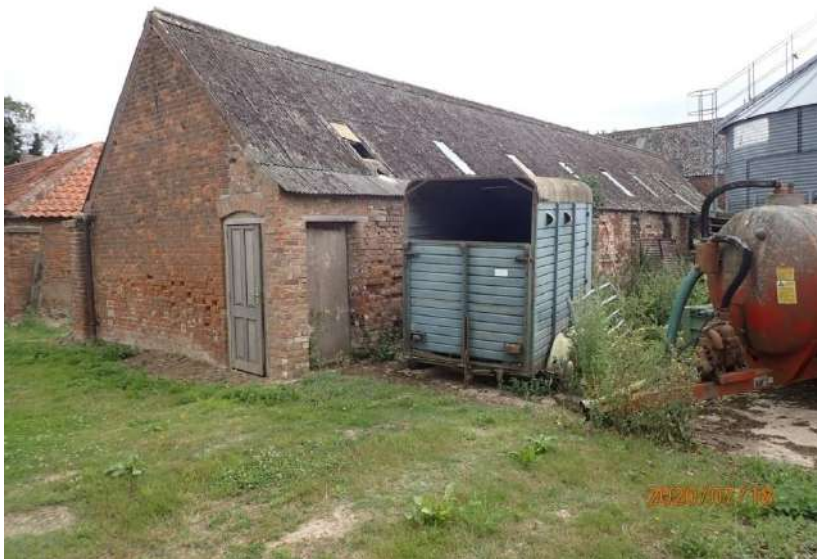
Plate 386: General view of the South Range, from the south-west
