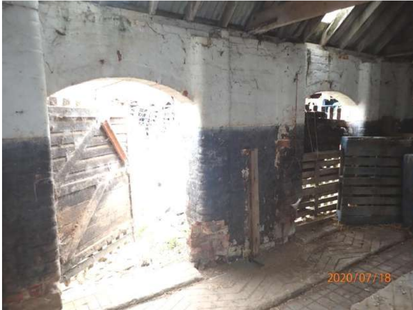
Plate 475: View of the interior of the South Range, from the south-west
