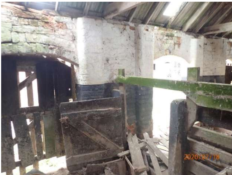
Plate 452: View of the interior of the South Range, from the south-west
