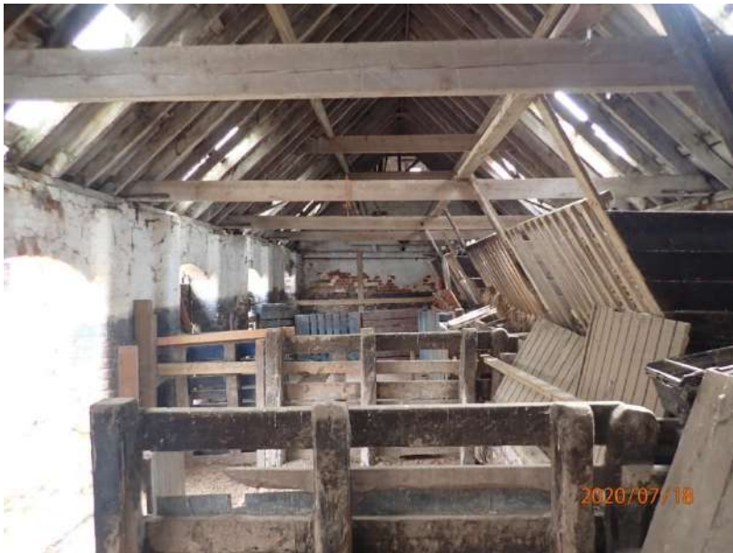
Plate 461: View of the interior of the South Range, from the west
