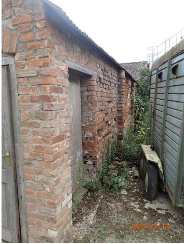
Plate 384: View of the South Elevation of the South Range, from the west
