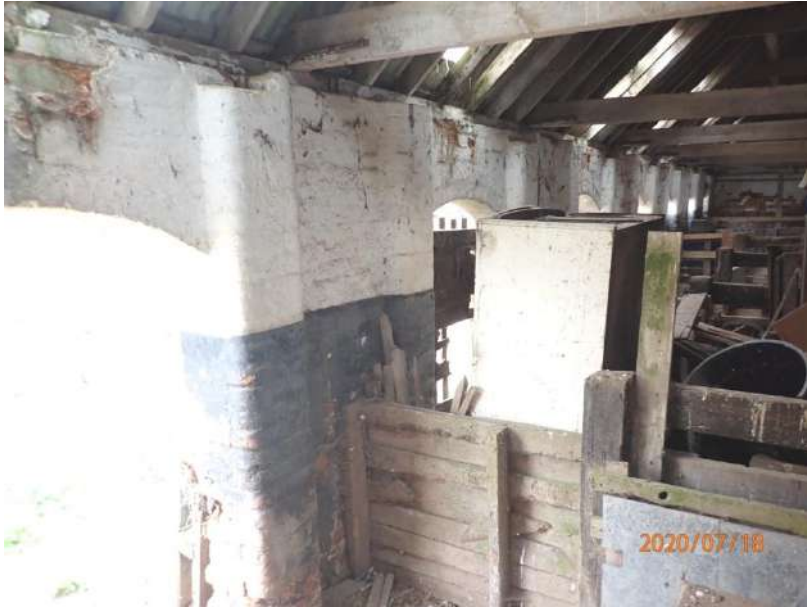
Plate 449: View of the interior of the South Range, from the west
