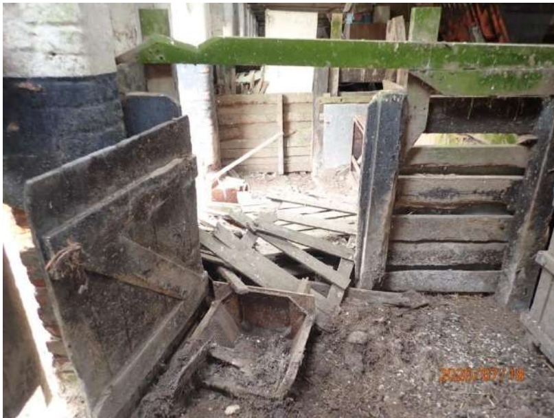
Plate 454: View of the interior of the South Range, from the west
