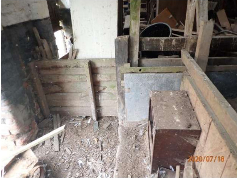
Plate 447: View of the interior of the South Range, from the west
