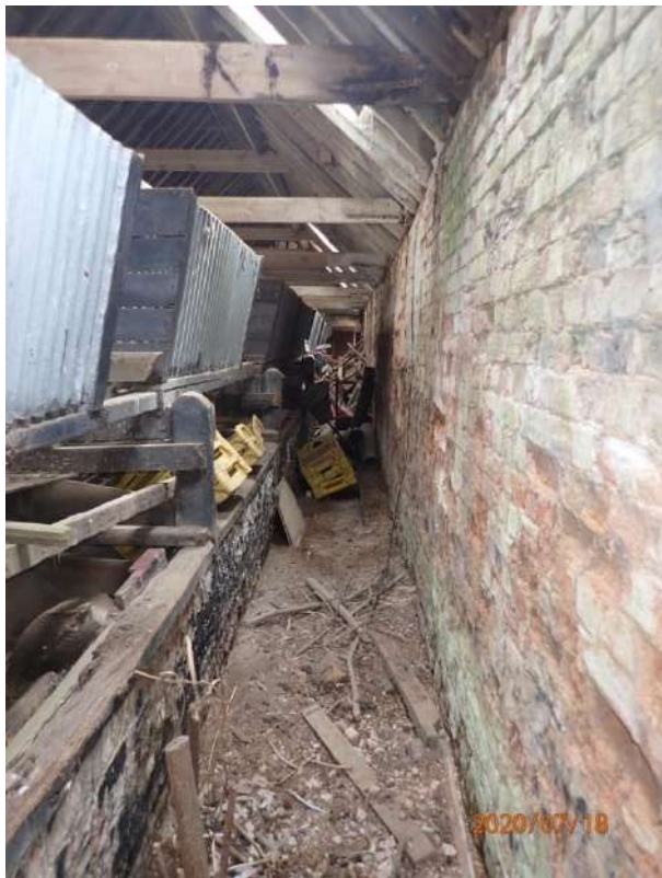
Plate 402: General view of the interior of Cell 18, from the west
