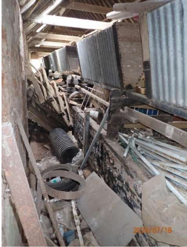
Plate 413: View of the interior of Cell 18, from the east
