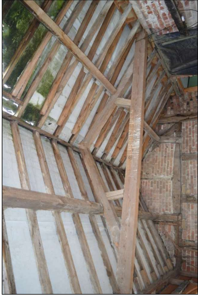
Fig. 43: Central truss of the former byre (CPAT 4900-0037)
