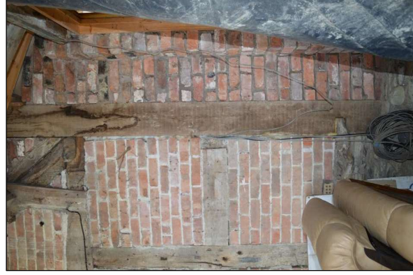
Fig. 38: The timber frame at the north end of the house (CPAT 4900-0032)
