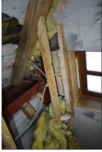
Fig. 54: Steel beam attached to apex of timber frame in bedroom 1 (CPAT 4900-0048)
