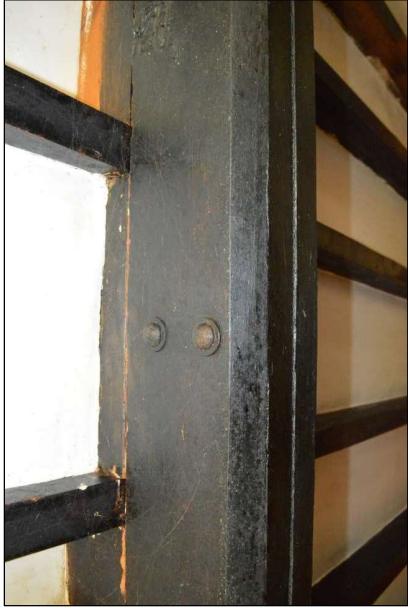
Fig. 31: The bolts in the main kitchen beam (CPAT 4900-0025)
