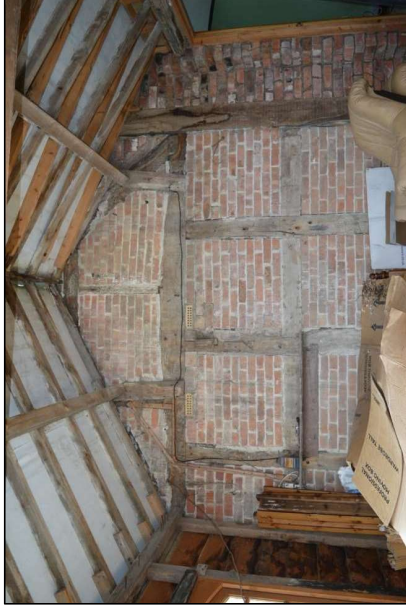
Fig. 38: The timber frame at the north end of the house (CPAT 4900-0032)
