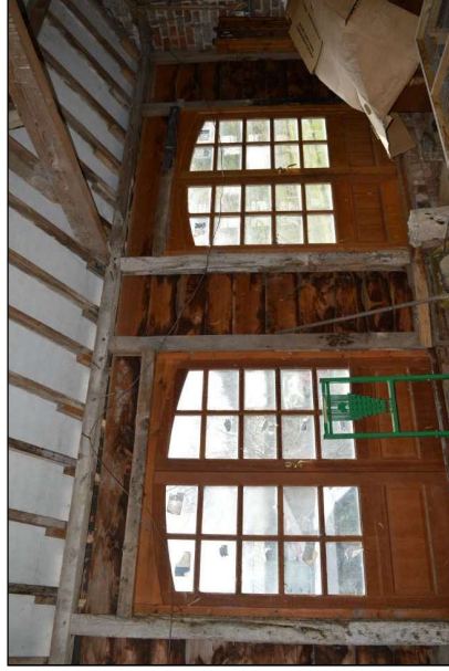
Fig. 47: East wall of former byre with modern doors (CPAT 4900-0041)
