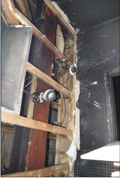
Fig. 51: Steel beam above the bathroom (CPAT 4900-0045)
