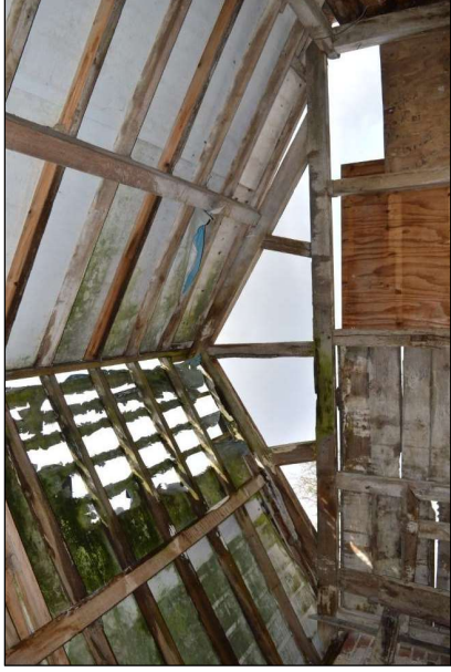
Fig. 44: Northern truss of the former byre (CPAT 4900-0038)
