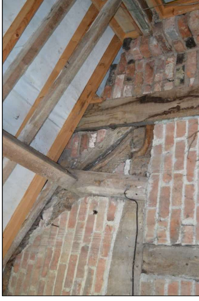
Fig. 39: West end of the frame showing the original roof pitch (CPAT 4900-0033)
