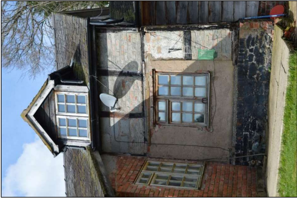
Fig. 25: Timber frame, note the upper panels are later (CPAT 4900-0019)
