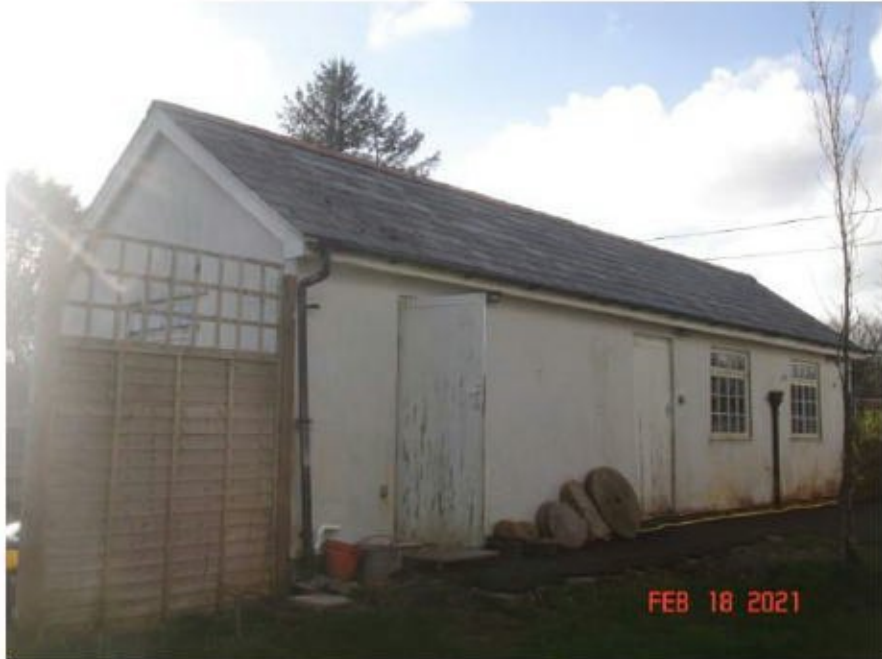
Photograph 1 – View of the northeast and south east aspect.
