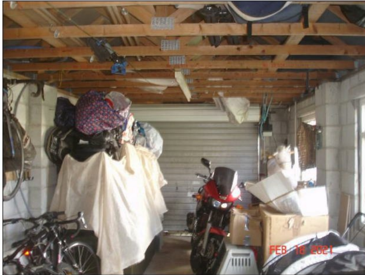
Photograph 2– Internal view of the garage structure.
