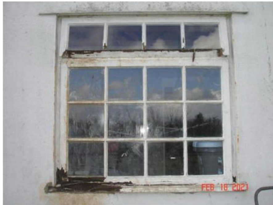
Photograph 4 – View of the window on the southeast aspect.
