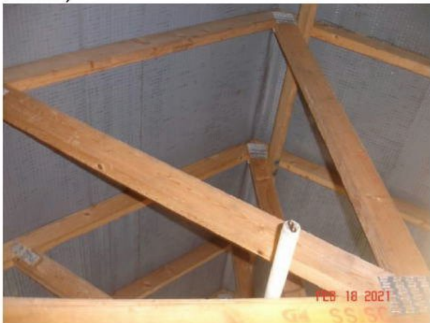
Photograph 5 – Internal view of the roof structure.
