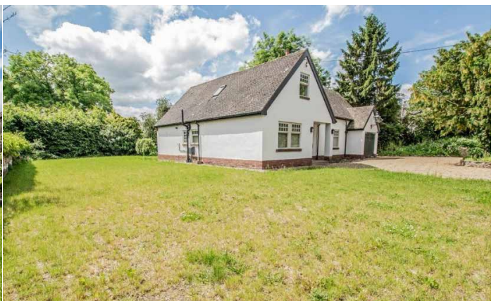
Looking North West
