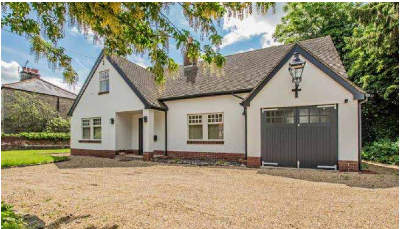
Looking North East
