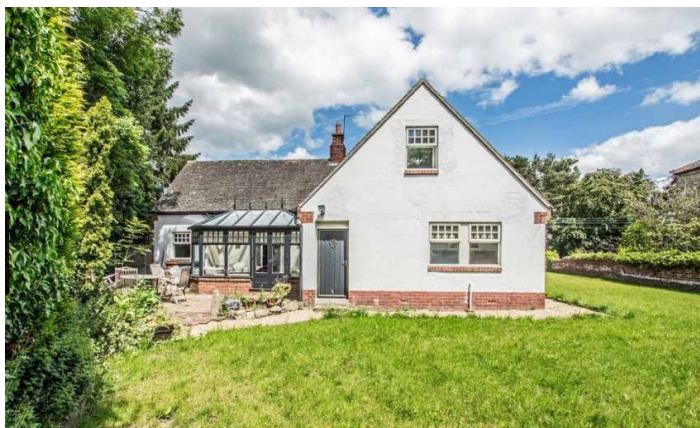
Looking North East
