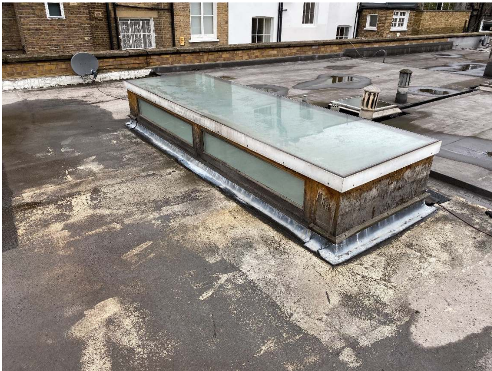
8 2A Montagu Mews South Existing Rooflight – To Be Replaced
