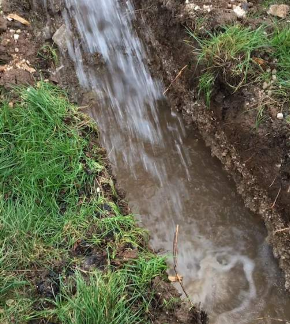
The above photo shows the test hole being filled.
