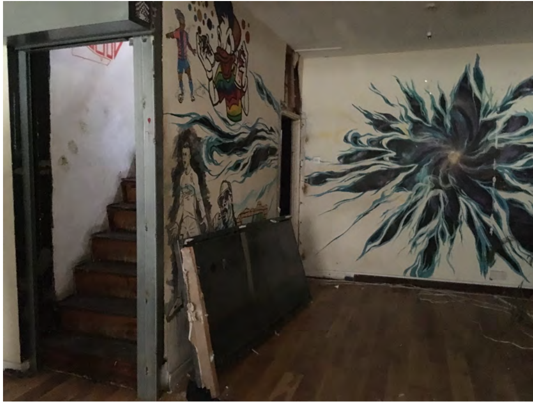
Stairs and rear section
