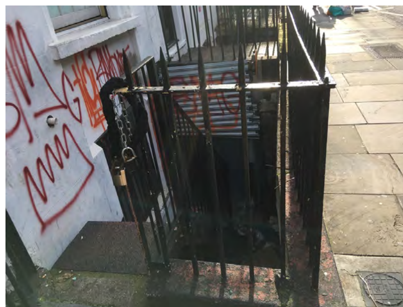
Access to the basement via metal stairs
