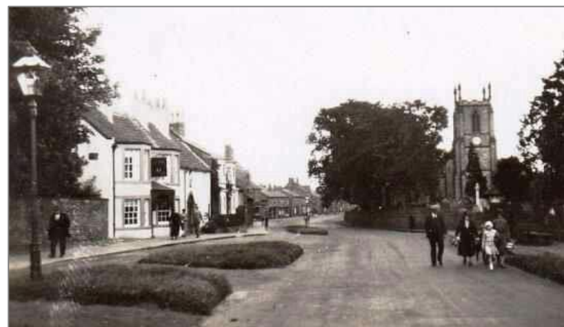
Figure 4 Historic photograph looking east
