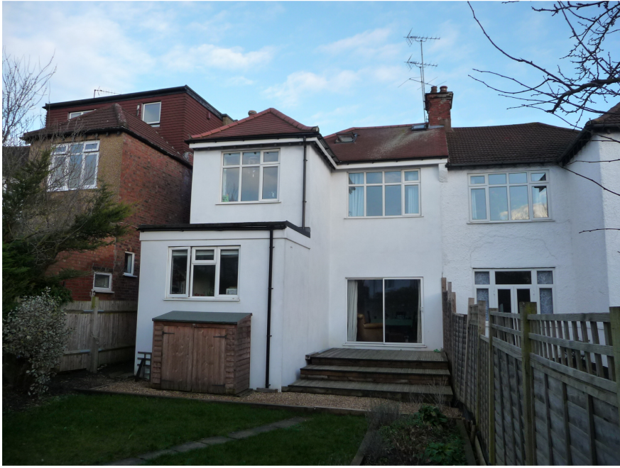
View of rear elevation
