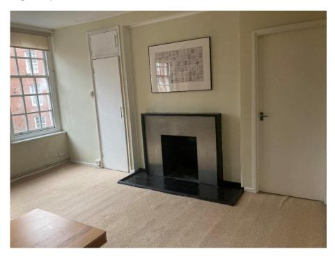
It is proposed to remove the fireplace surround and hearth, and to block off the chamber. The fireplace surround is mounted on a wall which is slightly inset from the walls either side. The proposal is to build out the wall using studwork, covered in plaster board, so that the entire wall is flush.
