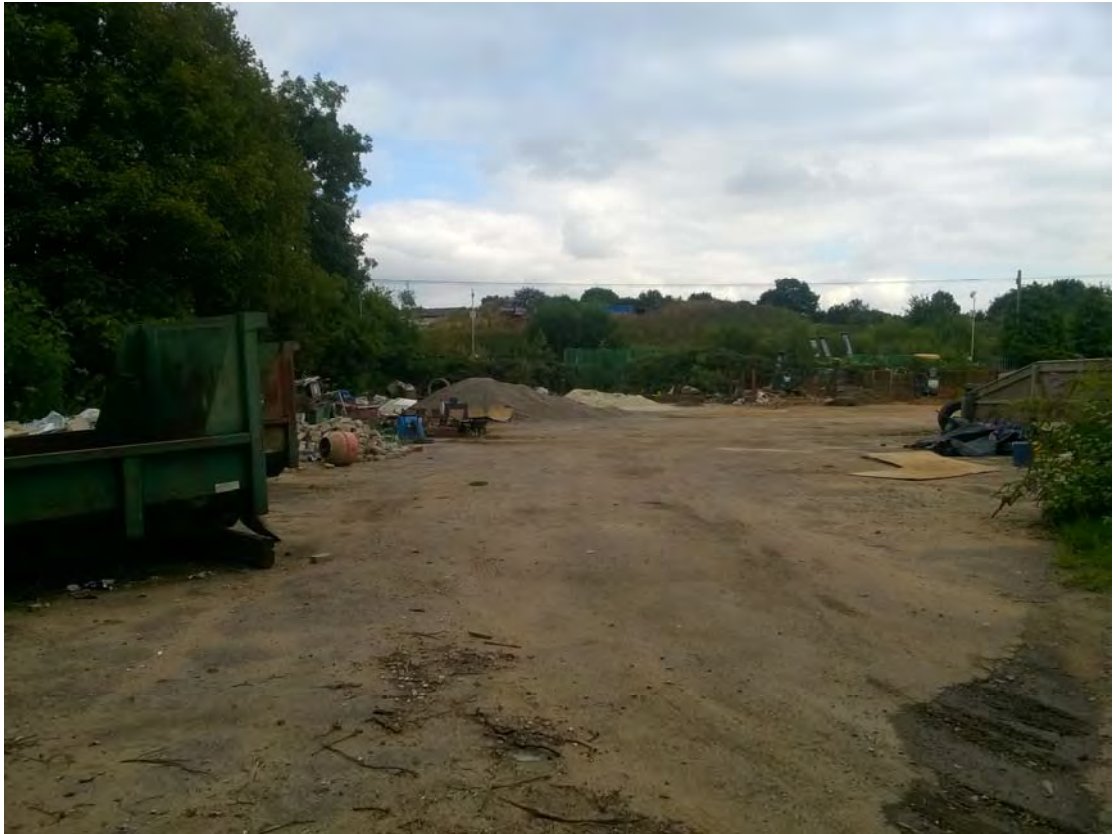
Photograph 6 – Northern boundary looking east.
