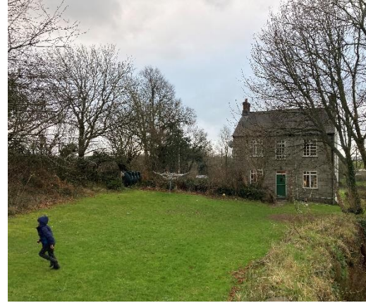
Photo 3: North Elevation of Polwartha Farmhouse showing entrance door (green)
