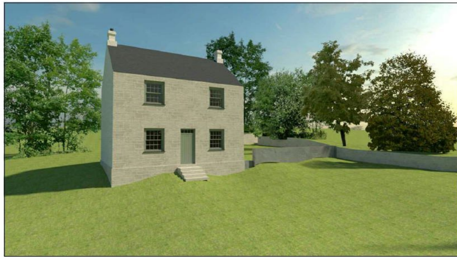
Existing South View
