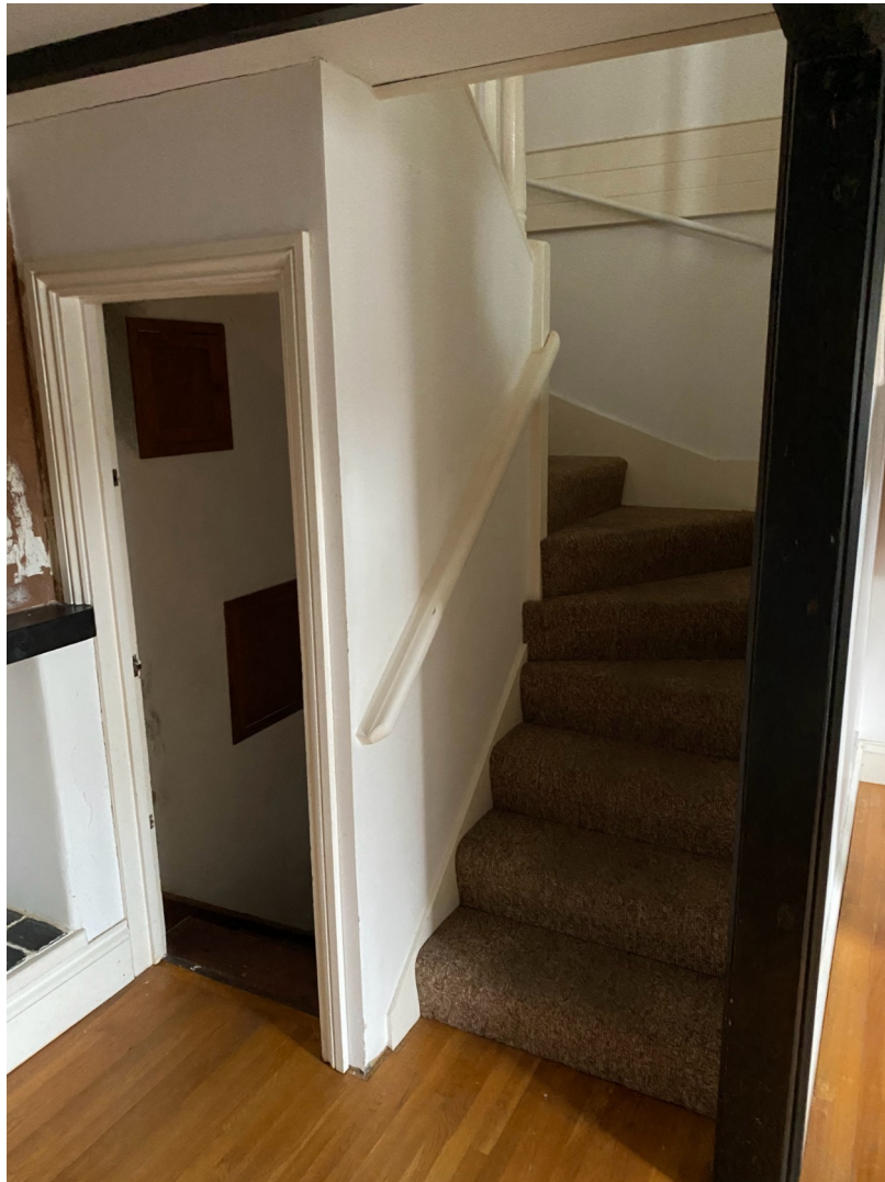
Stairs added in the late 1980s
