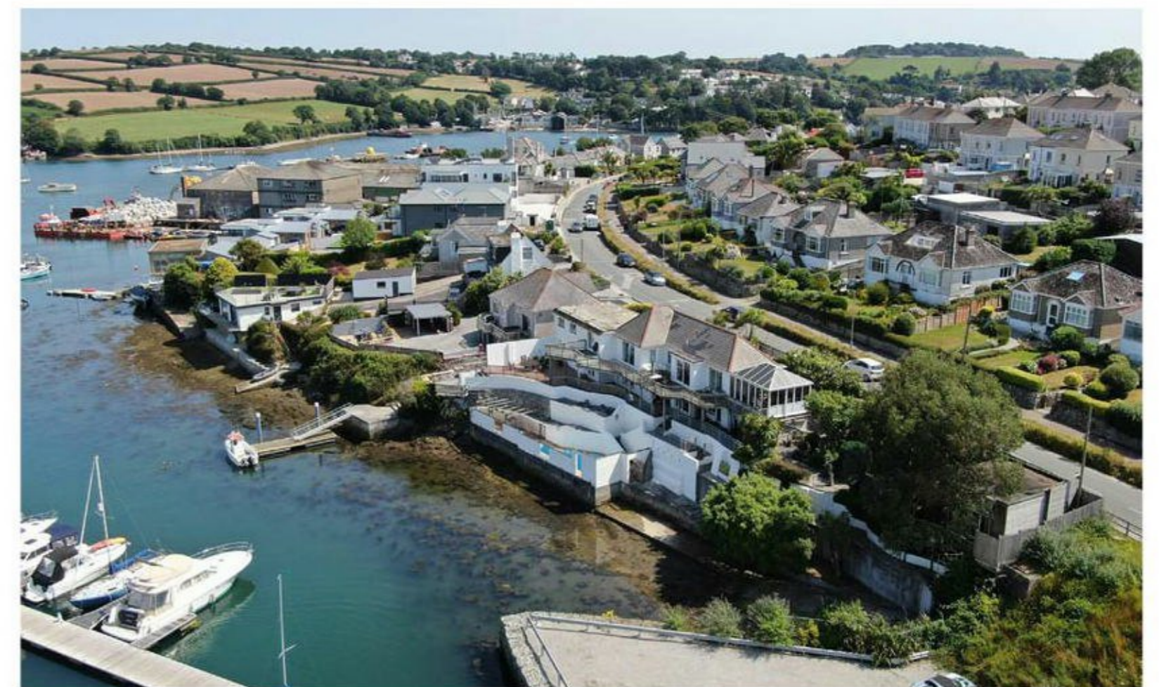
Residential Development at Anchorage 28 North Parade, Falmouth, Cornwall, TR11 2TD
