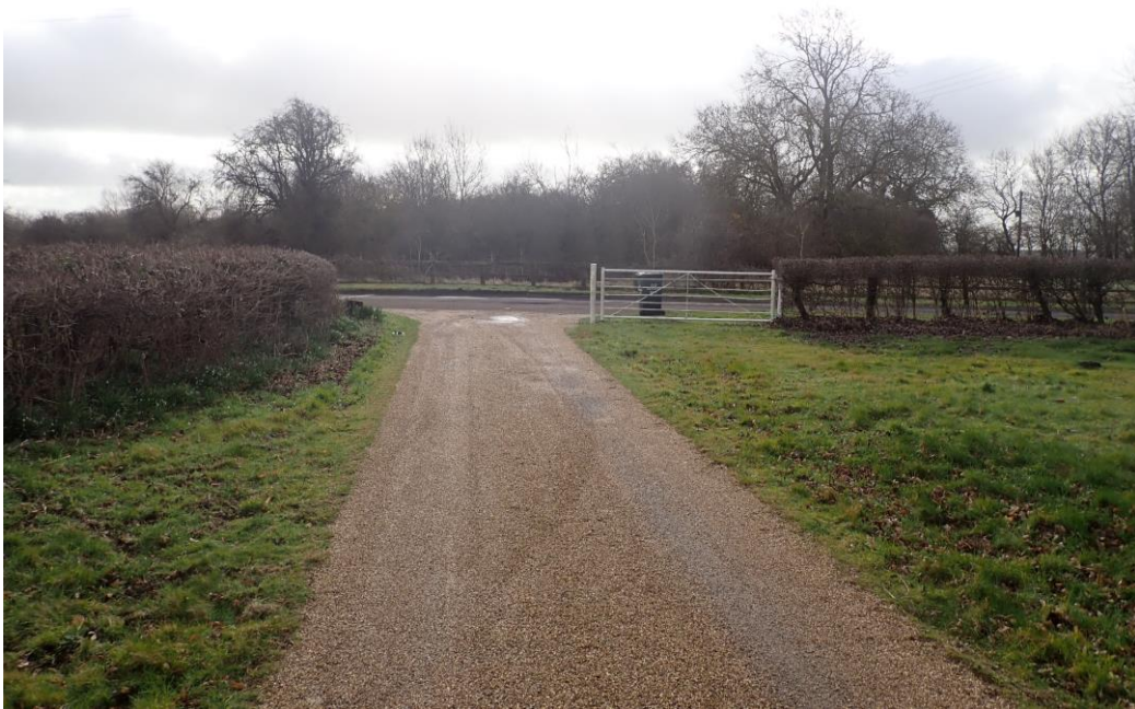
Above: The existing site entrance is open and not secure.
