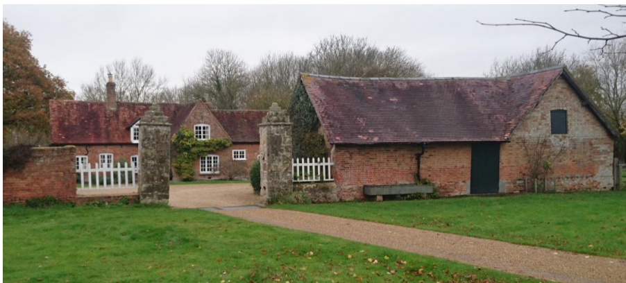
2) The pair of gate piers (List entry Number: 1124285)
