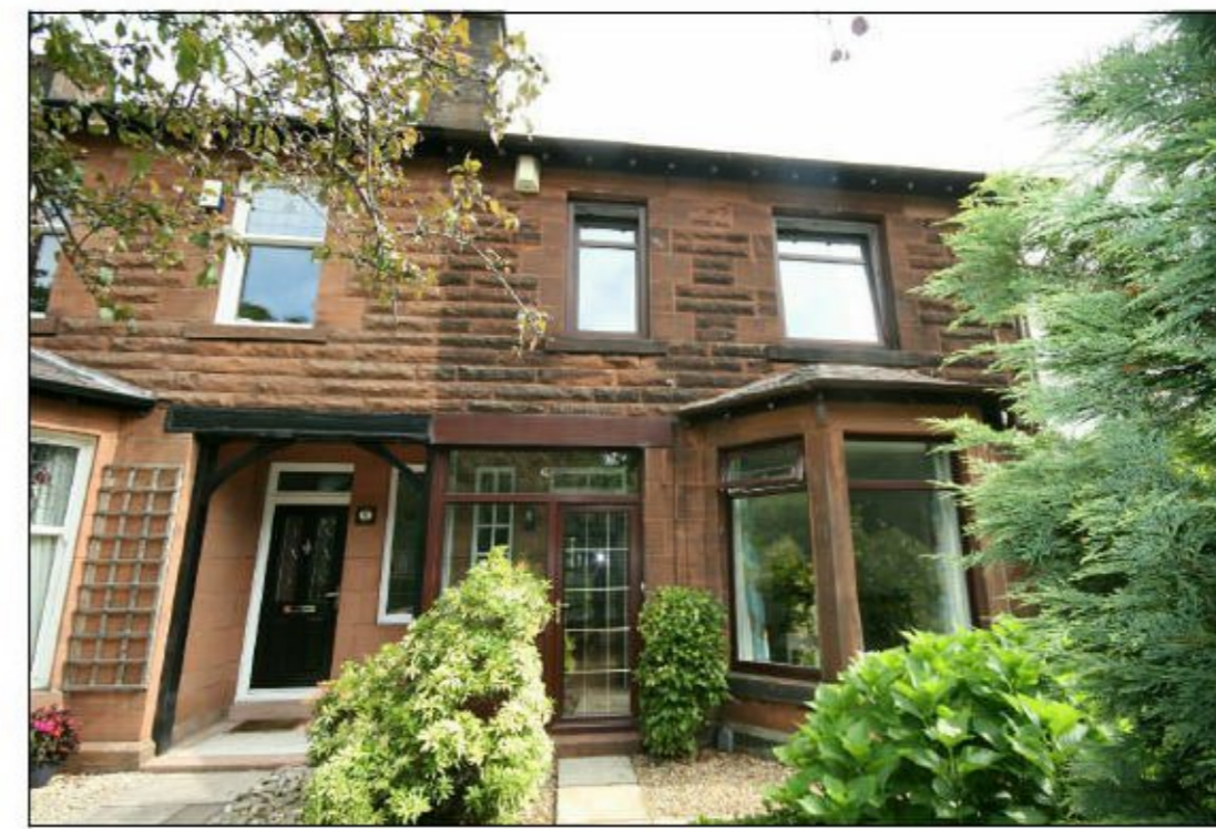
EXISTING PHOTOGRAPH OF FRONT
