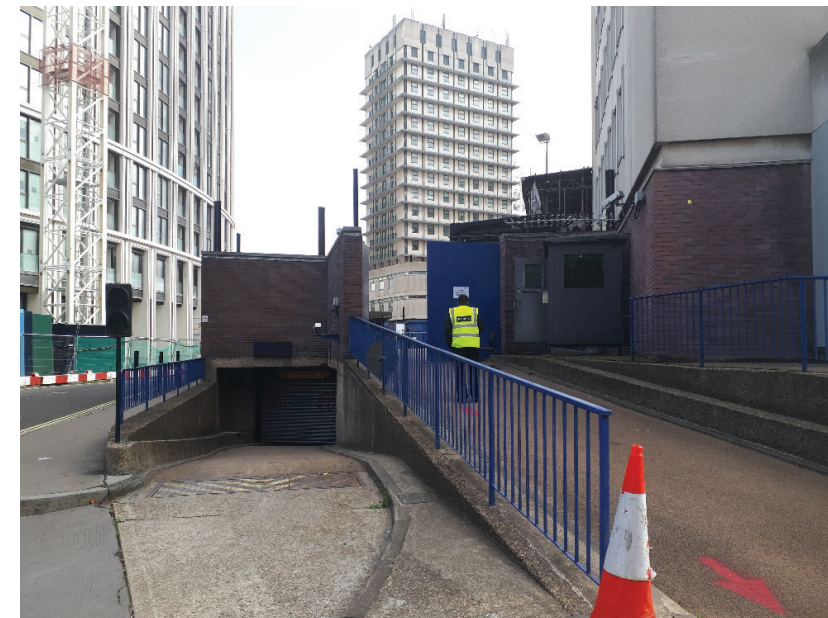
Photo 2. Vehicular site entrance from the west of Newcastle Place.
