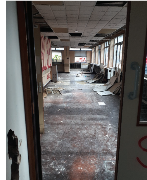
Photo 9. Vacant room located on the first floor of the western tower.
