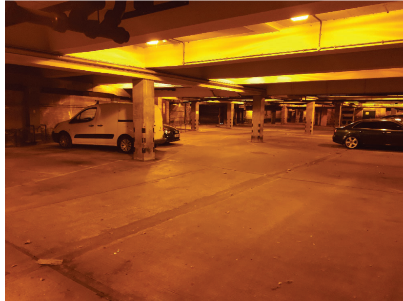
Photo 7. Single storey basement car park, accessed via a ramp located in the east of the site.
