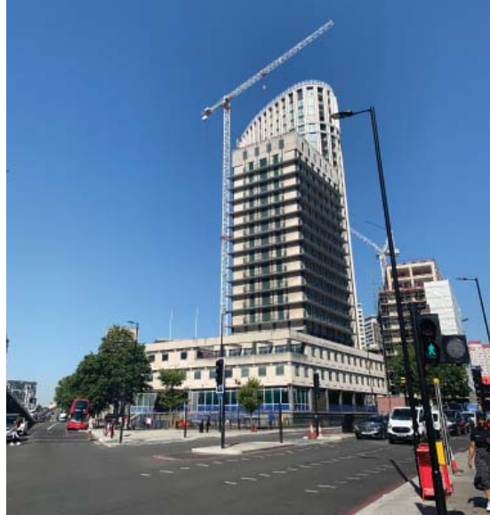
View 1 - Corner of Edgware and Harrow Road
