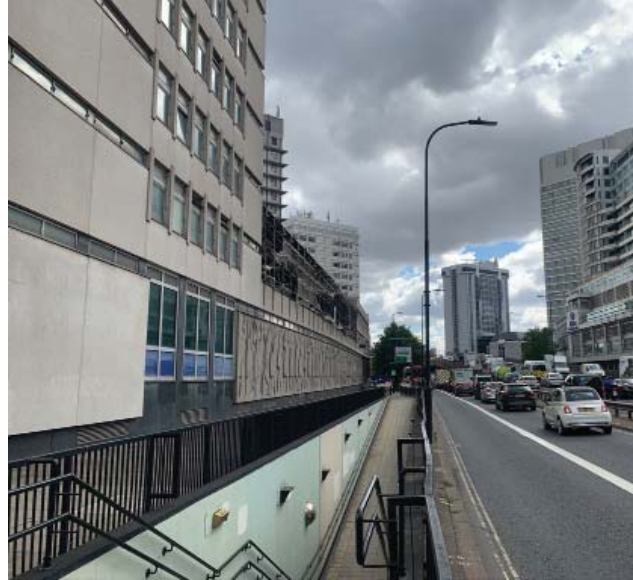
View 2 - View looking east along Harrow Road
