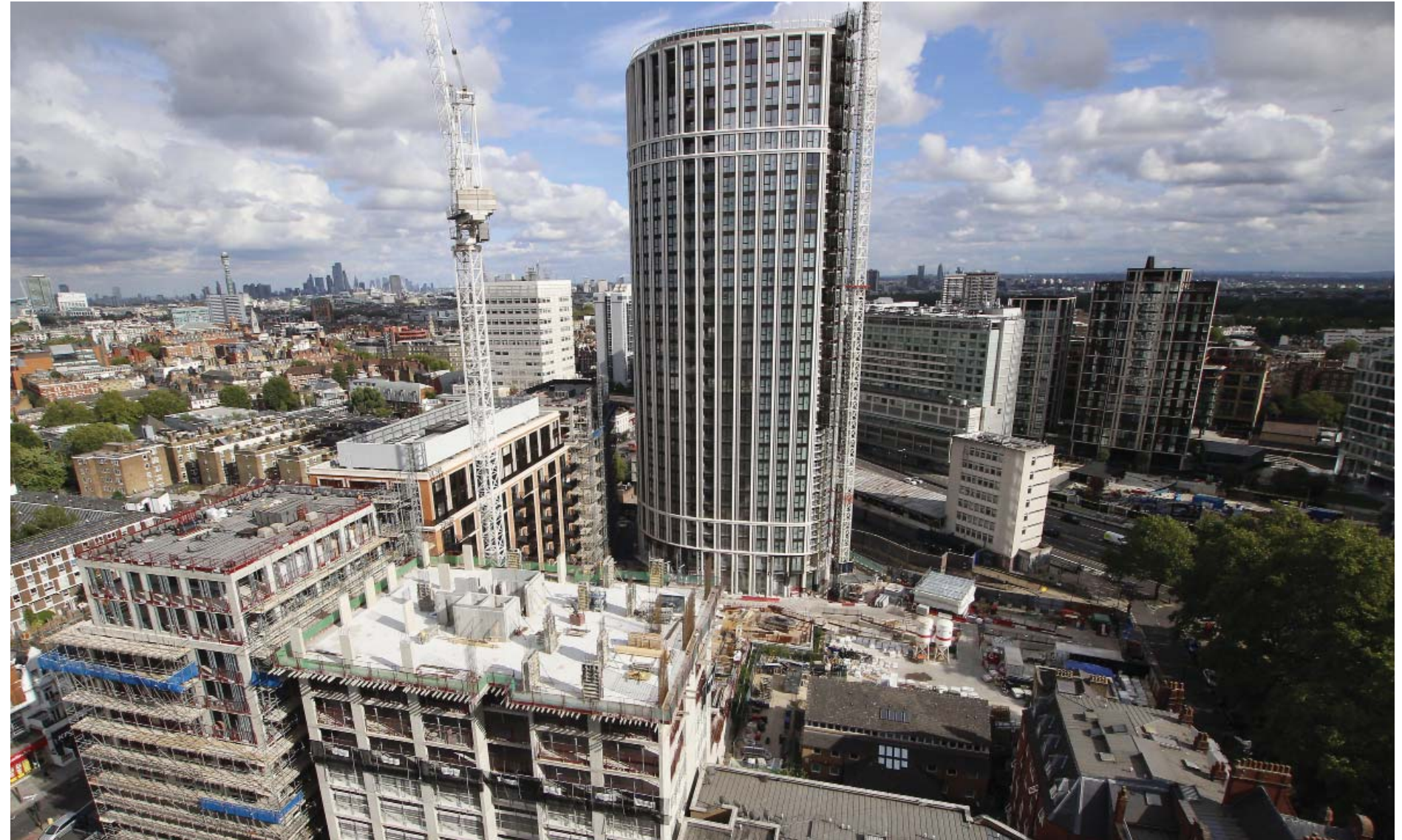
Fig. 2.21 Aerial photograph of site progress on West End Gate site - August 2020
