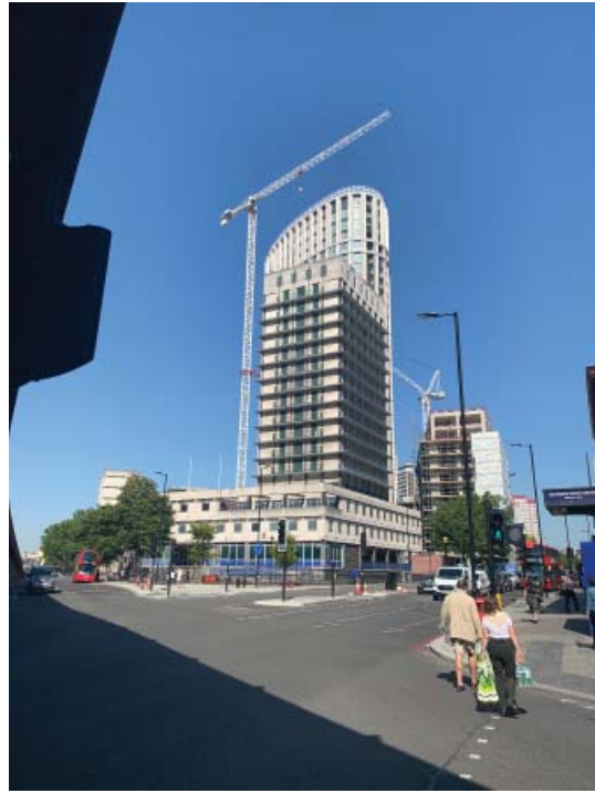
View 4 - View of site from below flyover
