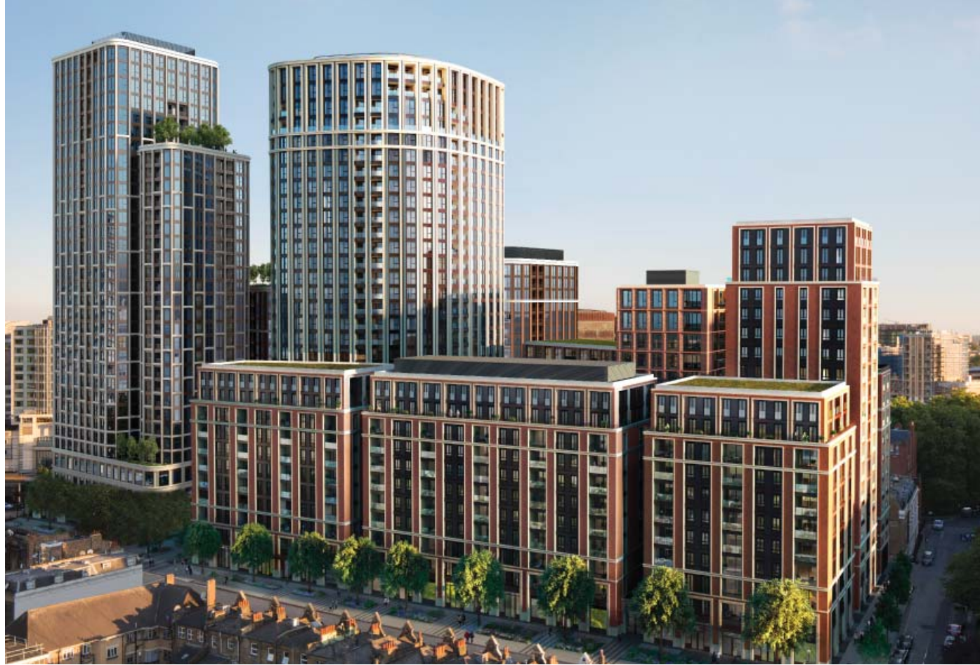
Fig. 7.3 Aerial view looking south-west to completed West End Gate Masterplan
