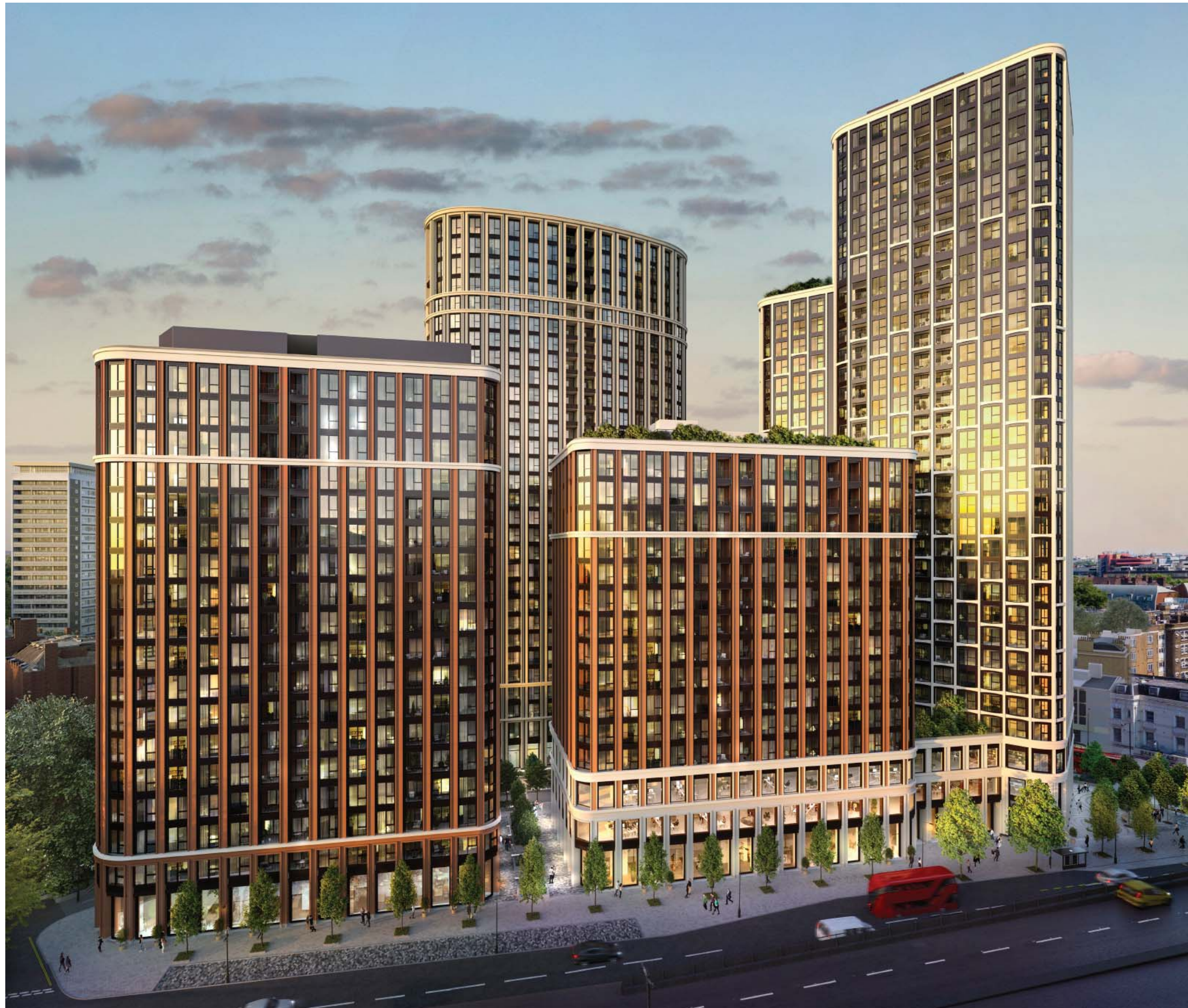
Fig. 7.6 Aerial view from Harrow Road looking north
