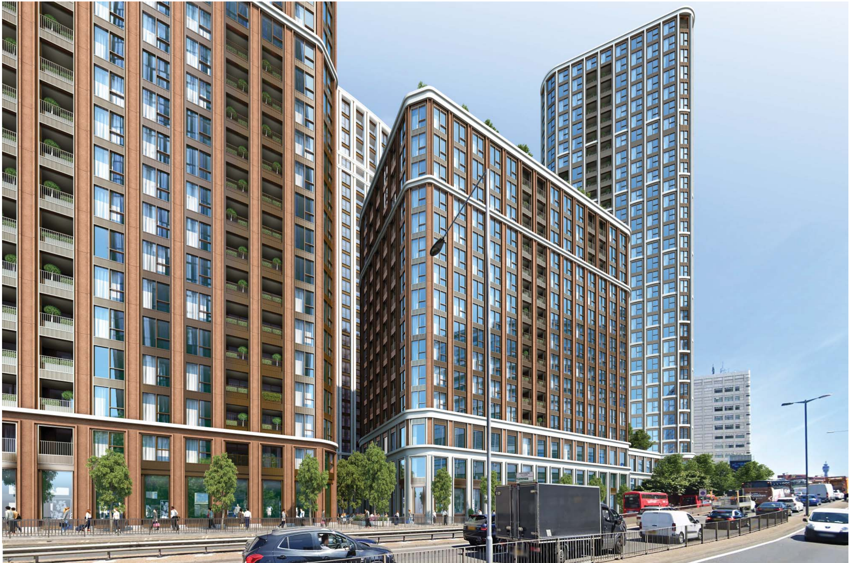
Fig. 72 View from Westway looking north at central mansion block (Block J)
