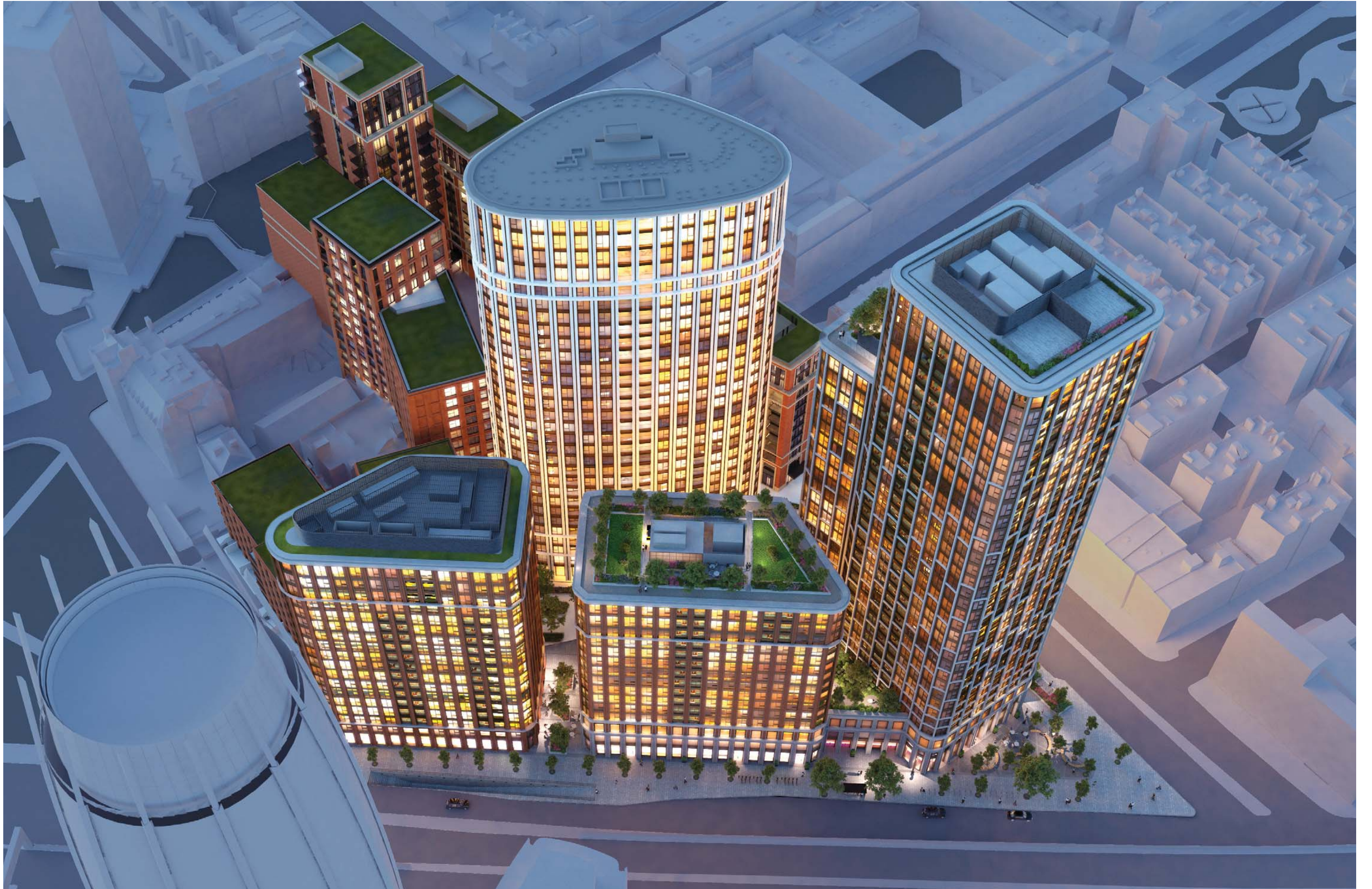
Fig. 79 Aerial view looking north to completed West End Gate Masterplan
