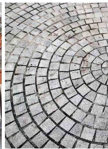
Feature granite paving
