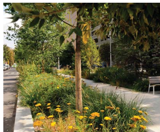
Streetscape improvements (incorporating TFL rain gardens)
