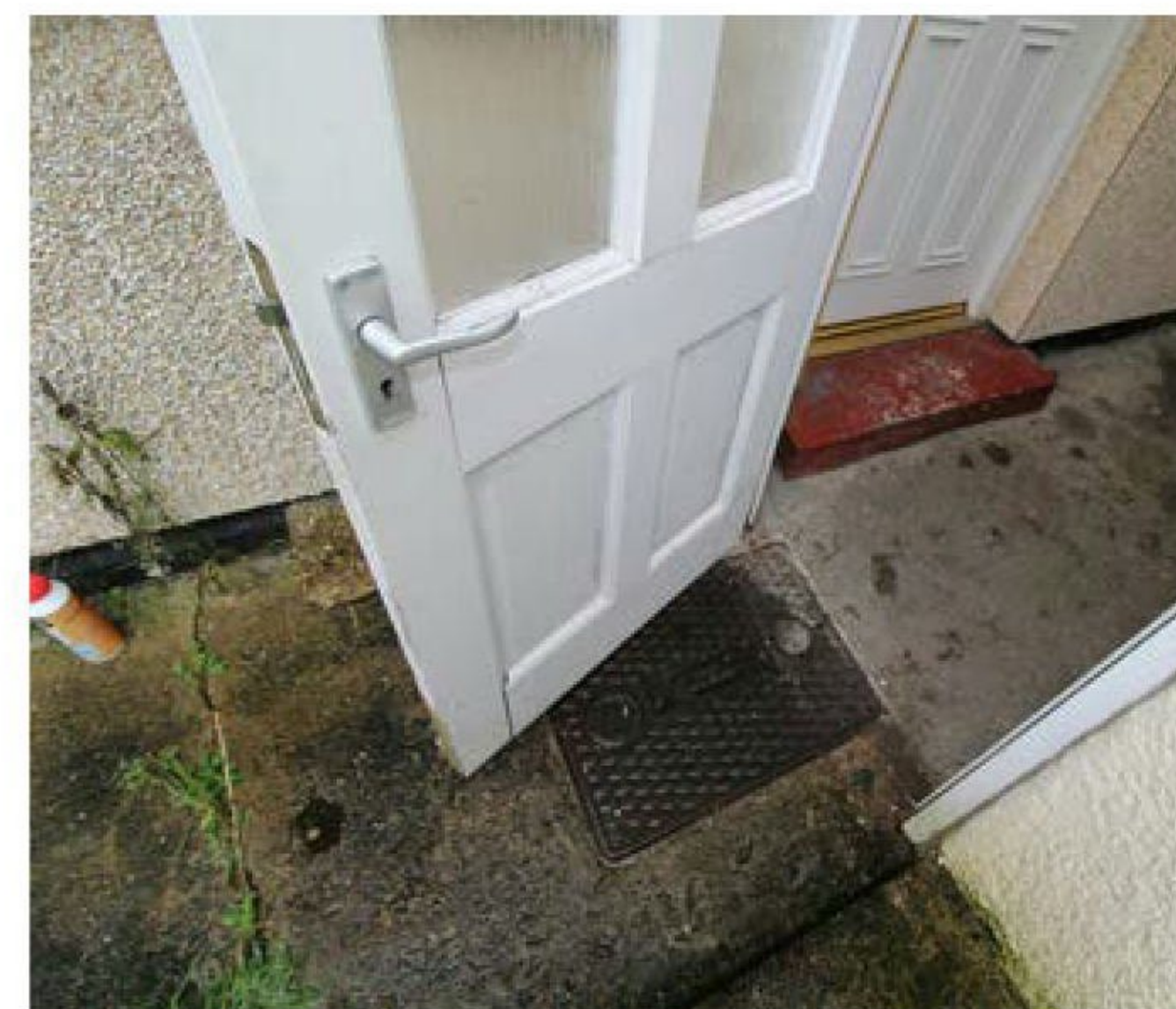
[Figure 41] Foul water cover to rear
