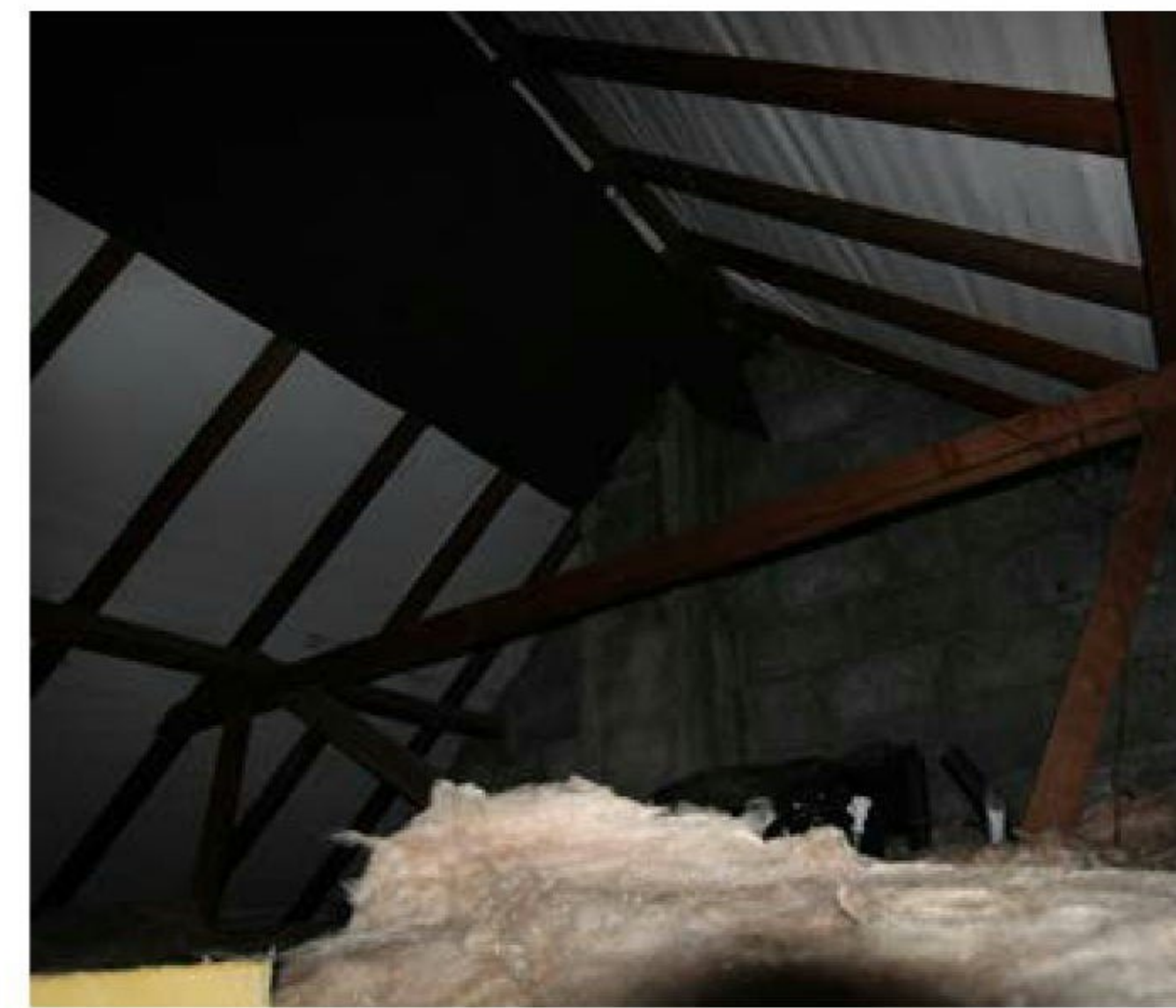
[Figure 38] Timber roof trusses
