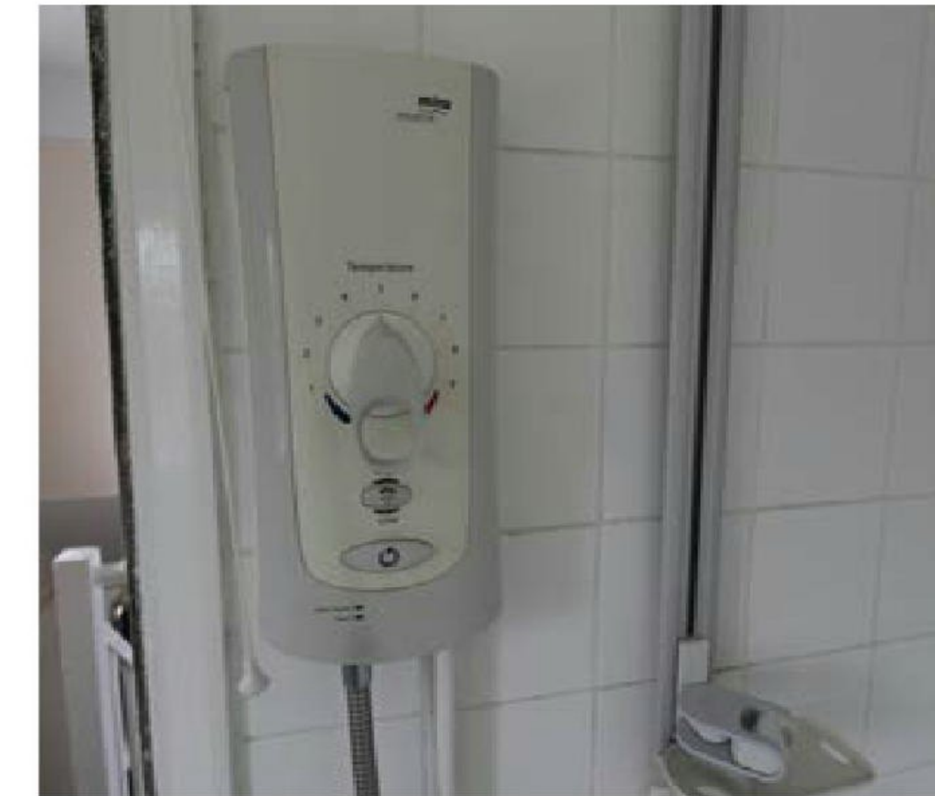
[Figure 29] First floor Bathroom
