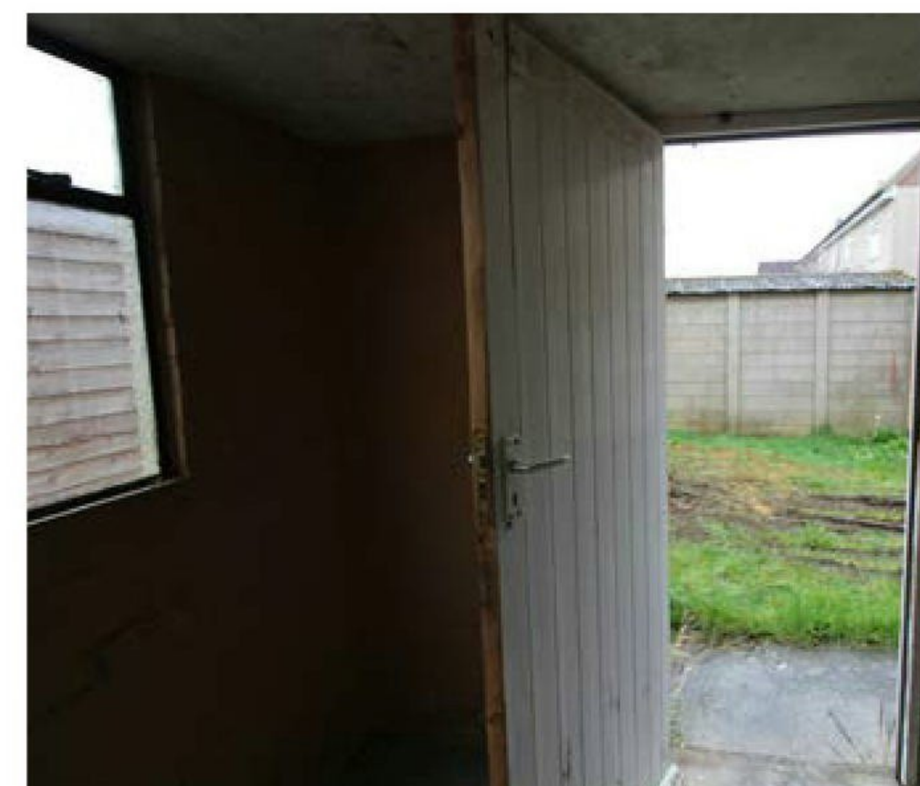
[Figure 24] Outbuilding room 3
