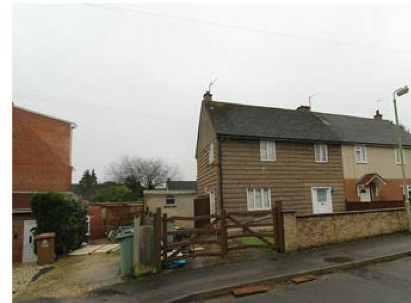
[Figure 39] Original cladding at No.22
