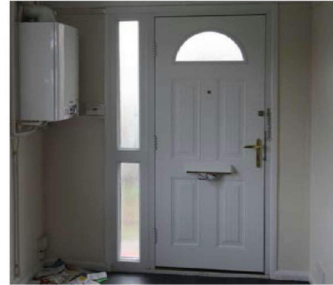
[Figure 15] Entrance hall and stairs
