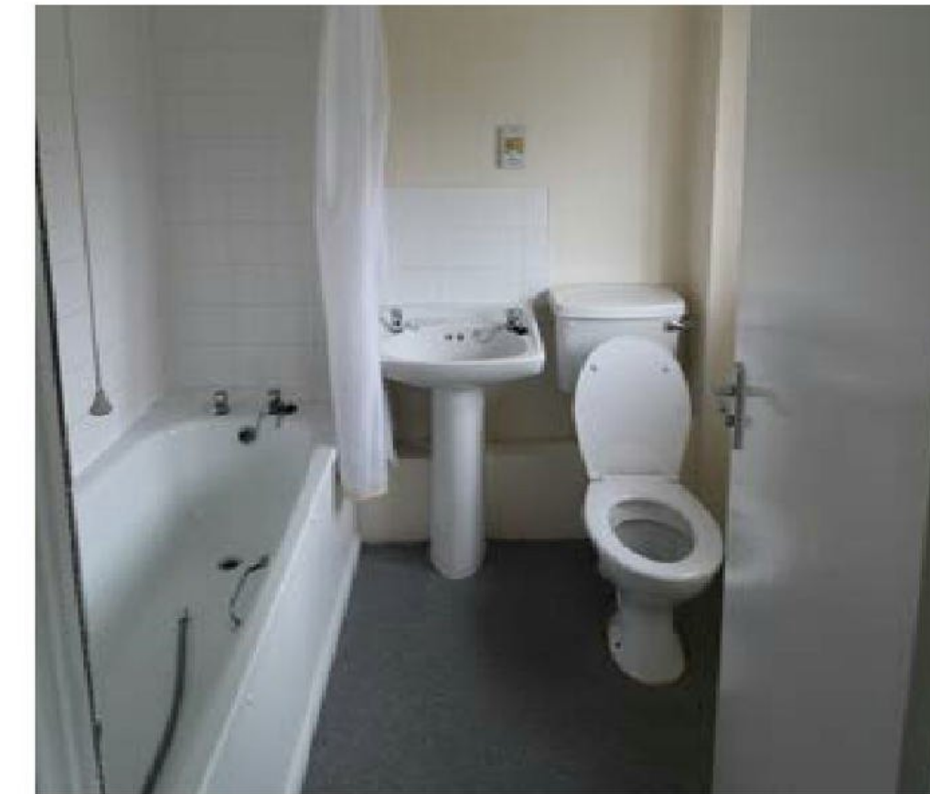
[Figure 28] First floor Bathroom
