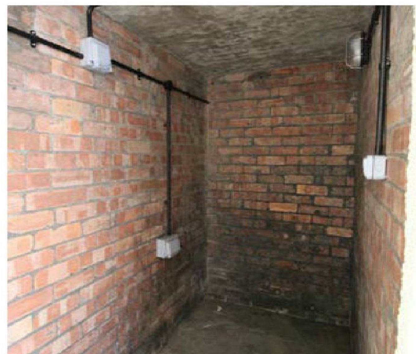
[Figure 22] Outbuilding room 1
