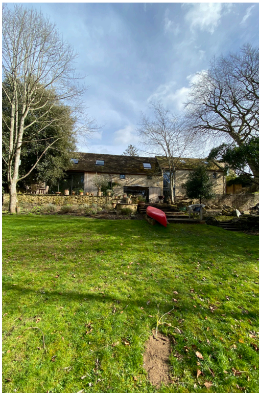
Rear elevation of the Malt Barn
