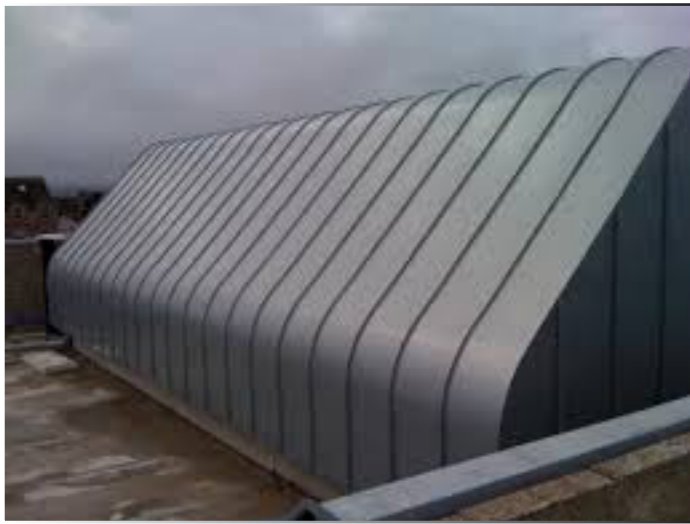
Standing seam copper roofing
