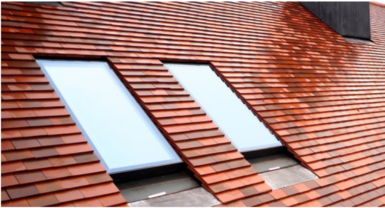
'Neo' flush roof glazing set into plain tile roof
