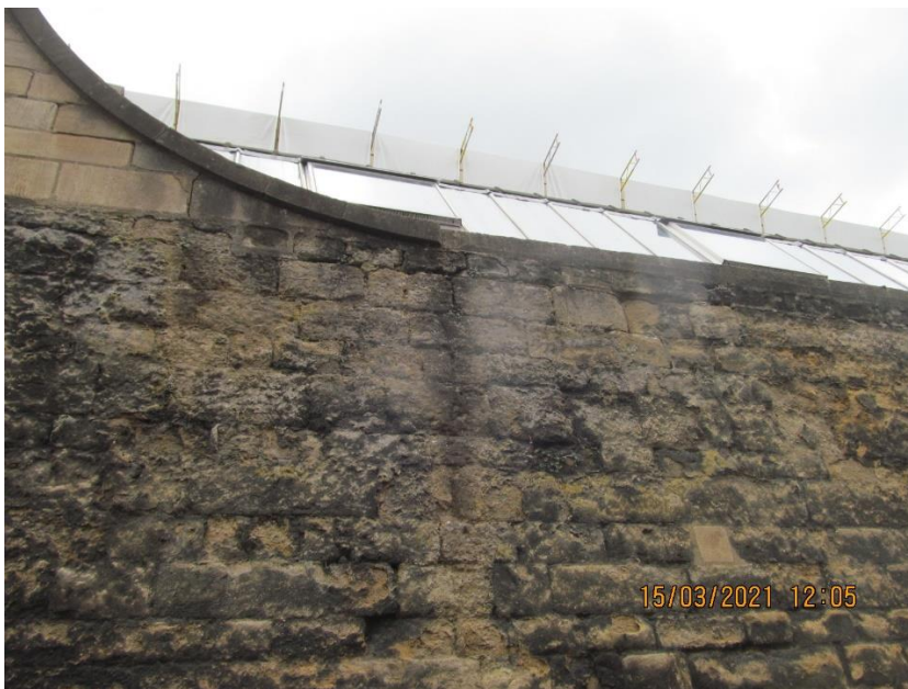
Transition original stone coping to central wall cast concrete
