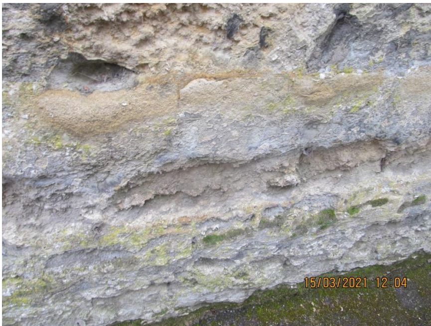
Friable surfaces/unsuitable patch repair and pointing materials
