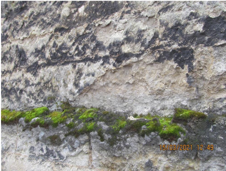
Friable surfaces/unsuitable patch repair and pointing materials
