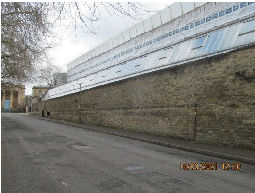
Transition original stone coping to central wall cast concrete
