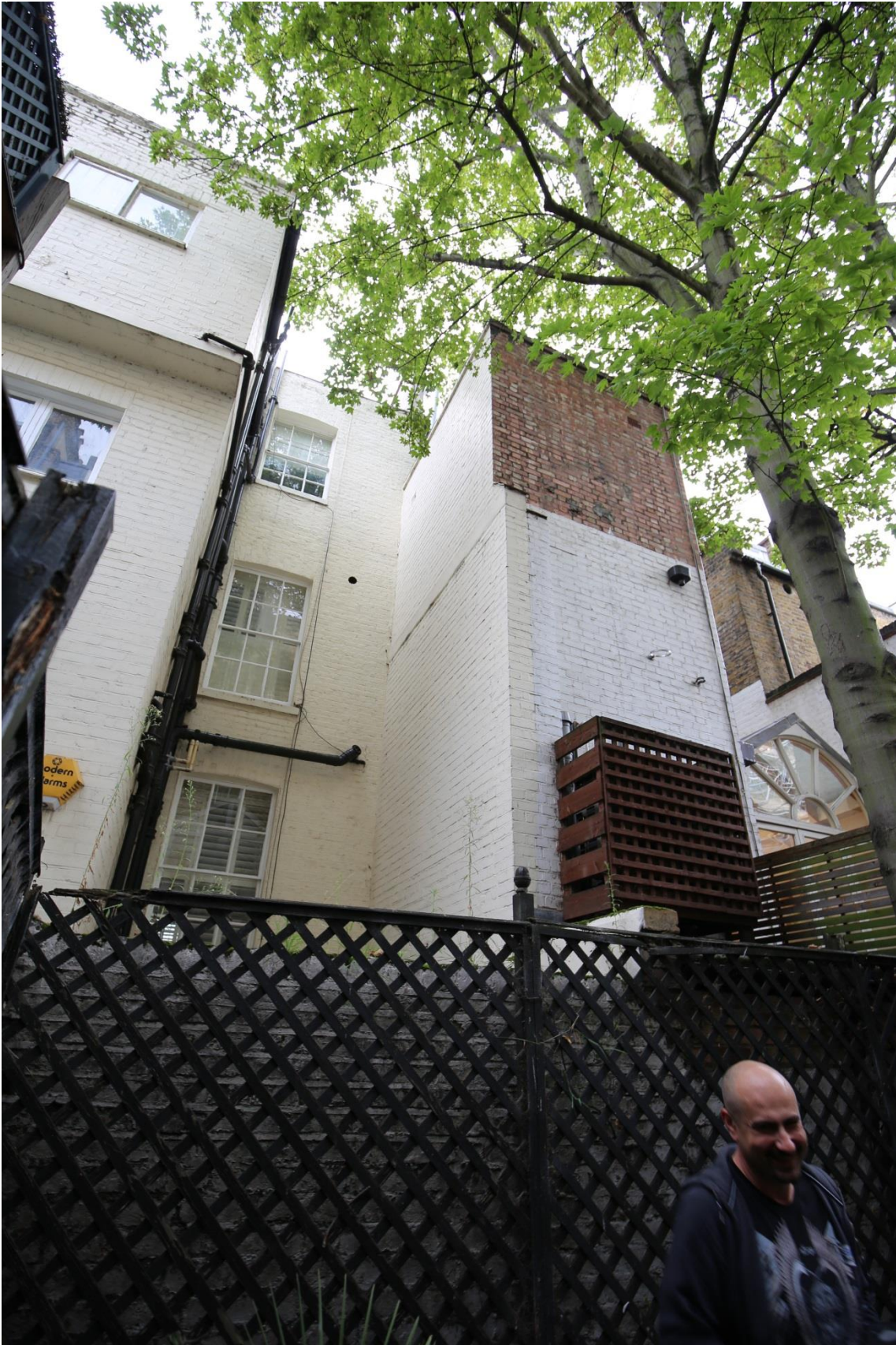
View of the elevations facing the rear garden
