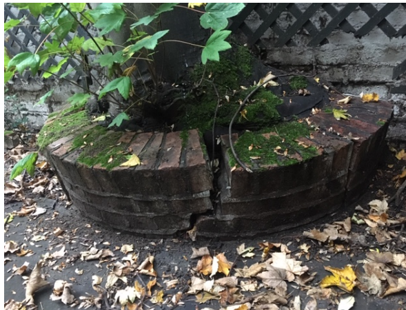
Base of tree T1 as viewed in an easterly direction showing constrained raised planter and root girdling
