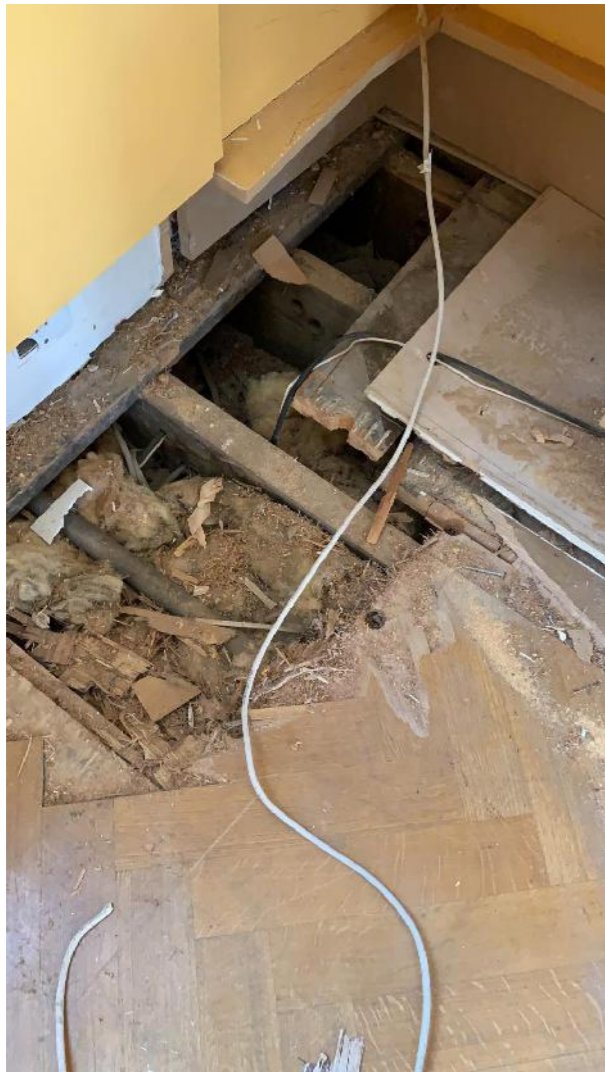
1 layer of Timber harring bone 1 layer of ply mixed with pine planks Joists 220X50
