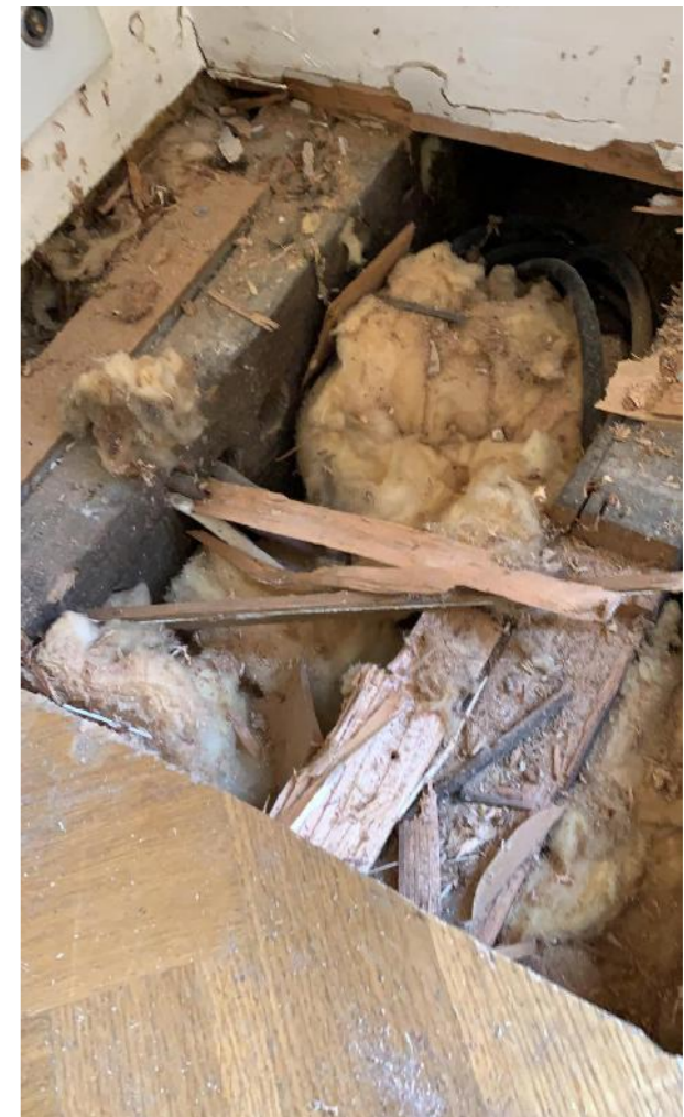
1 layer of Timber harring bone 1 layer of ply + firrings to level the floor Joists 220X50
