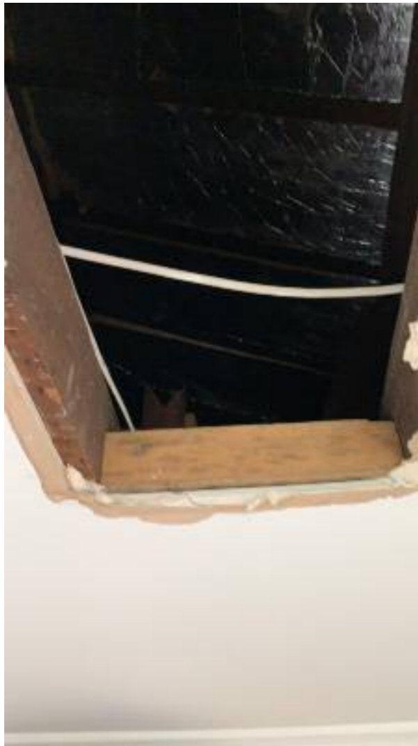
New roof structure visible New insulation Small fargments of the orginal roof structure , heavily altered
