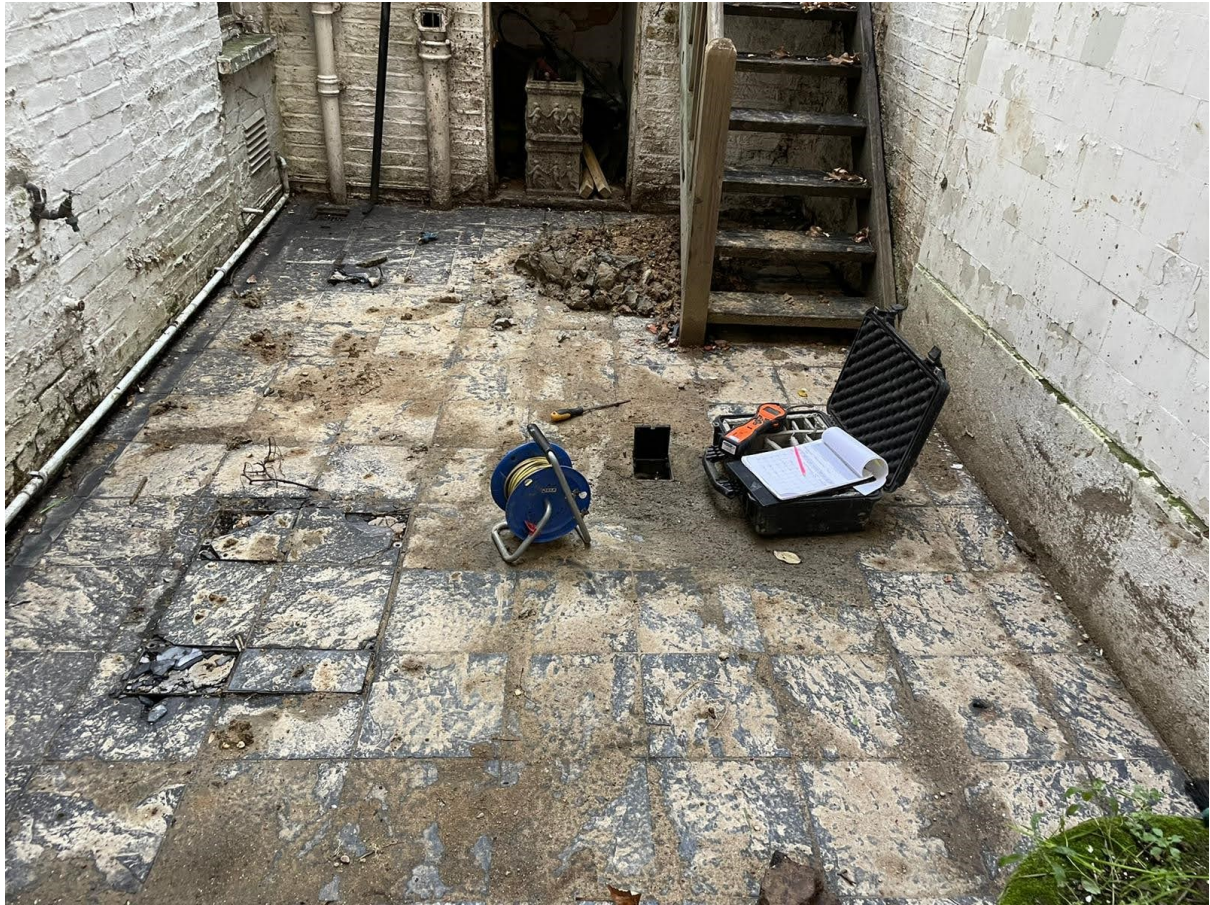
Photograph 6: Exploratory hole dug on the basement level terrace area.
