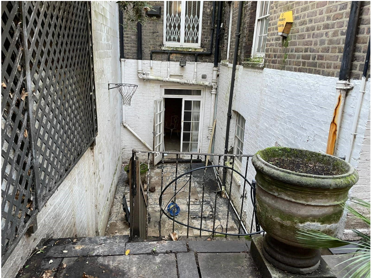
Photograph 10: View overlooking the basement level at the rear of the building.
