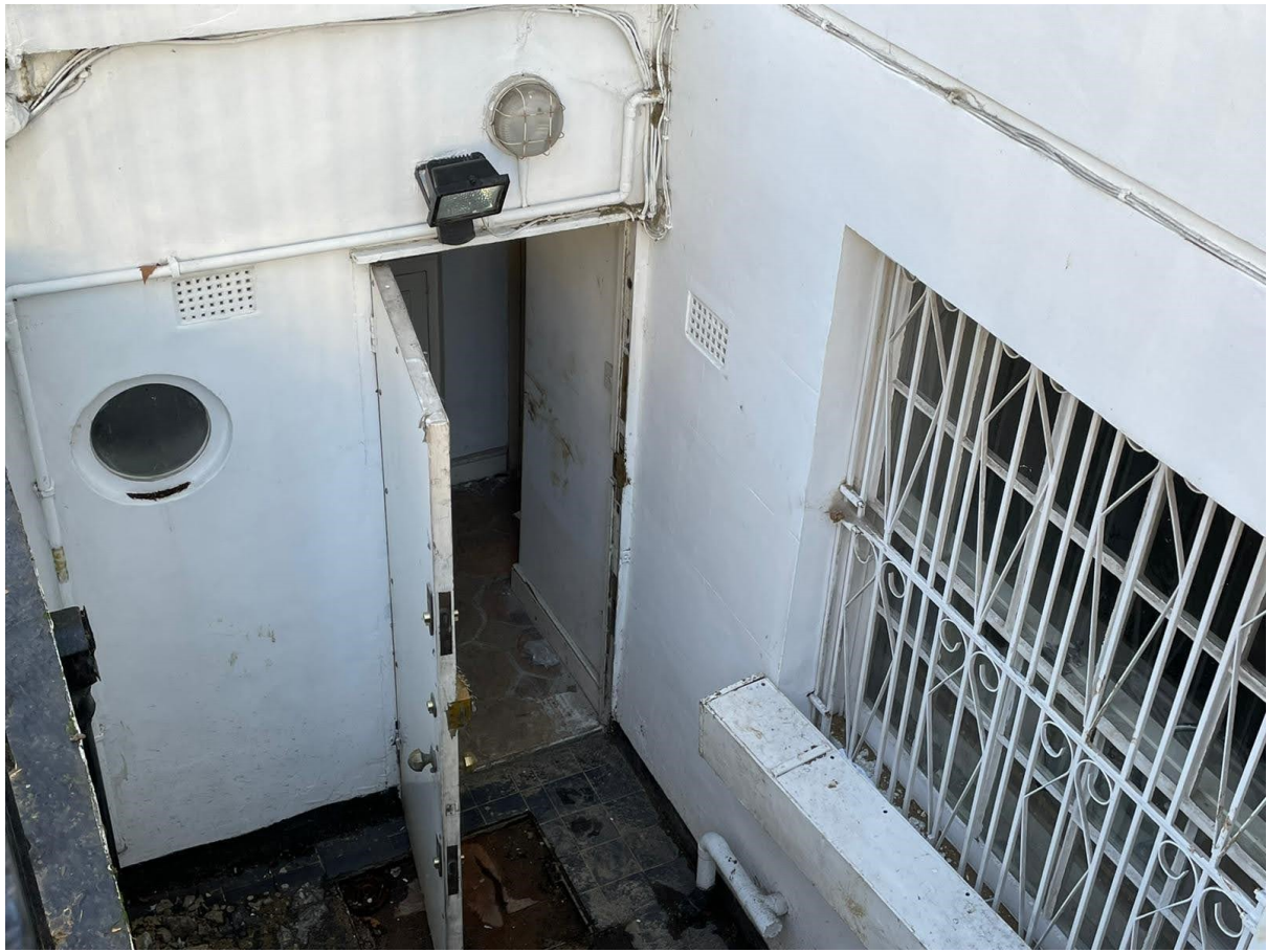
Photograph 5: Ground Floor (rear) of the building.
