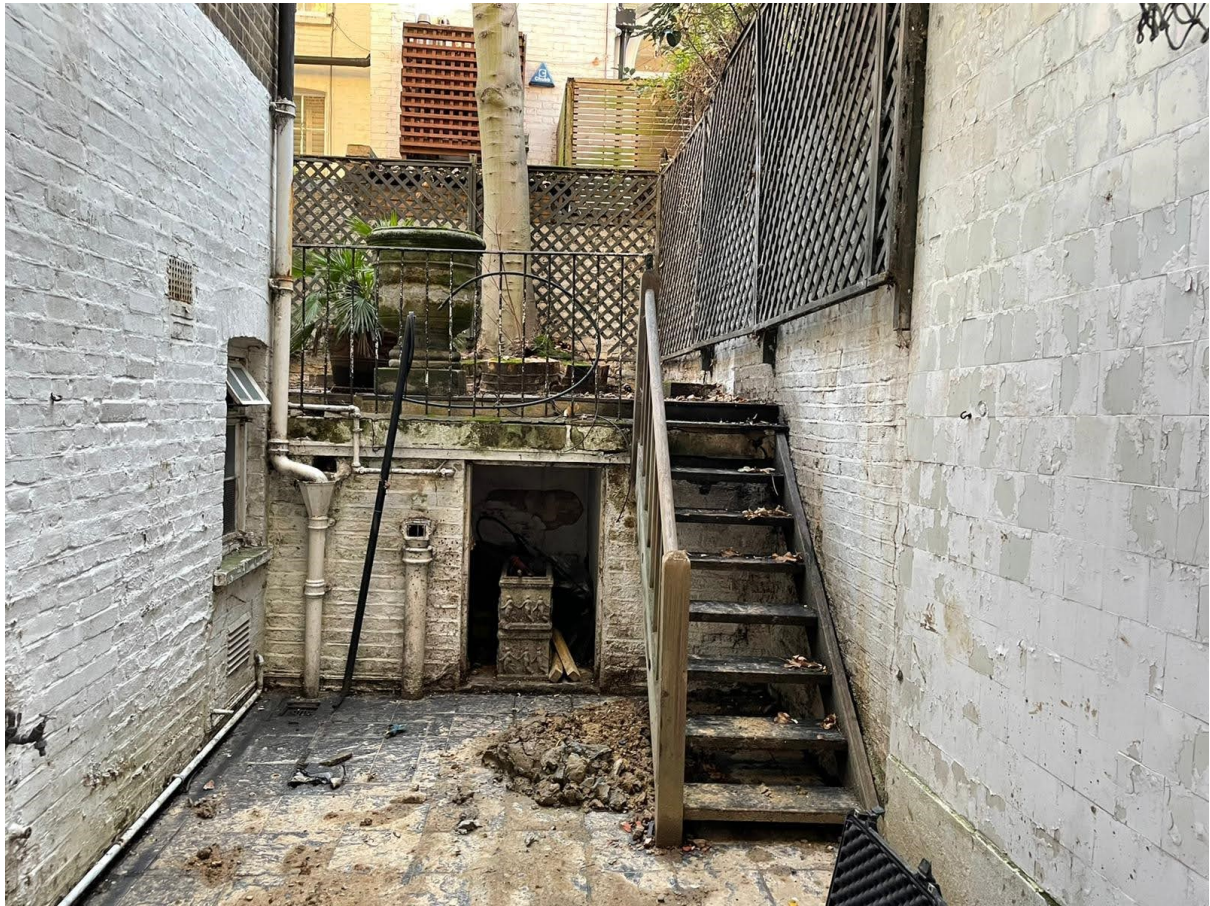
Photograph 8: Basement level at the rear of the building.
