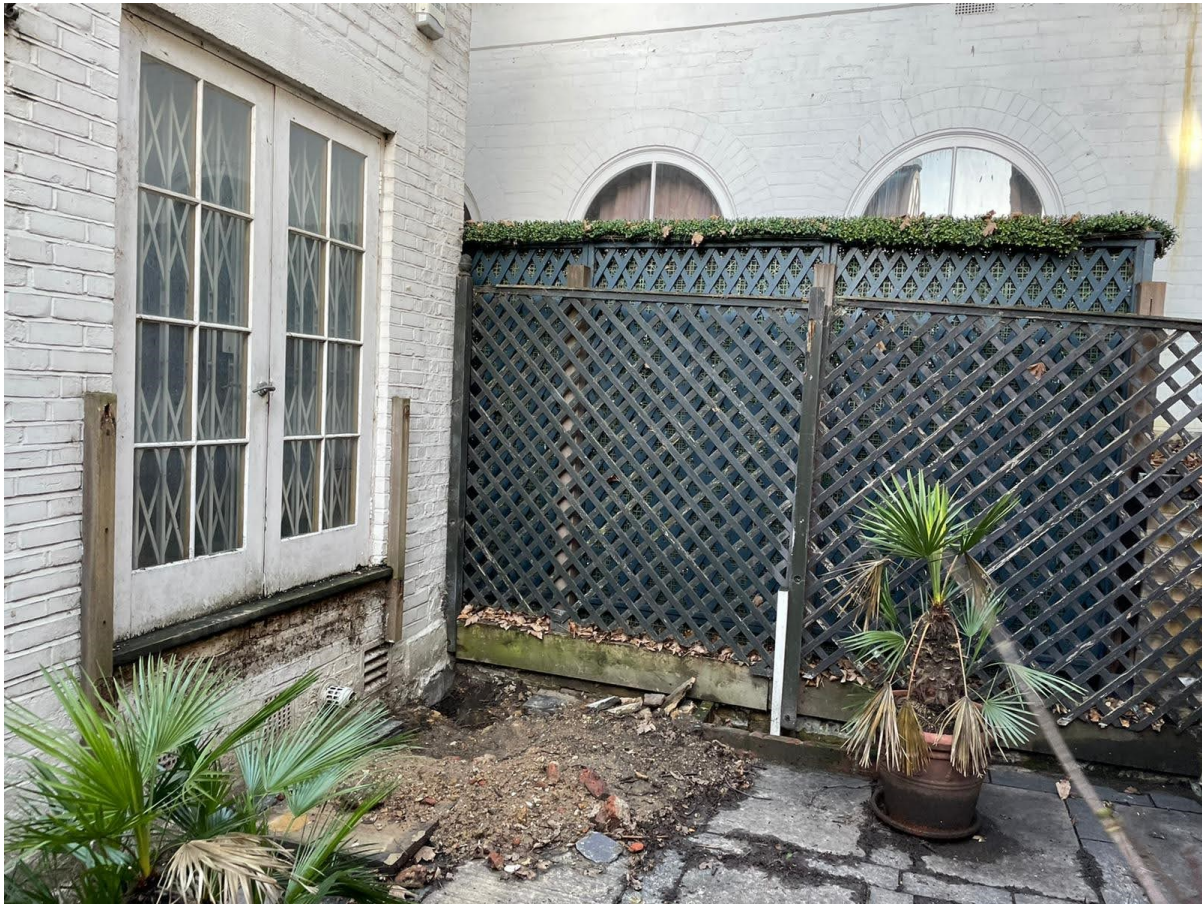
Photograph 12: Ground floor garden area, viewing towards the north.
