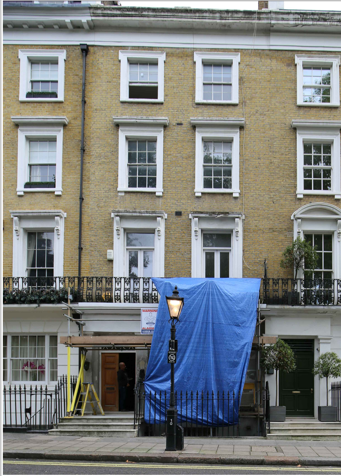
PHOTO OF EXISTING - FRONT ELEVATION
