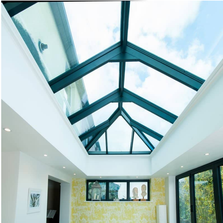
Roof lantern internal view
